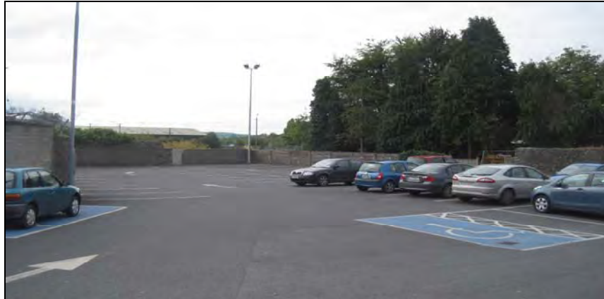
Figure 6.1 Council owned car park to the south of Main street which is not widely used
