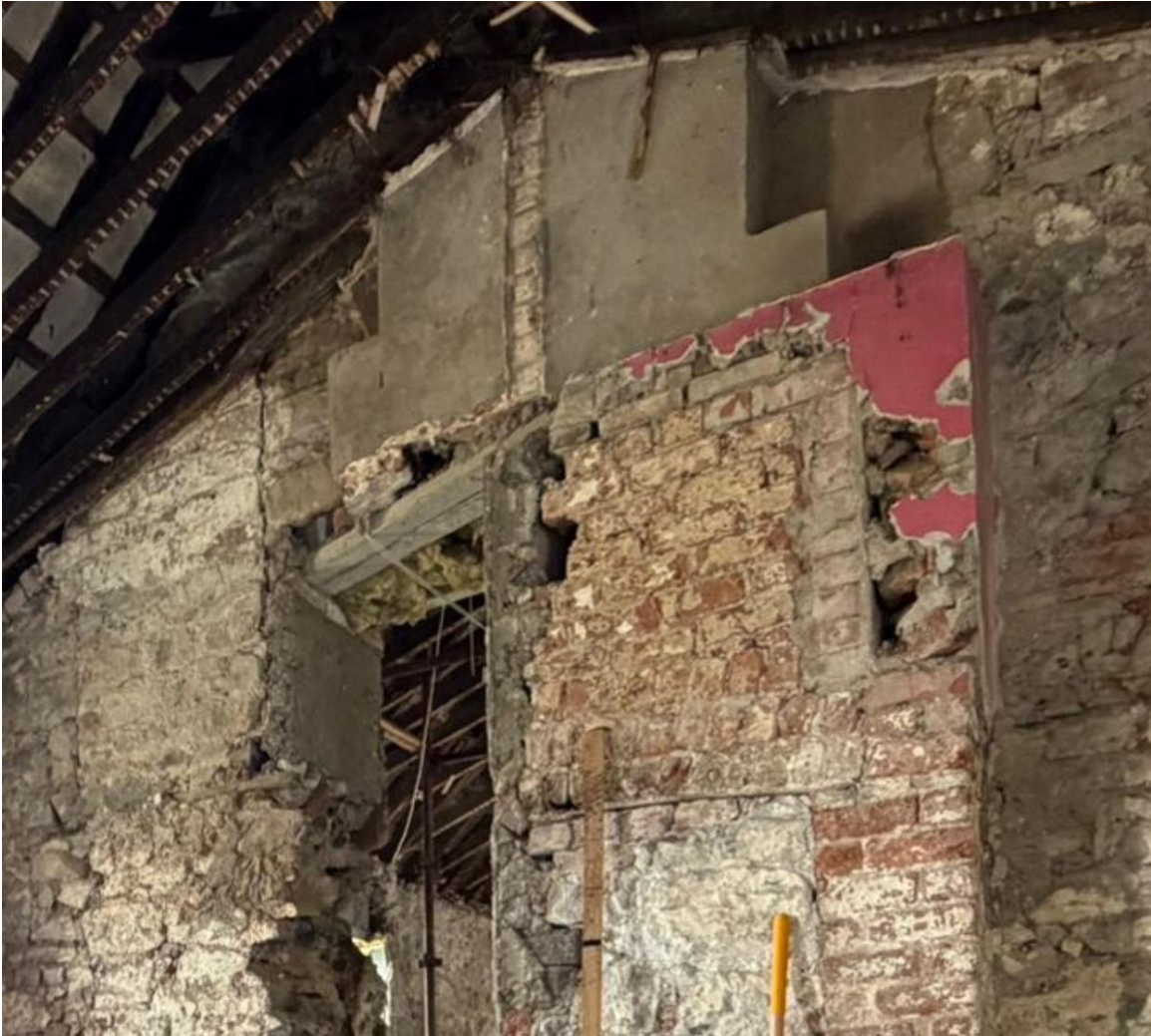
Existing Chimney requiring demolition / Stabilisation works
