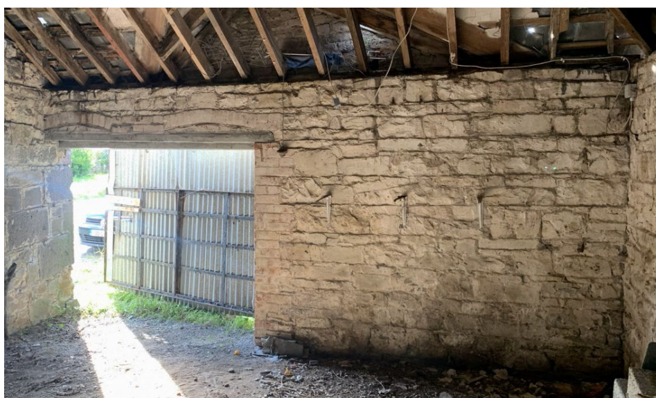
Figure 2-3: Building 2 Solid Walls
