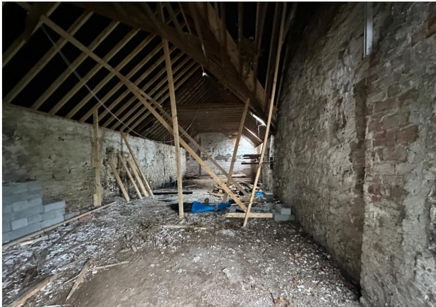
Existing roof requiring propping
