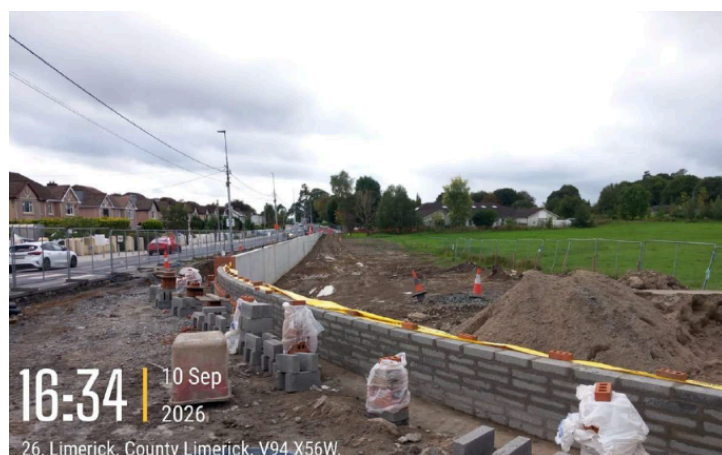
Blockwork for the new radius wall at the entrance to St Munchin's.
