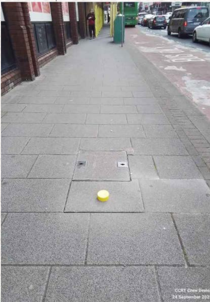
Footpath repairs City Centre
