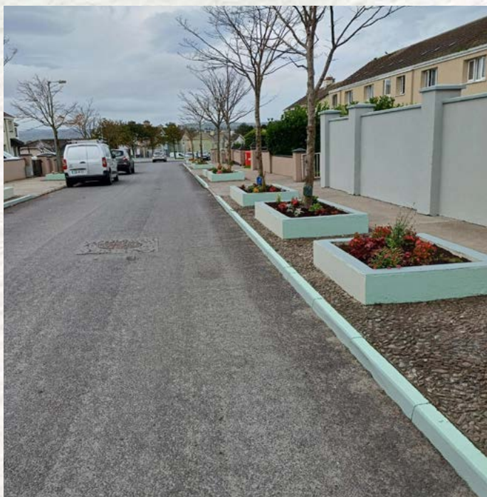
Hillview Drive Estate Enhancement Project
