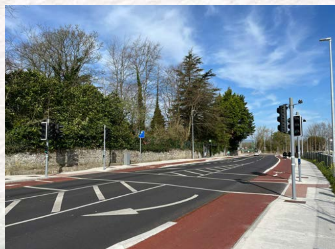
Plassey Park Road Improvement Scheme
