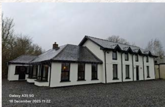
Derelict Property AFTER
