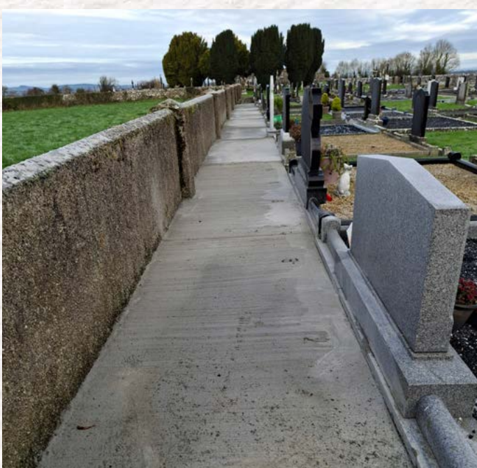
Effin Graveyard, Footpath Replacement Works
