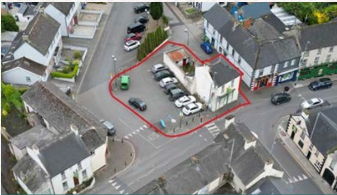
Croom Square Project Site
