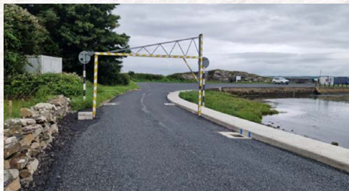
Surface Dressing Works Kiltewy Pier
