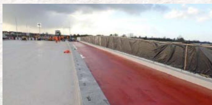
The Bridge Deck waterproofing of Ballygrennan Bridge has been completed with the remainder of Bridge works due for completion in Quarter 1 2026
