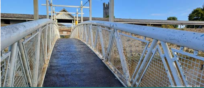
Footpath repairs City Centre
