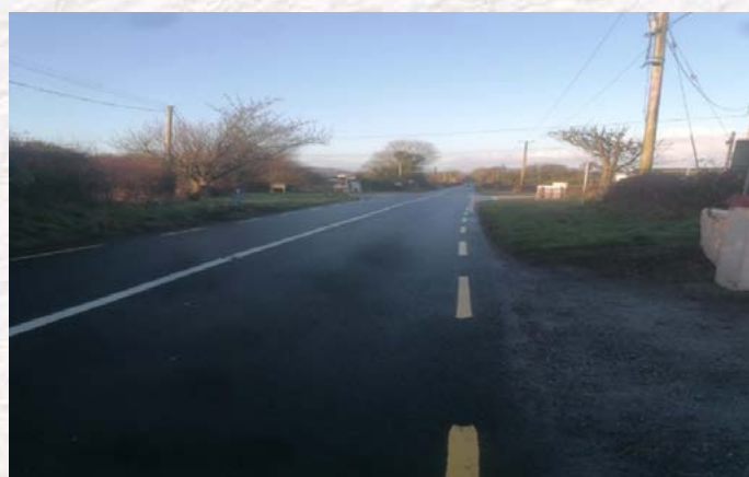
R516 Crean Cross Resurfacing
