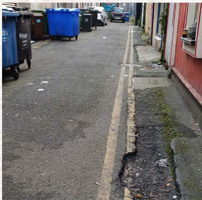
Limerick Lane before works
