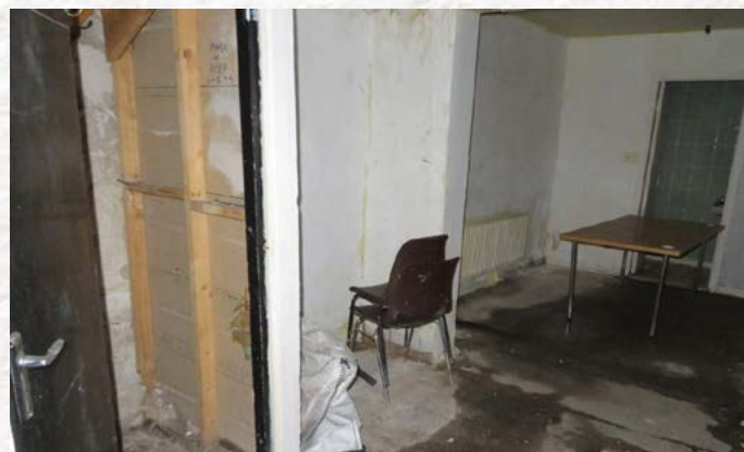
Refurbishment Greenhills Limerick – Before
