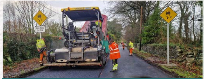
Road Overlay on the R512 between Ballyneety and Grange
