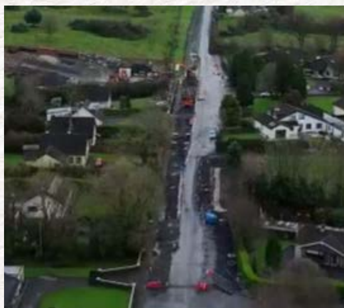
Works has commenced on the installation of the foul and storm sewer on the Cratloe Road
