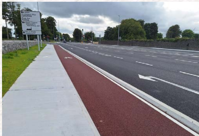
View West on R445 (Dublin Rd.)
