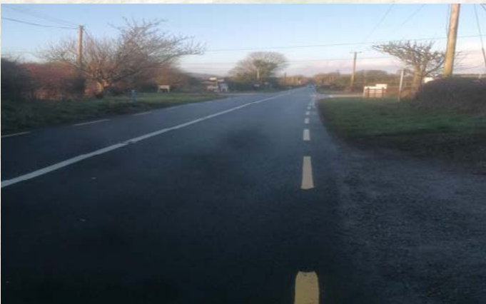
Road Reconstruction Works R516 Crean Cross
