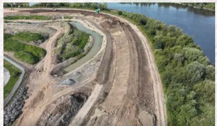
Embankment St. Marys Park
