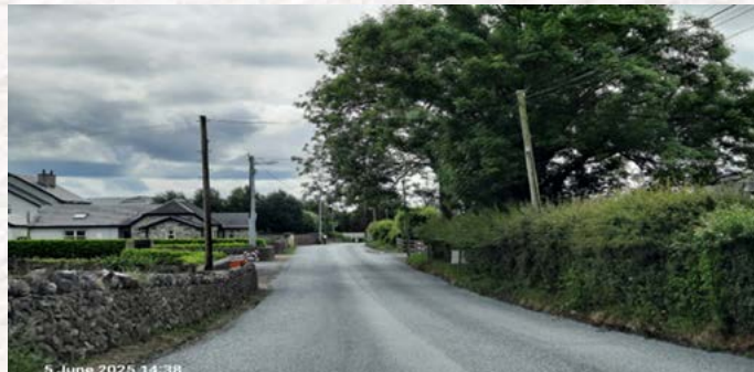
Surface Dressing Works Clonnanna
