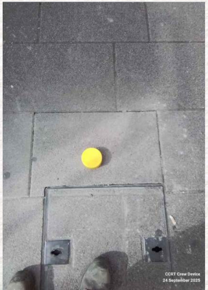
Footpath repairs City Centre
