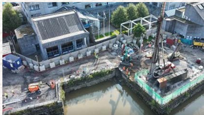
Piling at Civic offices
