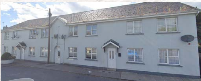
The Forge Apartments, Hospital
