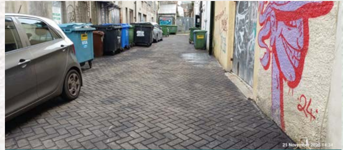
Limerick Lane after works
