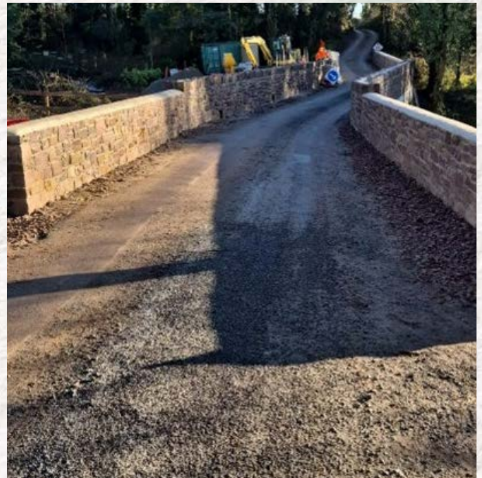
Structure A - L80001 Coolattin Bridge
