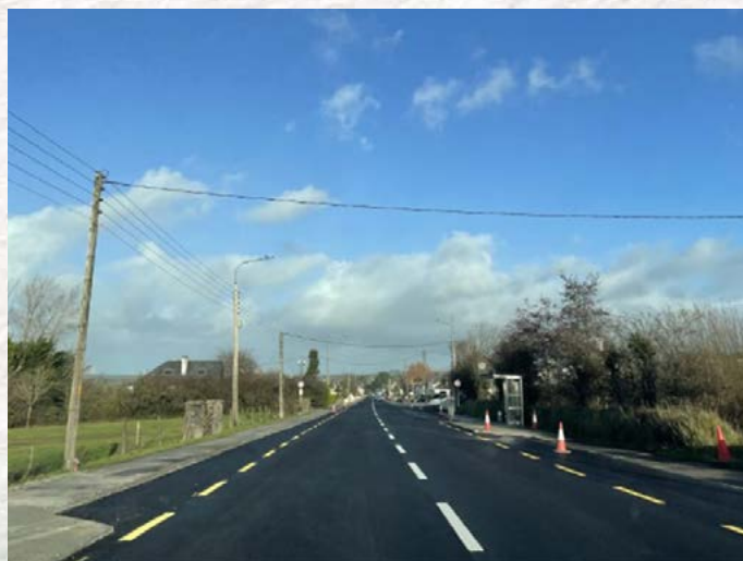
Abbeyfeale Western Approach Resurfacing
