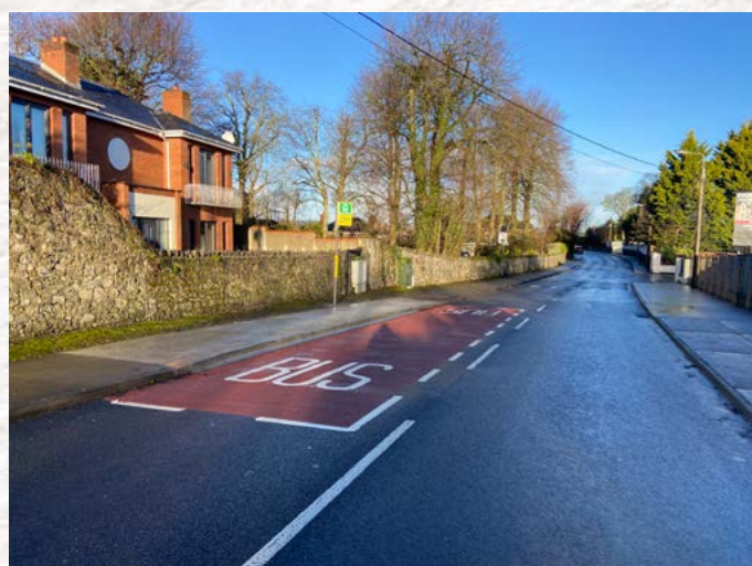
Bus stop enhancement at Golf Links Road
