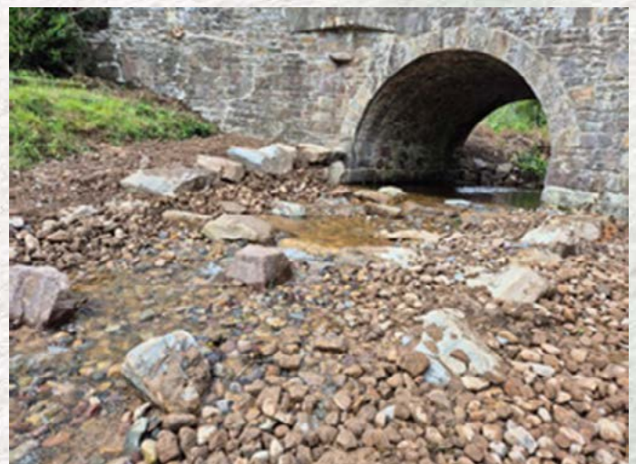
Structure B – R505 Toomaline Upper Bridge
