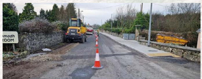
Footpath and Resurfacing works at Croom
