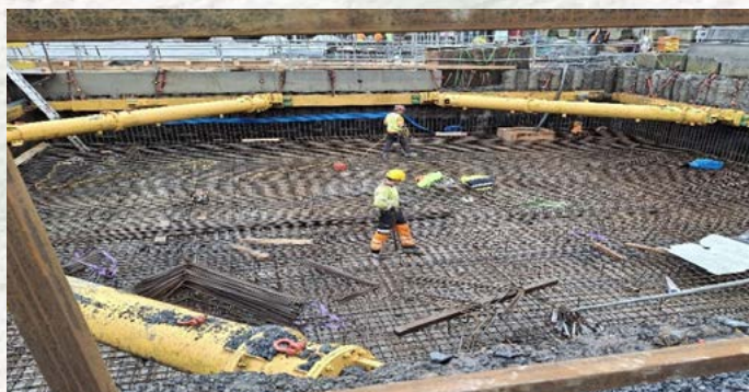
Steelfixing in Tidal Tank B
