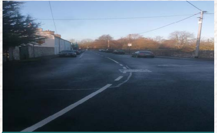
Restoration Improvement Scheme Works on L1413 Bruff
