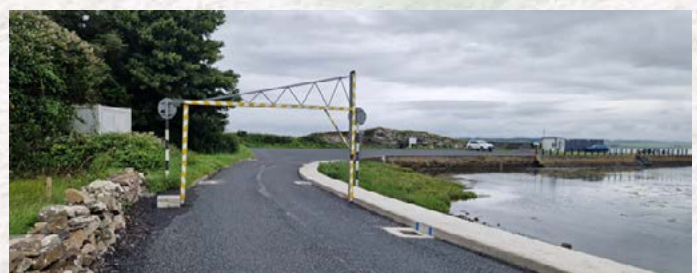
Resurfacing and Improvement works at Kiltteery Pier
