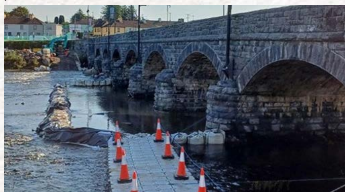
Refurbishment Works on Laune Bridge
