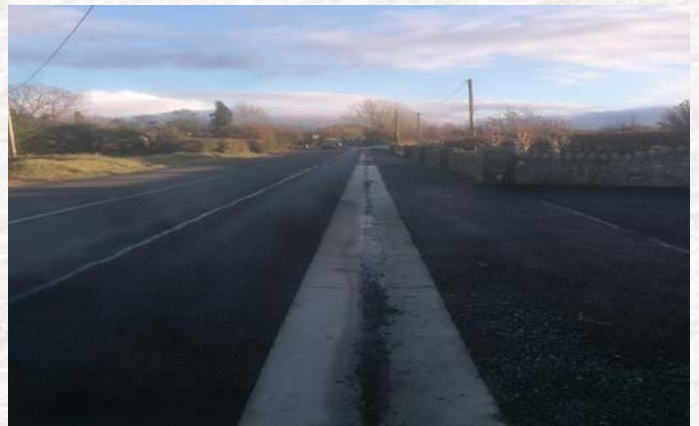
Drainage Scheme Works on R513 Knocklong
