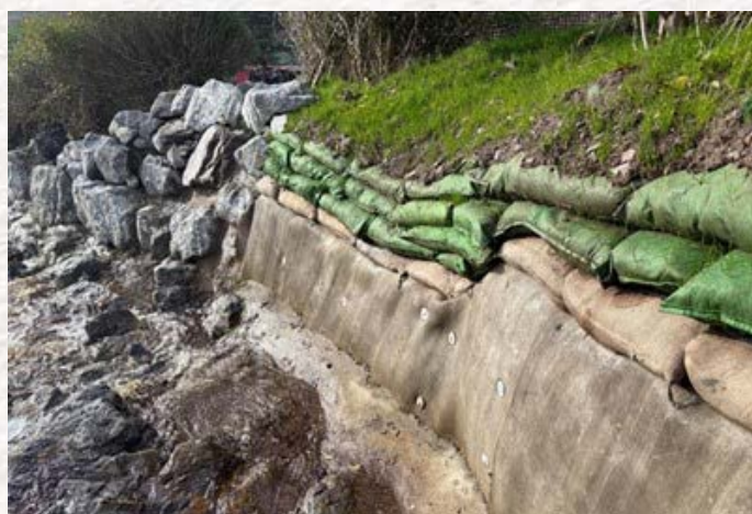
Embankment and Bridge Abutment Sytabilisation following flooding
