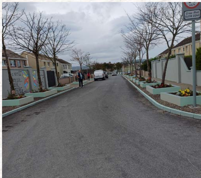
Hillview Drive Estate Enhancement Project
