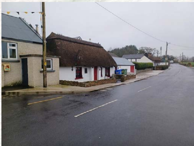
Footpath works at Ballyagran Village
