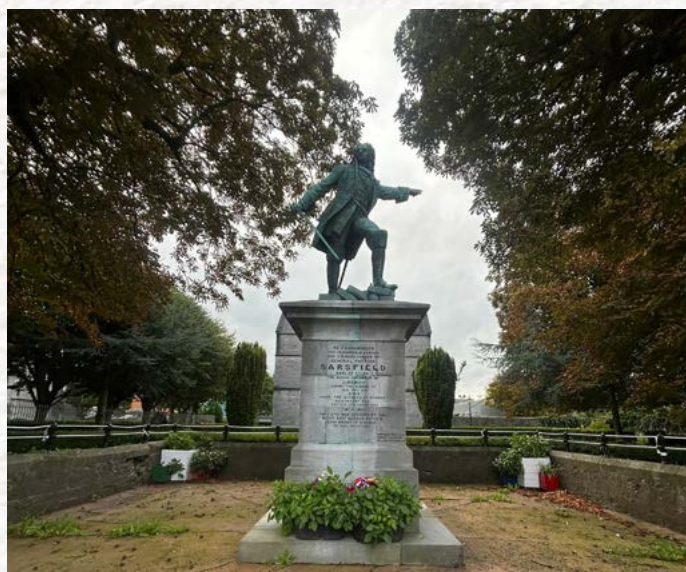
Sarsfield Monument, Cathedral Place before conservation works
