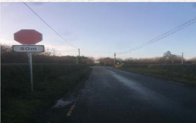
General Maintenance Safety Scheme Works R511
