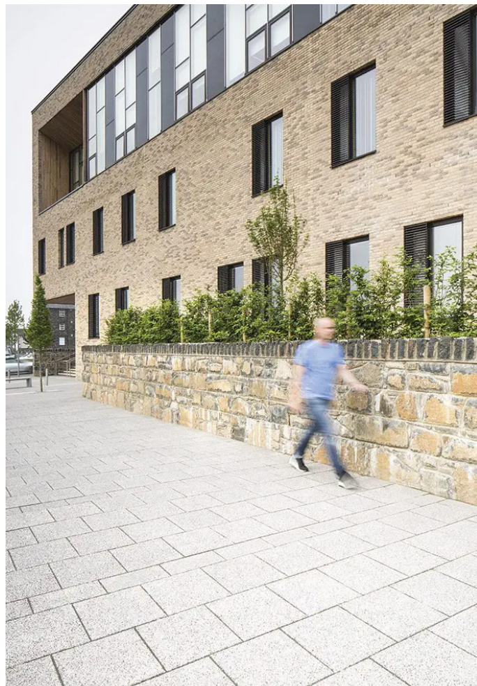
Example of pre-cast paving with natural stone aggregate surface (Credit: Acheson and Glover)
