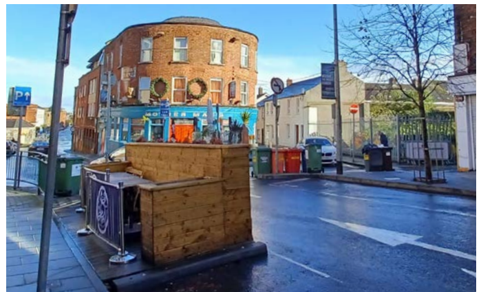
Parklet in front of protected building, High Street
