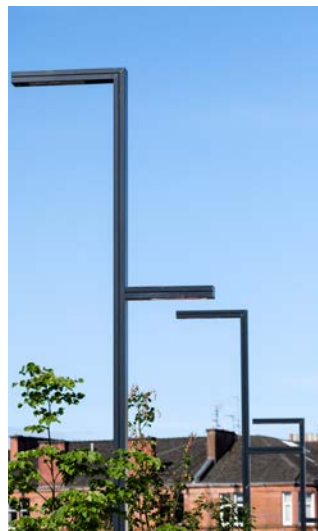
Dual headed columns, Glasgow University (LUC)
