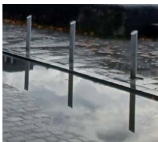
Chamfer steel CHS
