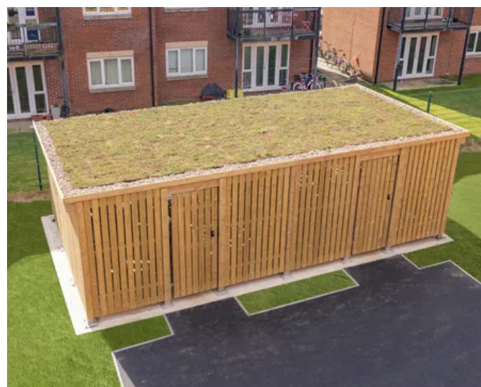
Green roof cycle shelter (Credit: Langley Design )
