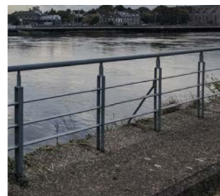
Painted steel with SHS supports
