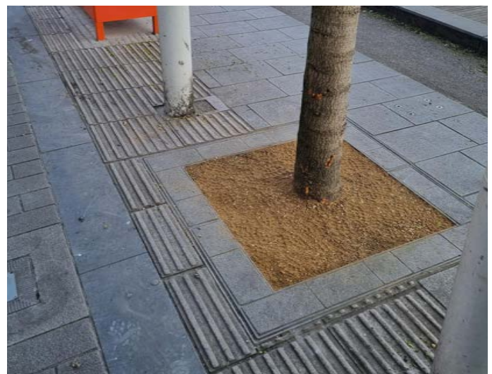
Bound Gravel Surface (Credit: LUC)
