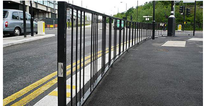
Guardrail with high degree of visibility (Credit: Store Fittings Direct)
