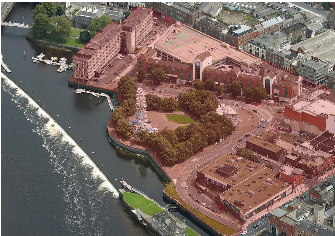
Existing aerial view
