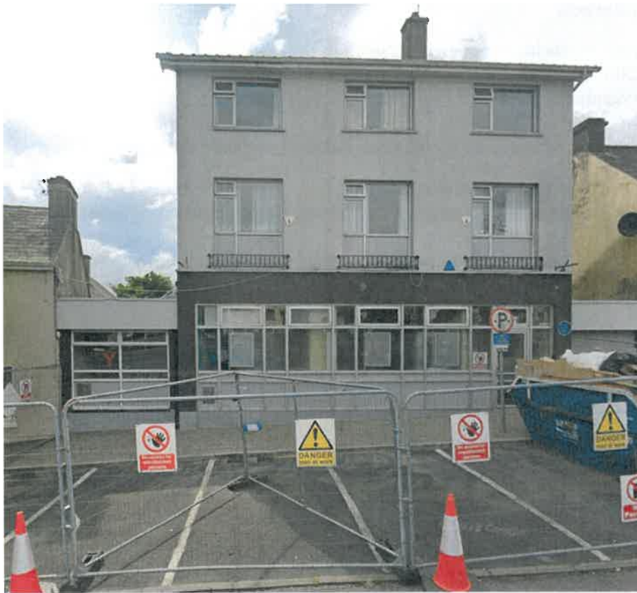
Plate 2 View of the site from The Square.
