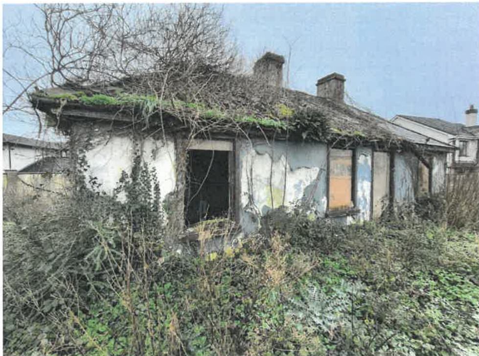
Figure 1: Existing Derelict Structure on site
