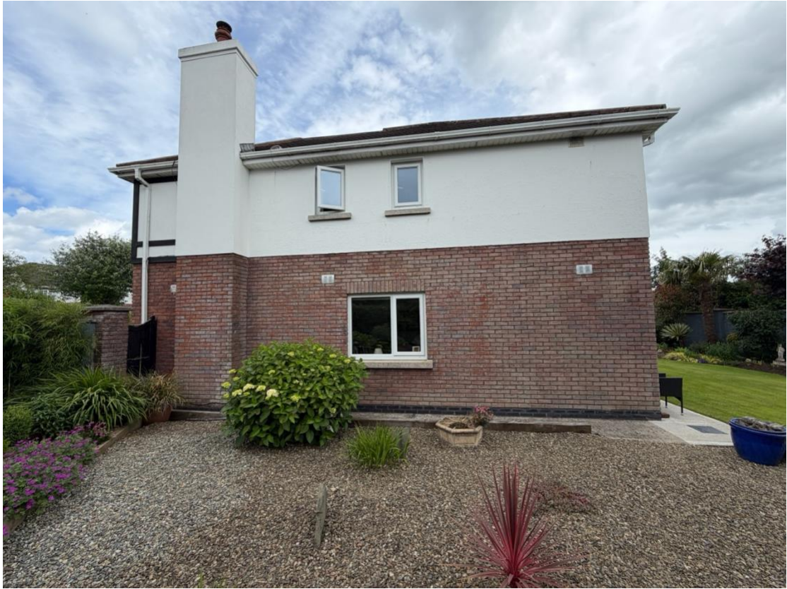
West side of house
