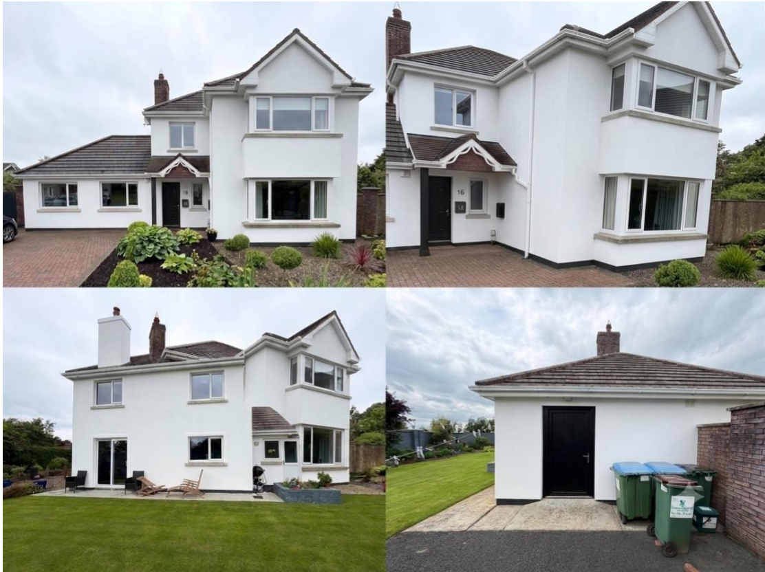
Image of House with EWI (External Wall Installation) installed
