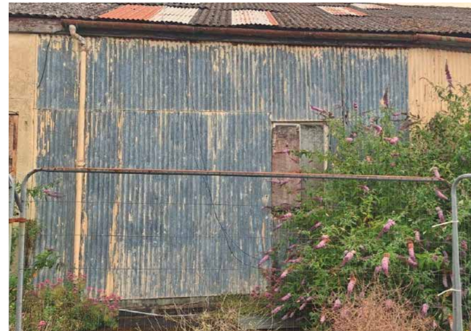
Corrugated metal sheeting This can be reused as cladding and roofing in various locations such as the bat houses
