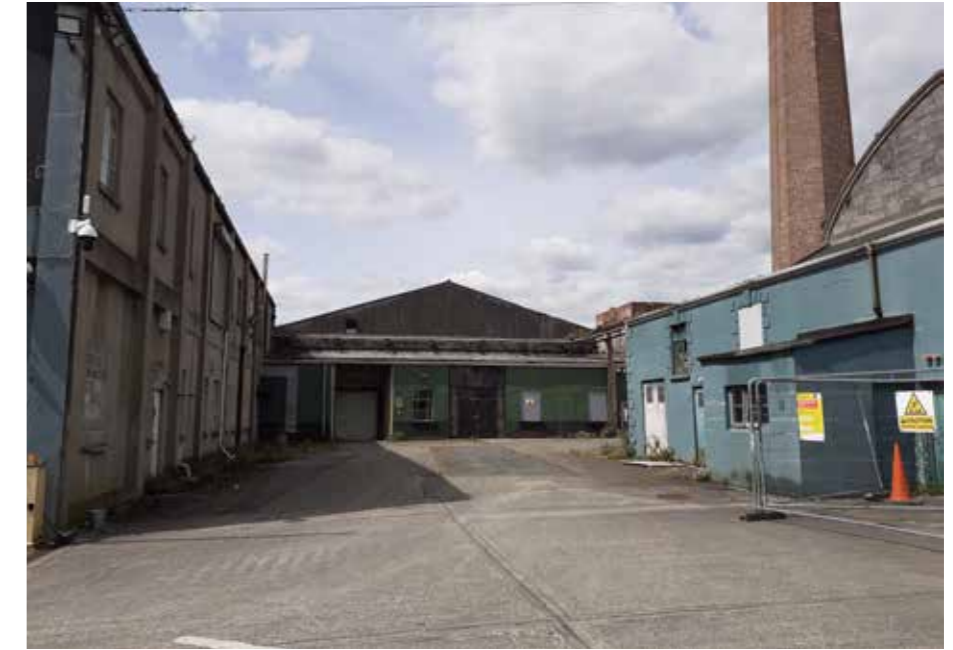
Areas on site with concrete in good condition are reused and inlaid.
