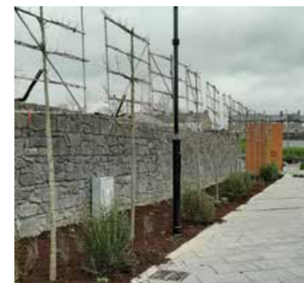
Limestone Mortar wall to North Circular Rd.
