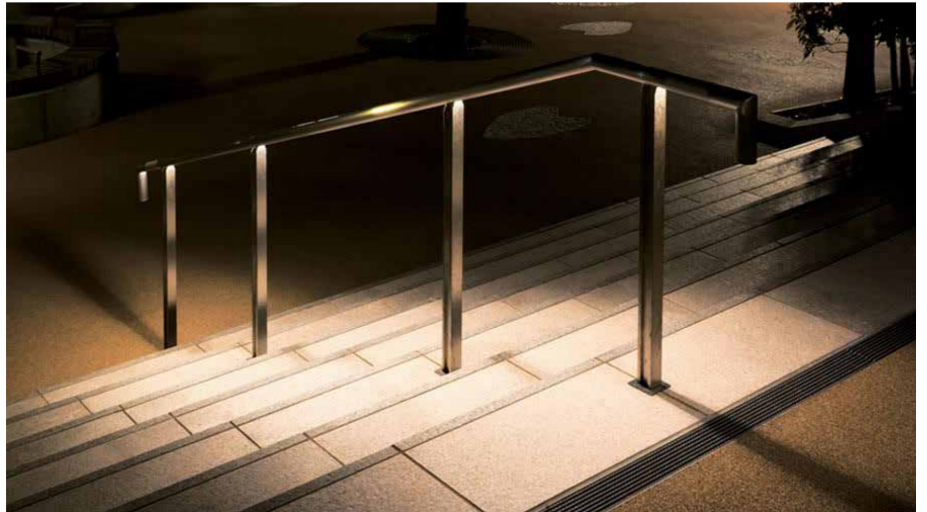
Recessed lighting to handrails to maximise safety on stairs
