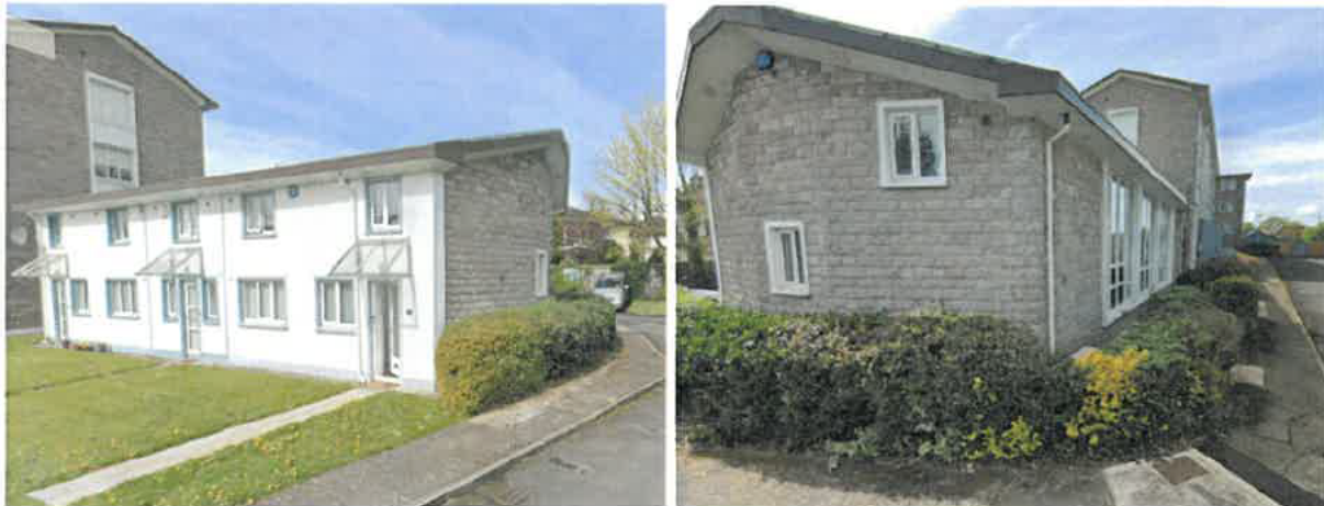
Figure 1: Images from front, side and rear of no. 22 The parc North Circular Road
