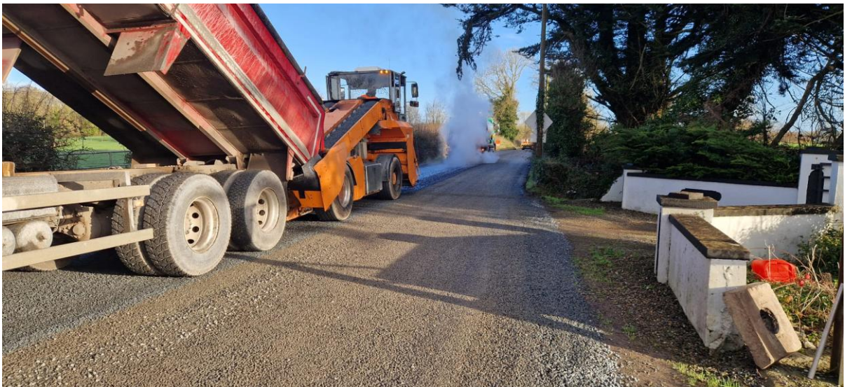
Road Sesurfacing Works as part of the 2026 Road Works Programme
