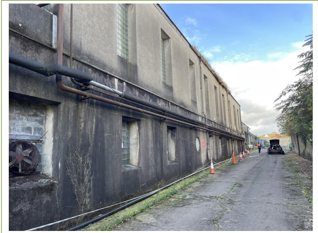
View of the asbestos cement gutters and downpipes on building 4
