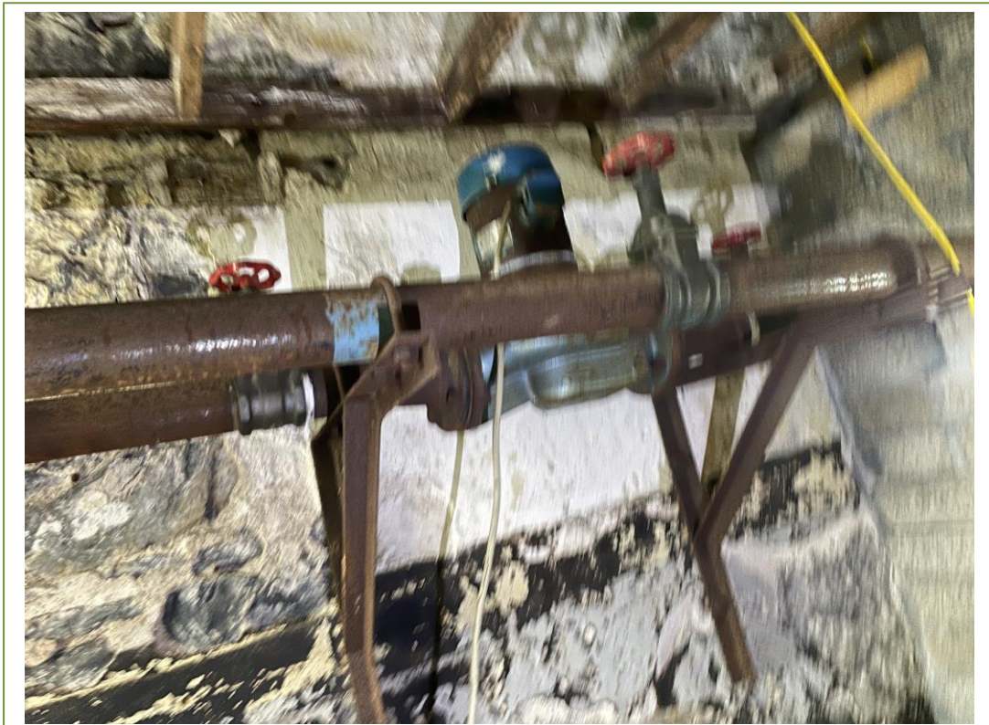
Rope on the pipework on the 3 rd floor in building 4
