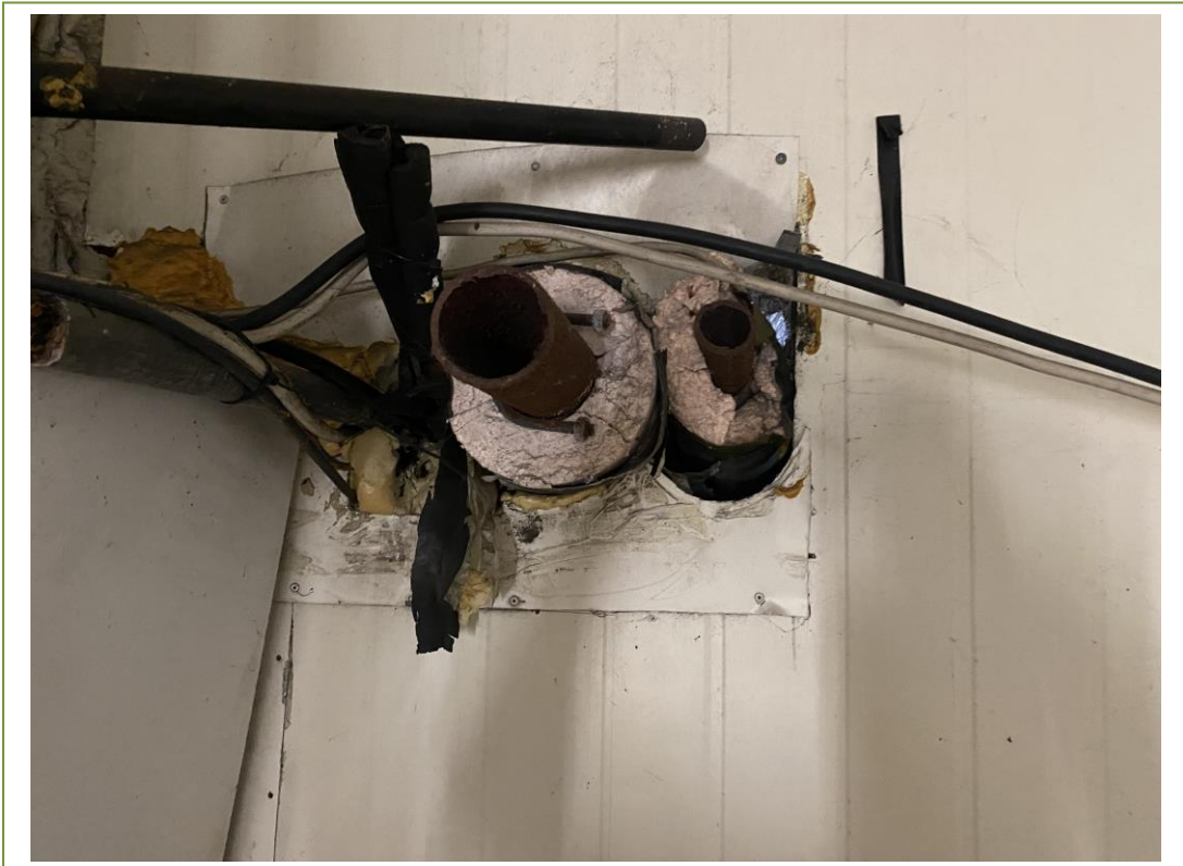
Pipework insulation sampled in building 5
