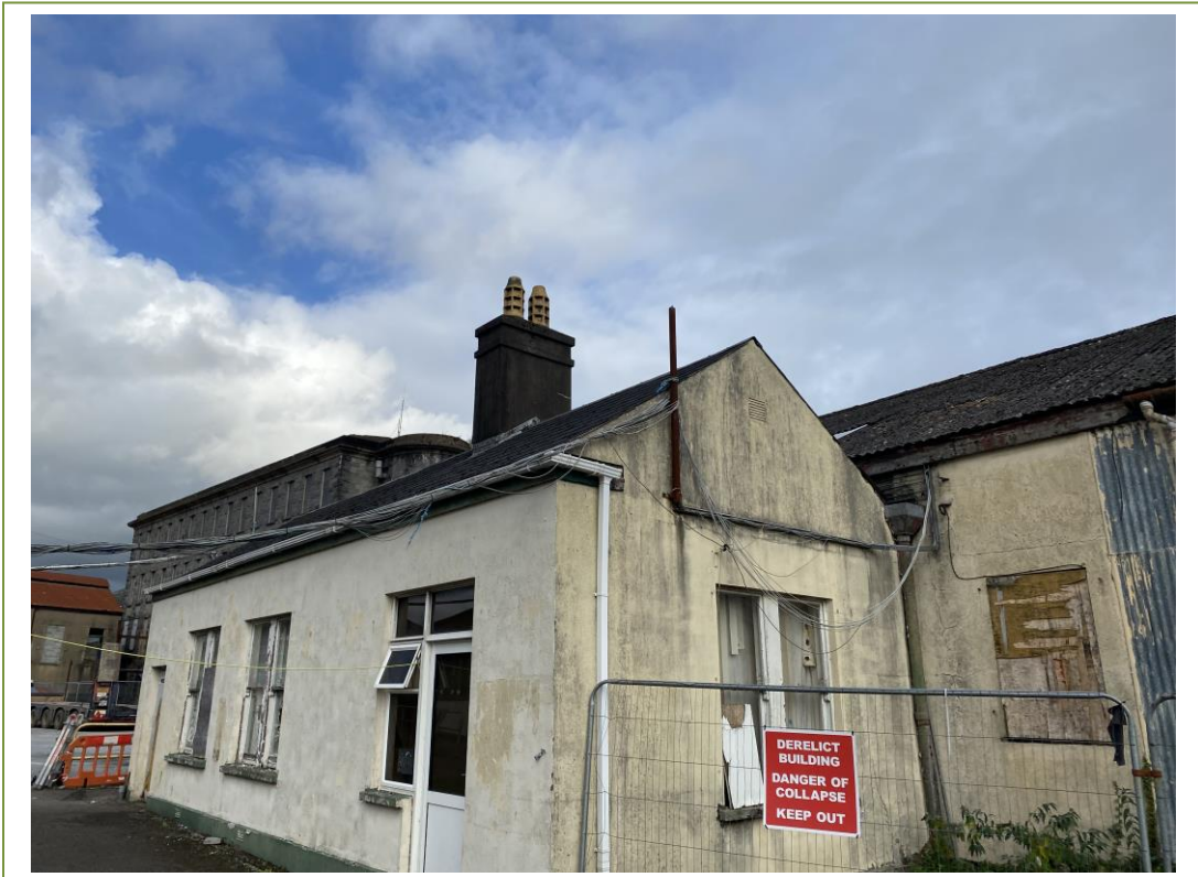
View of the side building which contains the asbestos cement slates
