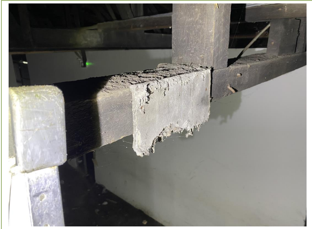
Closeup view of the remaining millboard on the lower level of the truss
