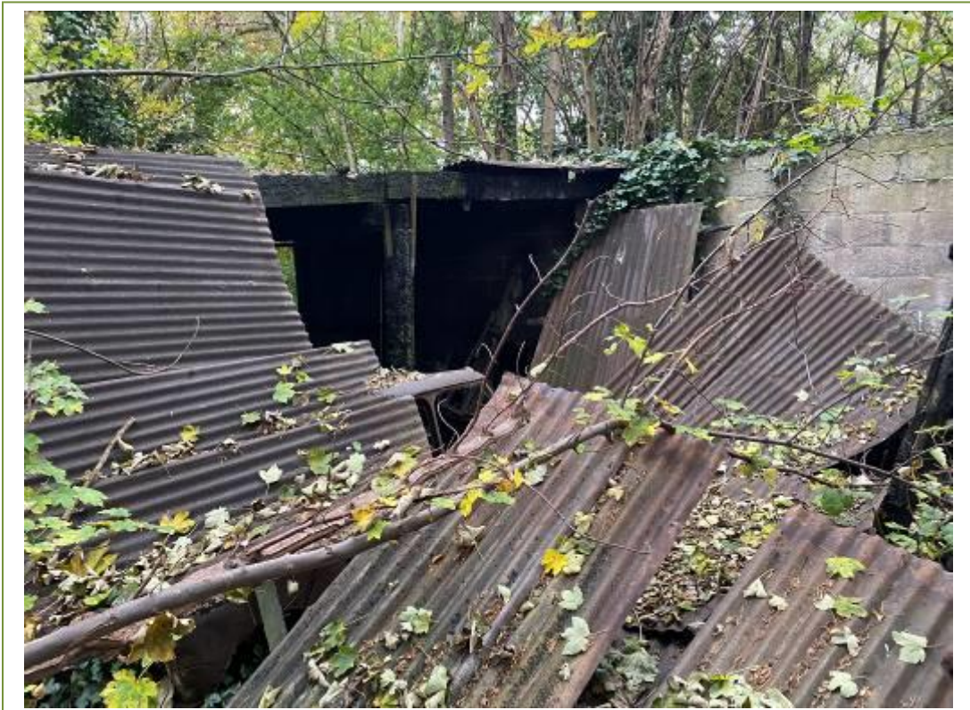
Metal cladding on the rear outbuilding
