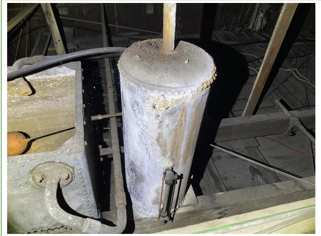
Coating sampled from the tank in the main attic of building 9
