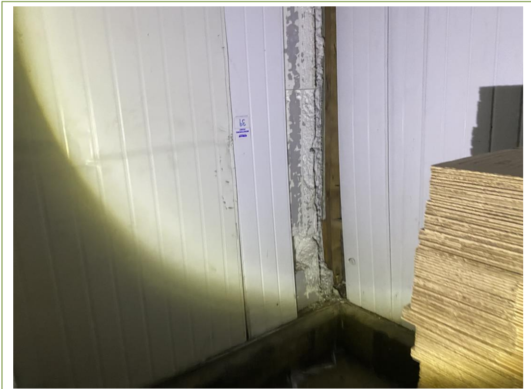
Polystyrene insulation in the wall panels of building 8
