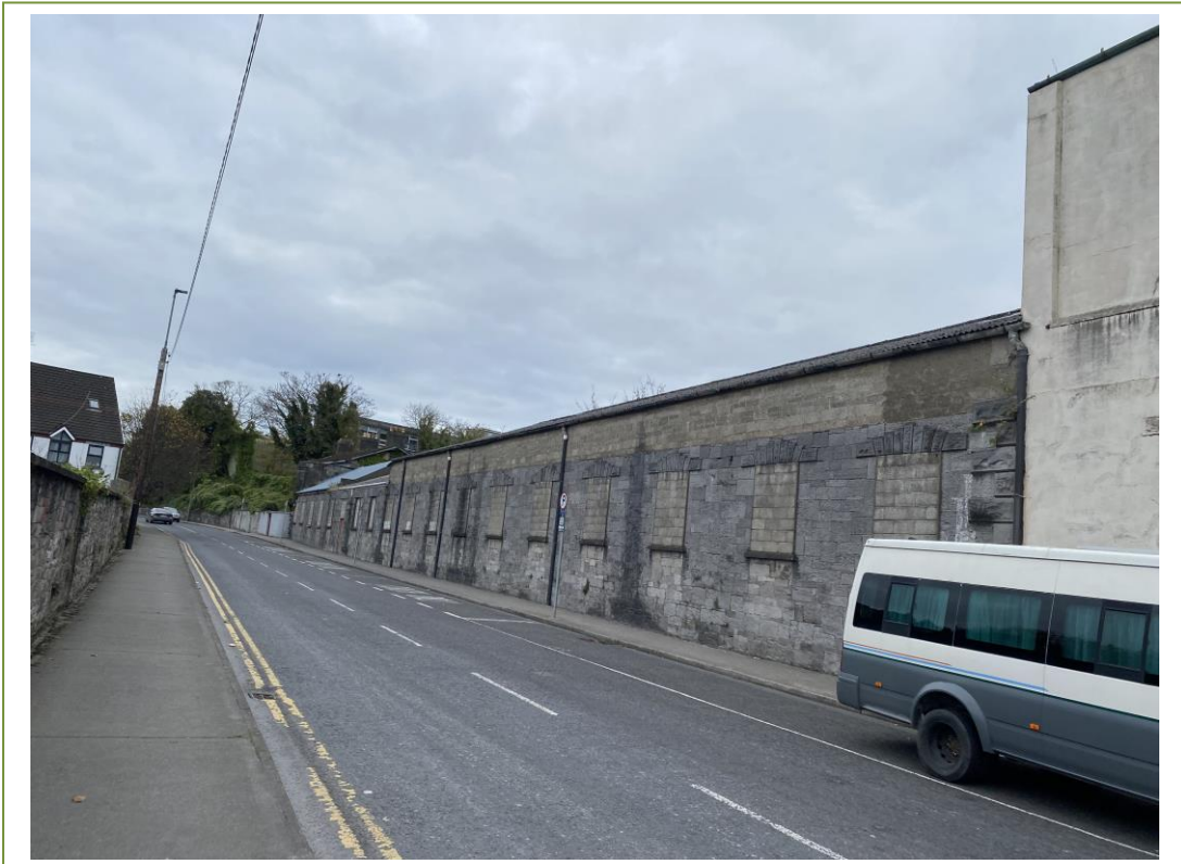
View of the asbestos cement gutters and downpipes on building 15
