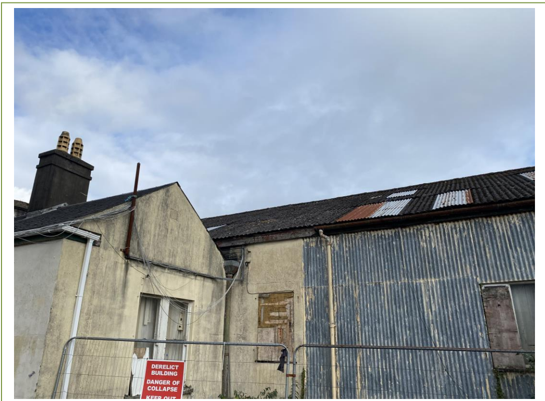
View of the asbestos cement gutters and downpipes on building 9
