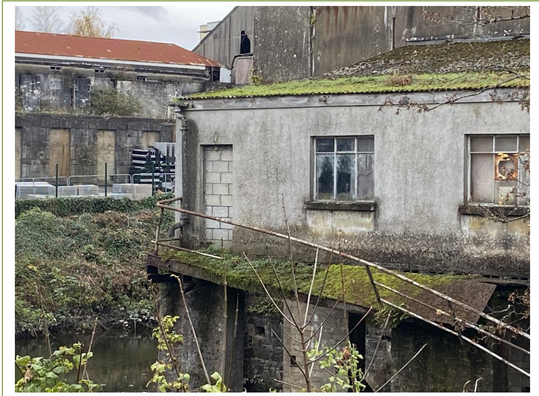
View of the asbestos cement gutters and downpipes on building 14
