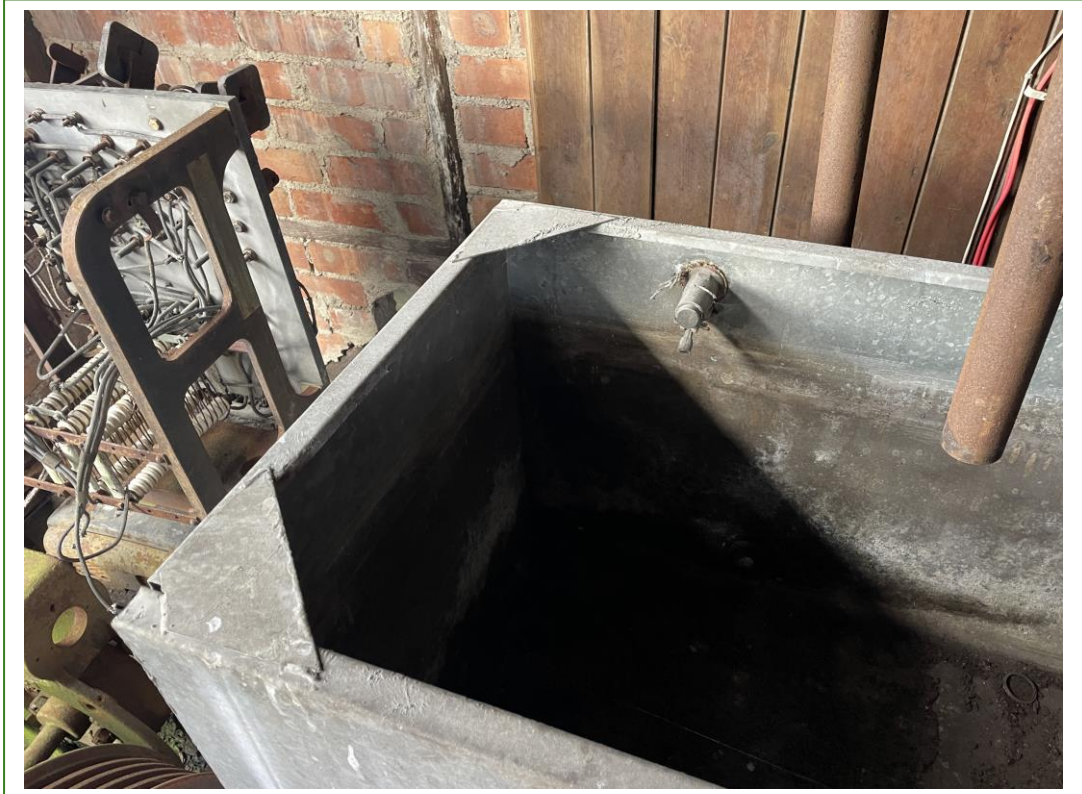
Rope on the tank in the attic in building 4
