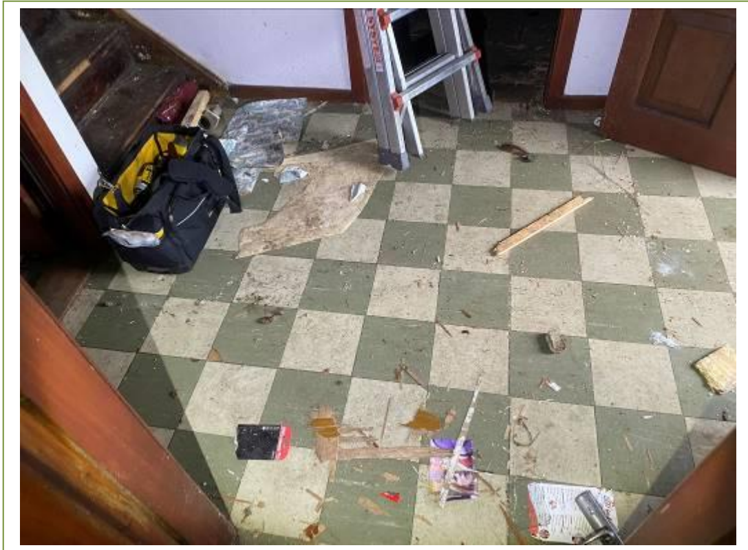
Floor tiles sampled from the hallway
