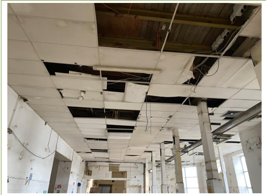
Plasterboard ceiling tiles in building 5
