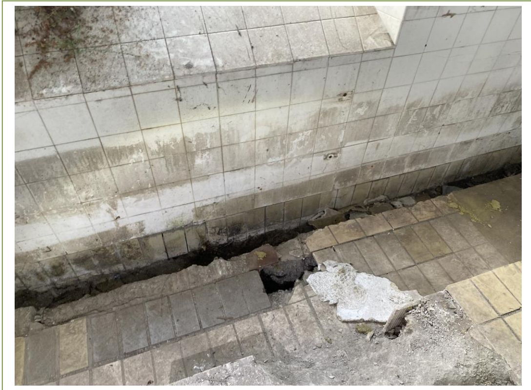
Ceramic floor tiles in building 5
