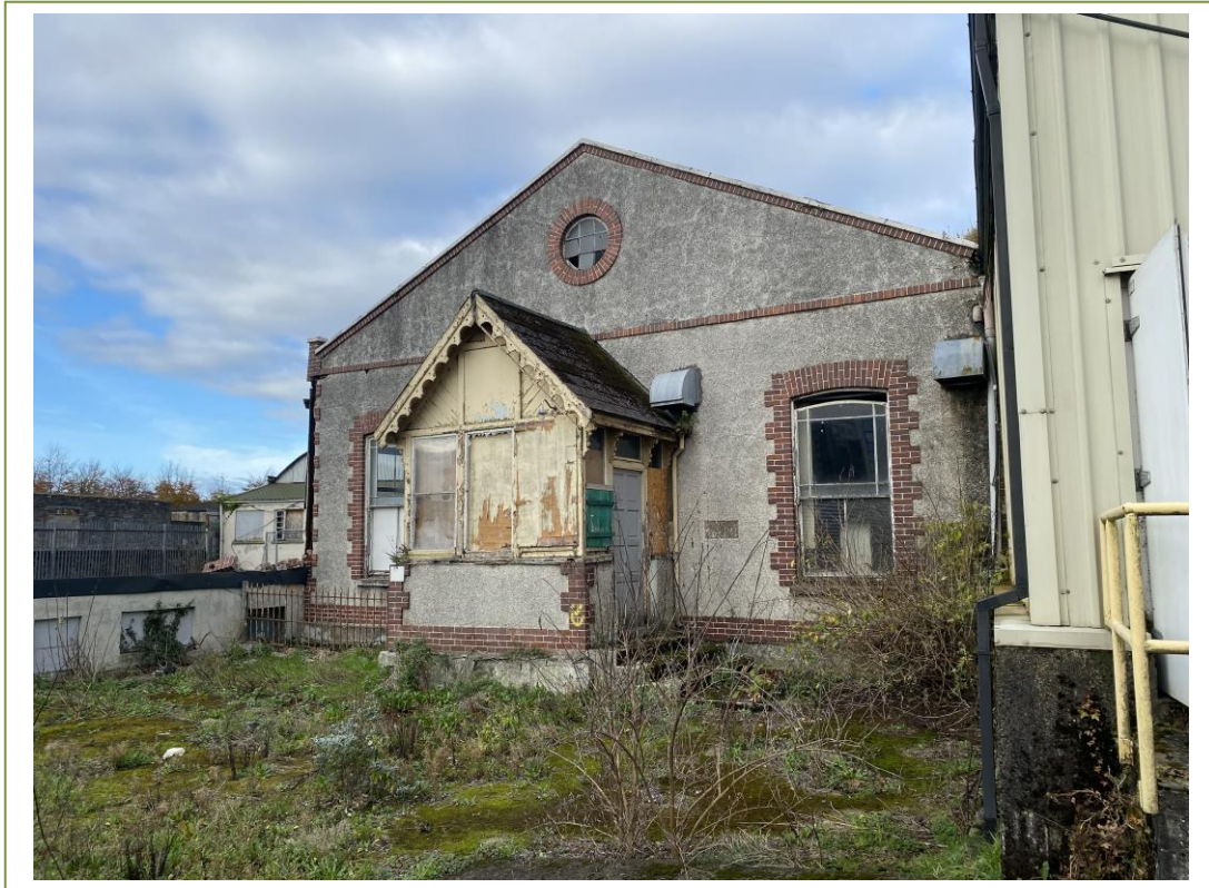
View of the slates on the rear porch roof
