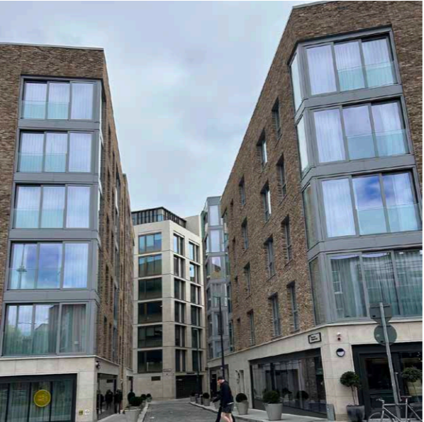
opposing & angled facades
