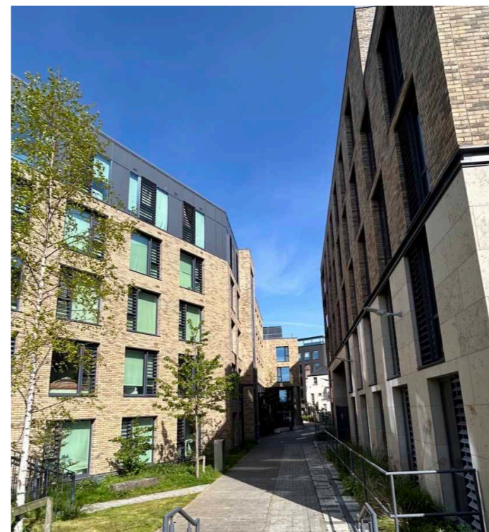
Opposing and angled facades
