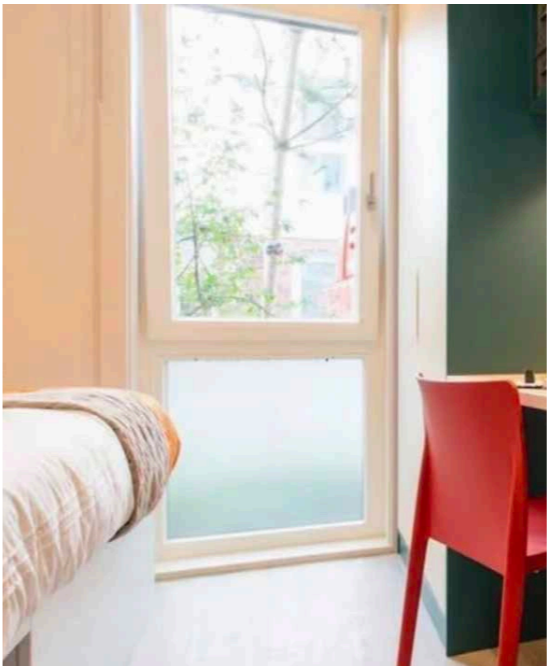
Ground Floor low level window with obscured glazing
