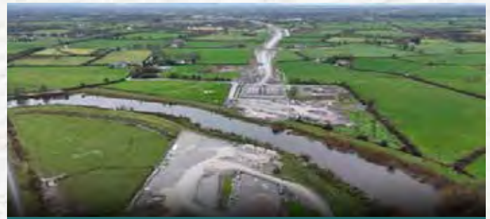
Beam installation complete at River Bridge M21-C3, over the Clonshire River and at underbridge UB07 over Local Road-L8025 in the background.
