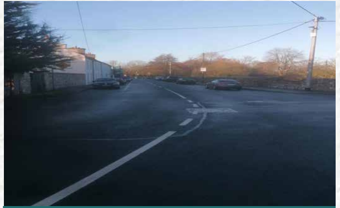
Restoration Improvement Scheme Works on L1413 Bruff
