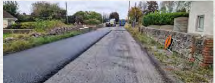
Road Overlay on the R518 between Rathkeale and Askeaton
