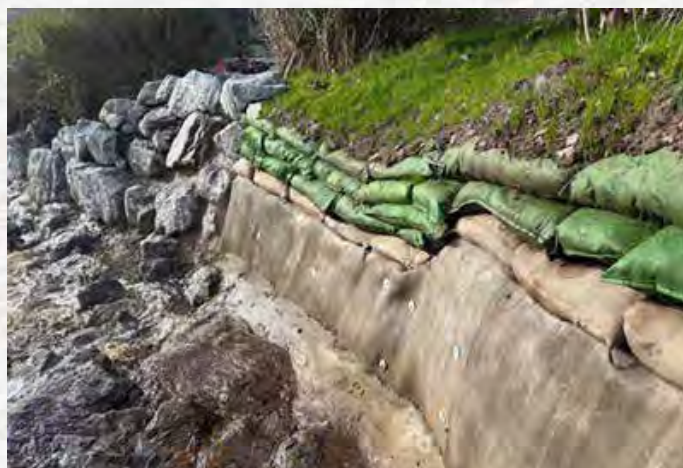
Embankment and Bridge Abutment Sytabilisation following flooding
