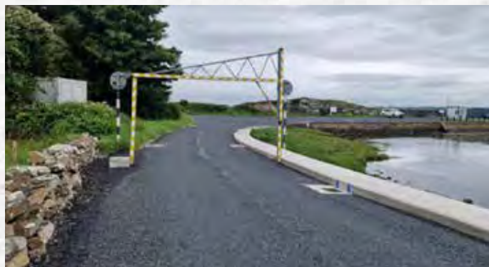
Surface Dressing Works Kiltteery Pier
