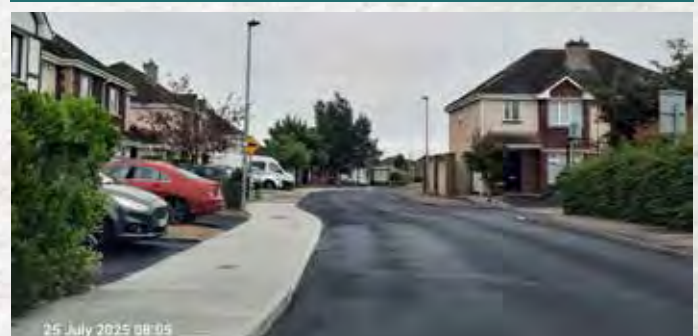
Upgrade works were carried out on Shannonvale footpath facilities, with unsafe sections replaced to enhance safety
