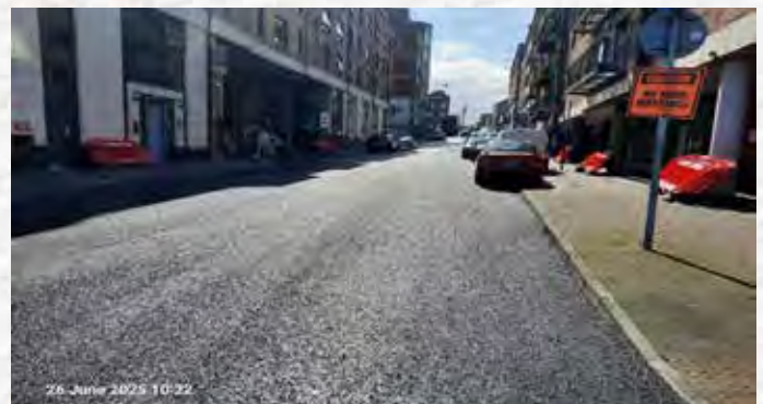
Mount Kenneth Road resurfacing
