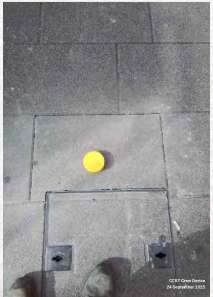
Footpath repairs City Centre
