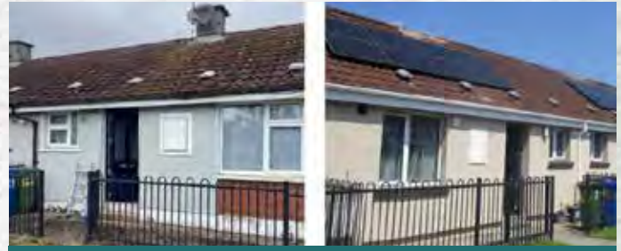
41 Canon Breen Park Thomondgate- Before and After EERP works
