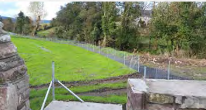
New link between Darragh Creamery Carpark and Molanna Loop Trail – funded under Outdoor Recreation Infrastructure Scheme
