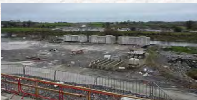
Aerial View of the River Maigue Bridge (RVB04) looking west
