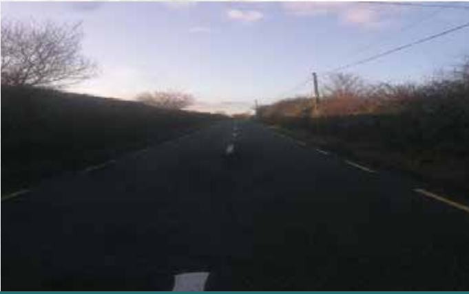
Surface Dressing Scheme Works on R511 Meanus
