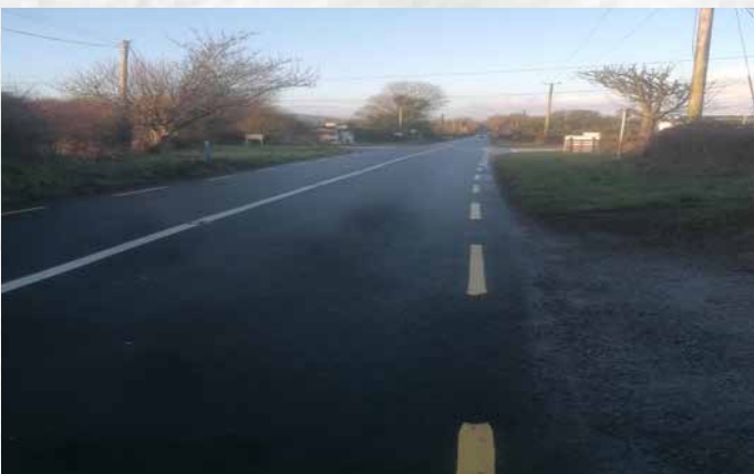
Road Reconstruction Works R516 Crean Cross
