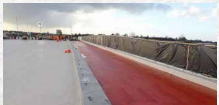
The Bridge Deck waterproofing of Ballygrennan Bridge has been completed with the remainder of Bridge works due for completion in Quarter 1 2026
