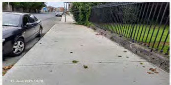
Old Clare Street Footpath Upgrade Works, where unsafe sections of the footpath were replaced to enhance pedestrian safety
