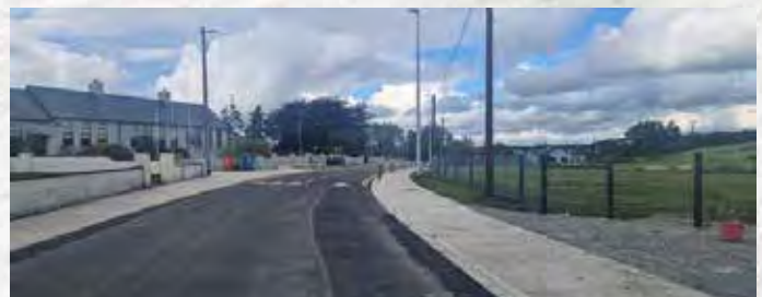
Active Travel Project near Loughill school
