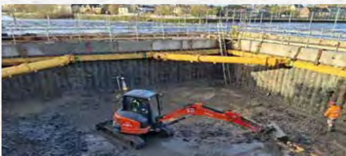
Tidal Tank B excavation
