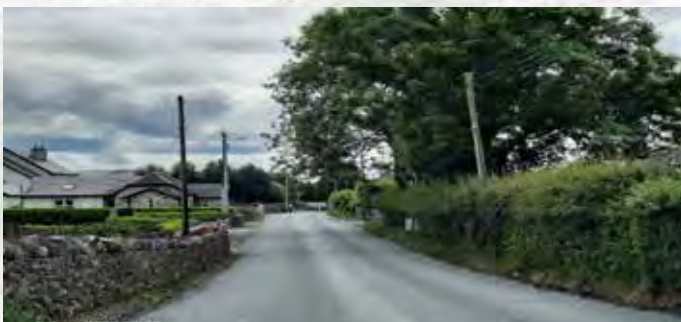
Clonnanna Surface Dressing Improvement resurfacing scheme involving a double surface dressing, delivered as part of the multi-annual road resurfacing programme
