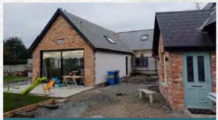
Vacant Property 1 – AFTER
