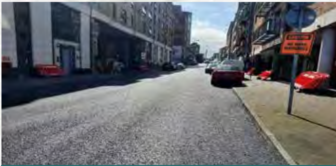
Mount Kenneth Road resurfacing scheme involving a macadam overlay, delivered as part of the multi-annual road resurfacing programme
