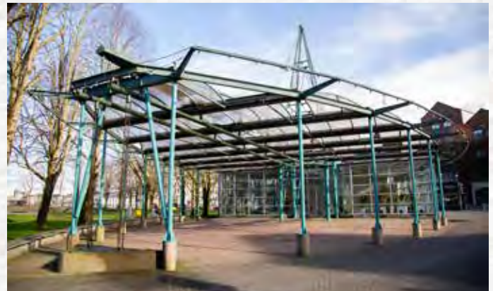
Former Tourist Office, Arthur's Quay – Current photograph
