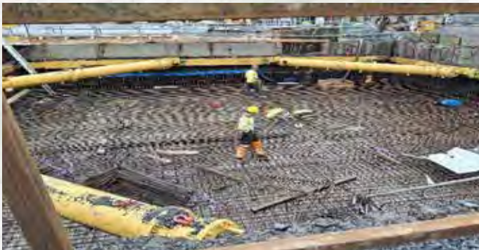
Steelfixing in Tidal Tank B
