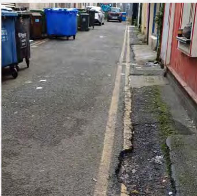
Limerick Lane before works
