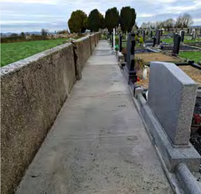
Effin Graveyard, Footpath Replacement Works
