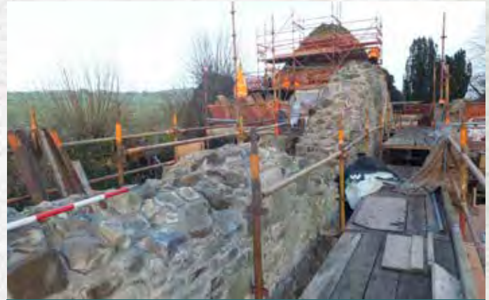
Community Monuments Fund works in progress on Galbally Medieval Church
