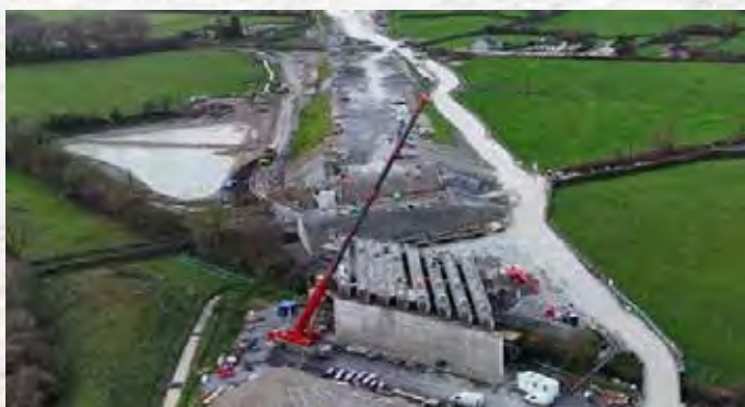
View of Eastern Central Piers of River Maigue Bridge (RVB04) looking west. Note plinths cast on top in preparation for steel girder placement in Quarter 2 2026.
