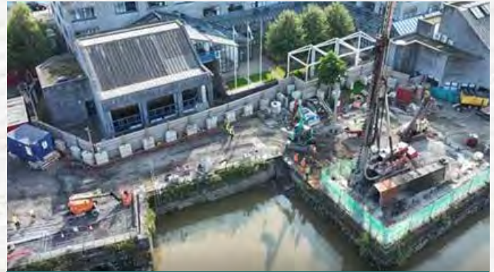
Piling at Civic offices
