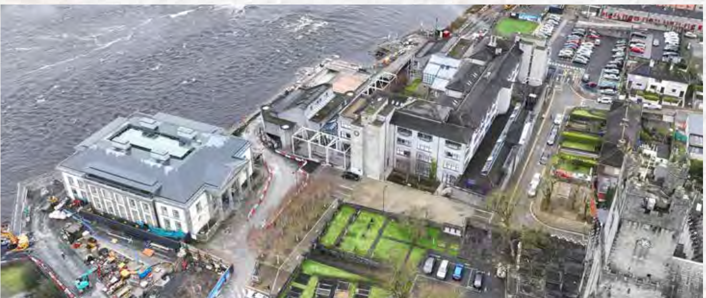
Aerial Photograph of Corporate Headquarters, Merchant's Quay
