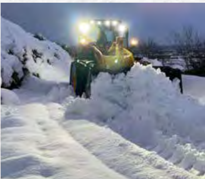
Snow Clearing Operation West Limerick NCW MD
