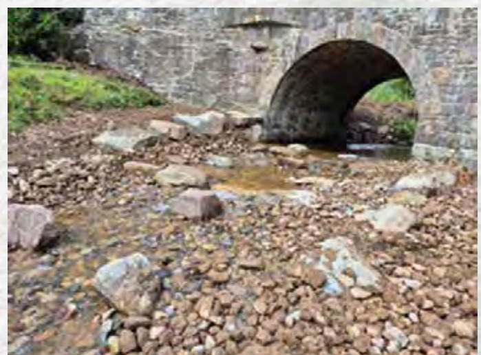
Structure B – R505 Toomaline Upper Bridge
