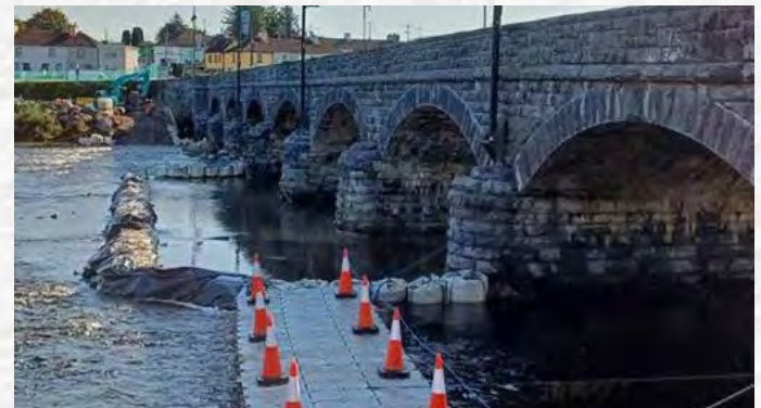
Refurbishment Works on Laune Bridge
