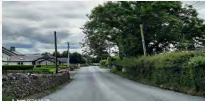
Surface Dressing Works Clonnanna
