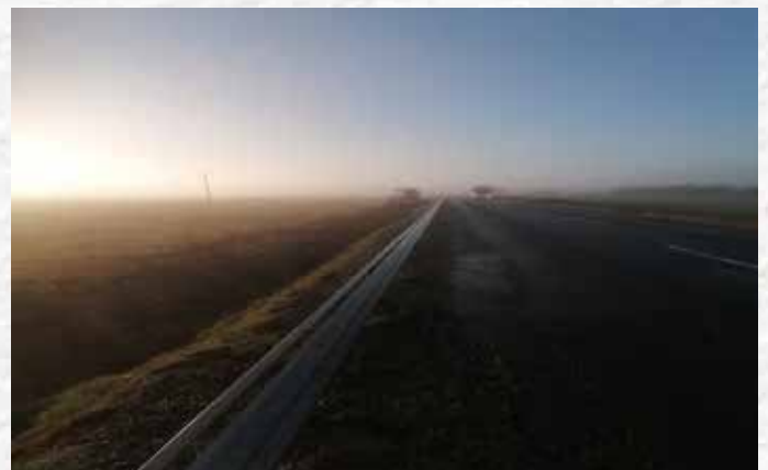
Low Cost Safety Scheme Works on R513 Rathjordan Herbertstown
