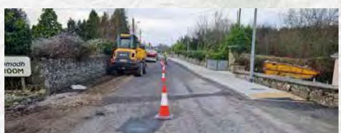
Footpath and Resurfacing works at Croom
