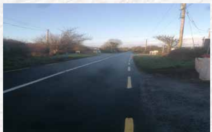
R516 Crean Cross Resurfacing
