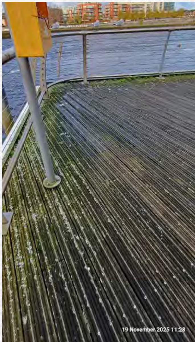
Cleaning the Boardwalk
