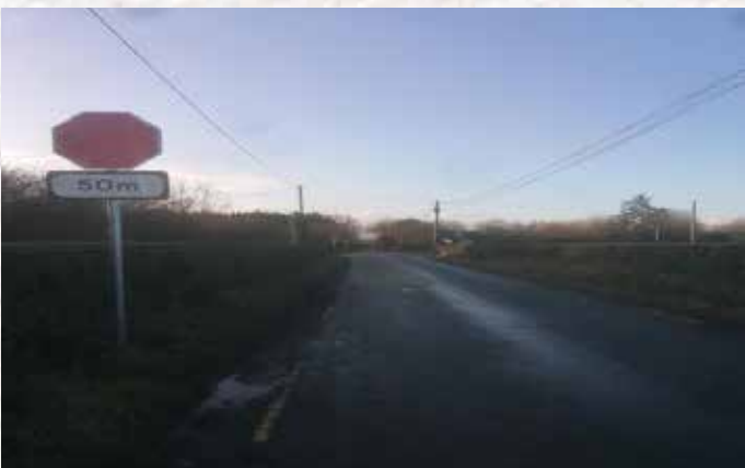
General Maintenance Safety Scheme Works R511
