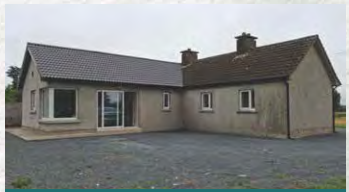
Vacant Property 2 – AFTER
