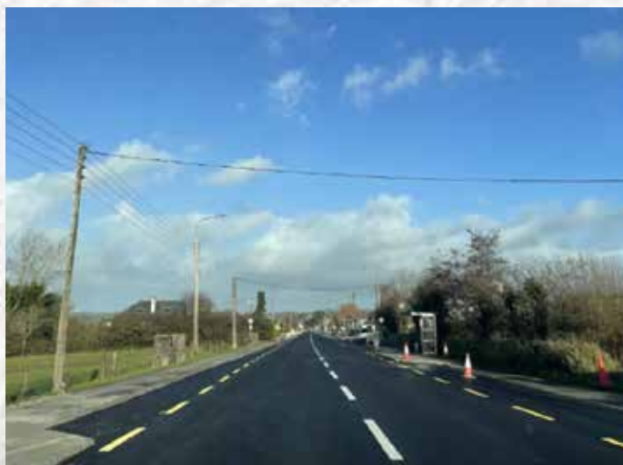
Abbeyfeale Western Approach Resurfacing
