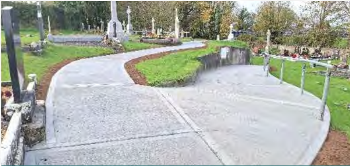
Castlemahon (Old) Graveyard, Footpaths and Boundary Fence Replacement
