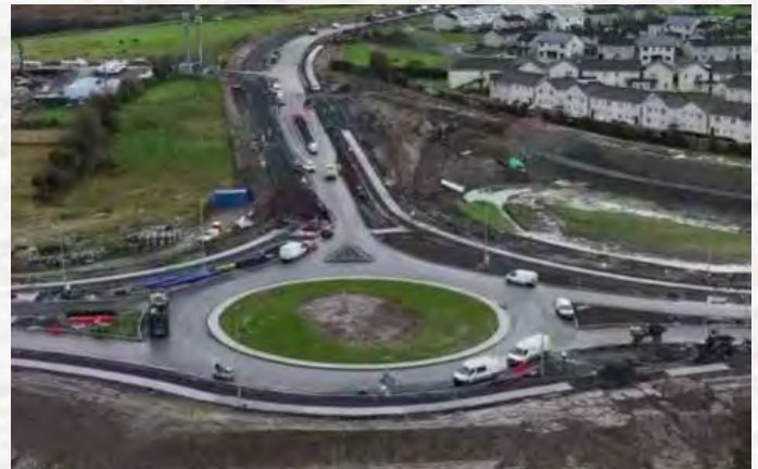
The newly constructed transformative Link Road into Moyross is nearing completion and due to open in Quarter 1 of 2026
