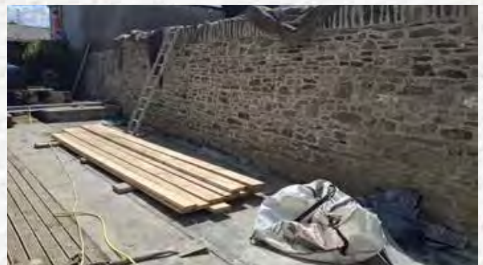
Abbeyfeale Old Burial Ground boundary wall from adjoining property
