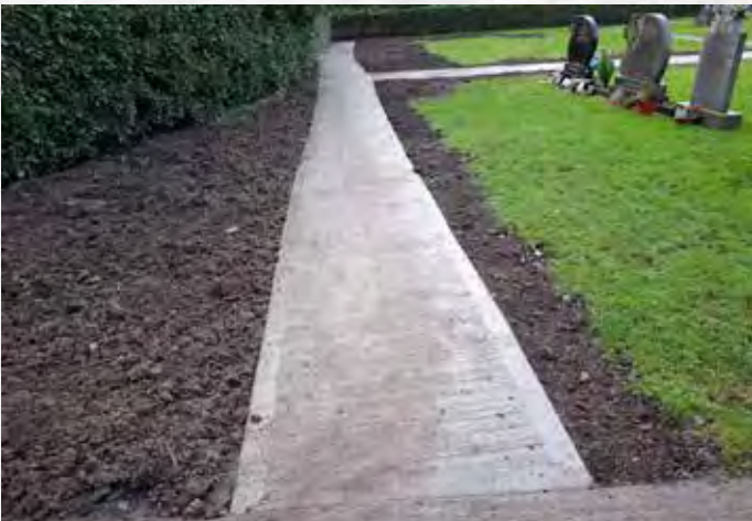
Caherelly Graveyard, Footpath Upgrade Works.
