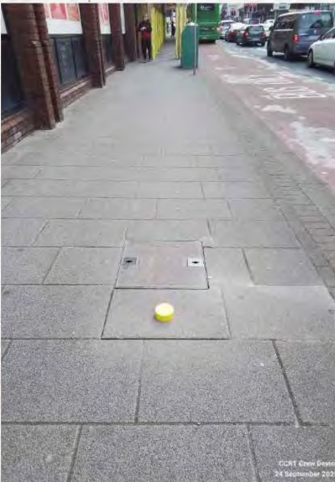
Footpath repairs City Centre
