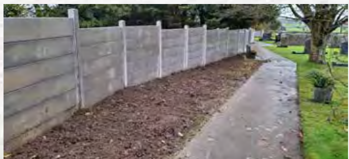
Saint Peter and Paul's Graveyard, Crecora following footpath repairs and boundary wall replacement.
