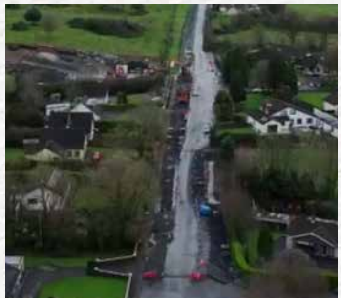
Works has commenced on the installation of the foul and storm sewer on the Cratloe Road
