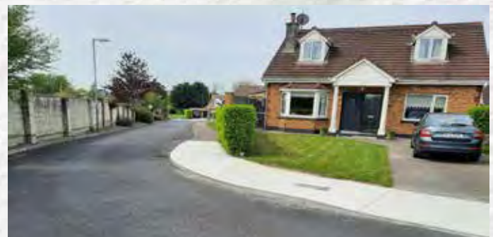
As part of the estate taking-in-charge scheme, unsafe sections of the footpath in Meadows, Corbally were replaced to improve pedestrian safety
