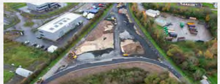
The Limerick Greenway Hub at Newcastle West Carpark Project – construction commenced September
