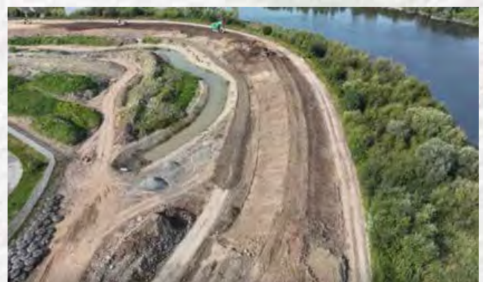
Embankment St. Marys Park
