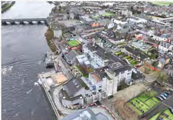
Aerial Photograph of Corporate Headquarters, Merchant’s Quay
