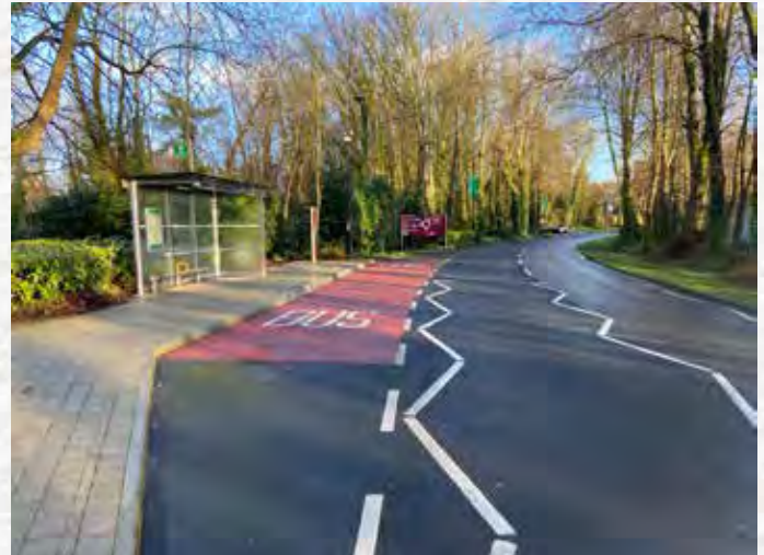
New bus shelter at University of Limerick
