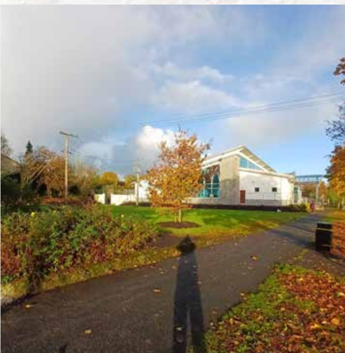
Askeaton Park Upgrade Works
