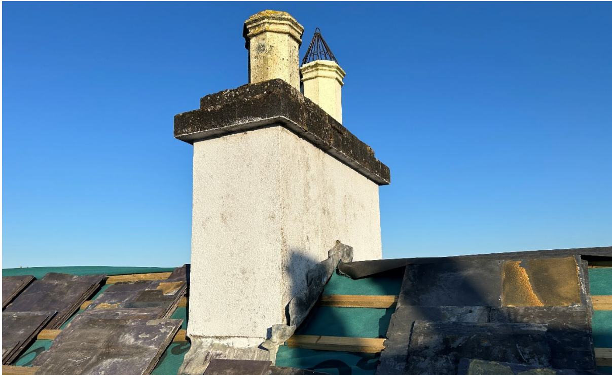
Figure 5: Chimney photographed during 2024 works.
