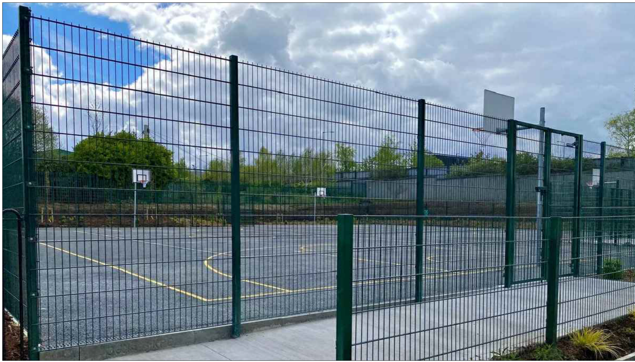
NK IBEX SUPREME 868 POST AND RIGID MESH PANEL SYSTEM. SCALE N.T.S.
