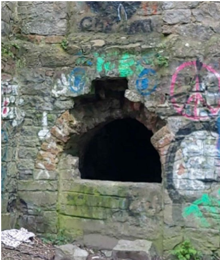
Figure 3.4 The hole in the wall of the tower to be infilled
