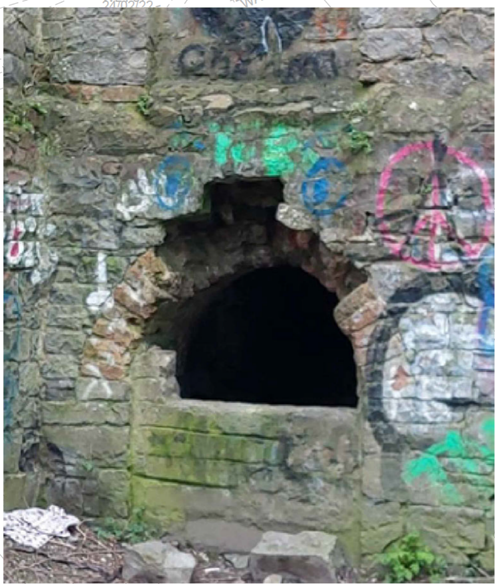
PHOTO OF EXISTING OPENING TO BE INFILLED
