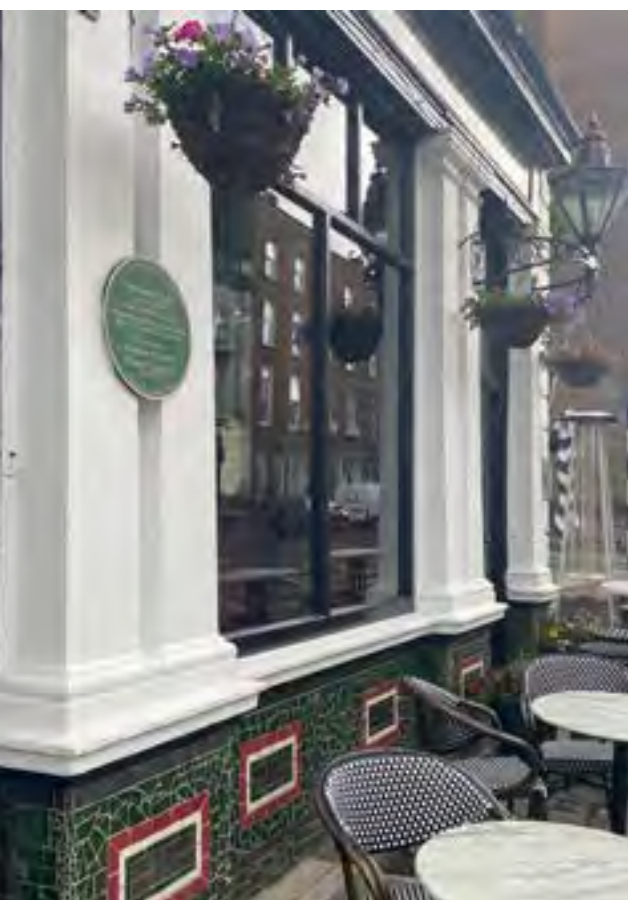
Figure 57 The White House, Limerick Mosaic tiled shopfront stallriser with plastered pilasters
