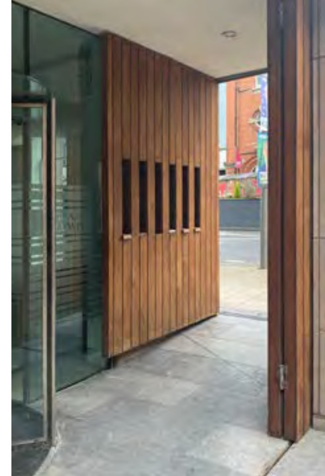
Figure 72 Glass Lewis & Co., Henry St, Limerick Timber security shutters fold into the reveal including a glazed entrance elevation
