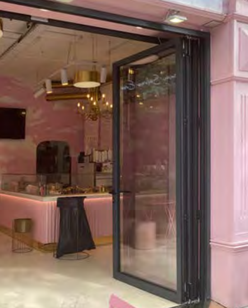
Figure 67 Cloud 9, Dublin. Contemporary shopfront with fully opening folding doors and an internal security grille. Example of a modern shopfront.
