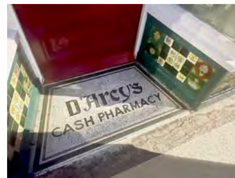
Figure 91 N. Rainsford Grocer, Doon. Example of good threshold surfacing in a recessed entrance with great accessibility for all
