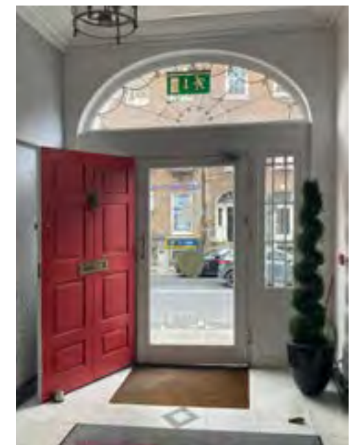
Figure 75 Georgian door security nocturnal shutter with a modern glazed door at the entrance. An example of providing security while also preserving the important traditional features of the building.
