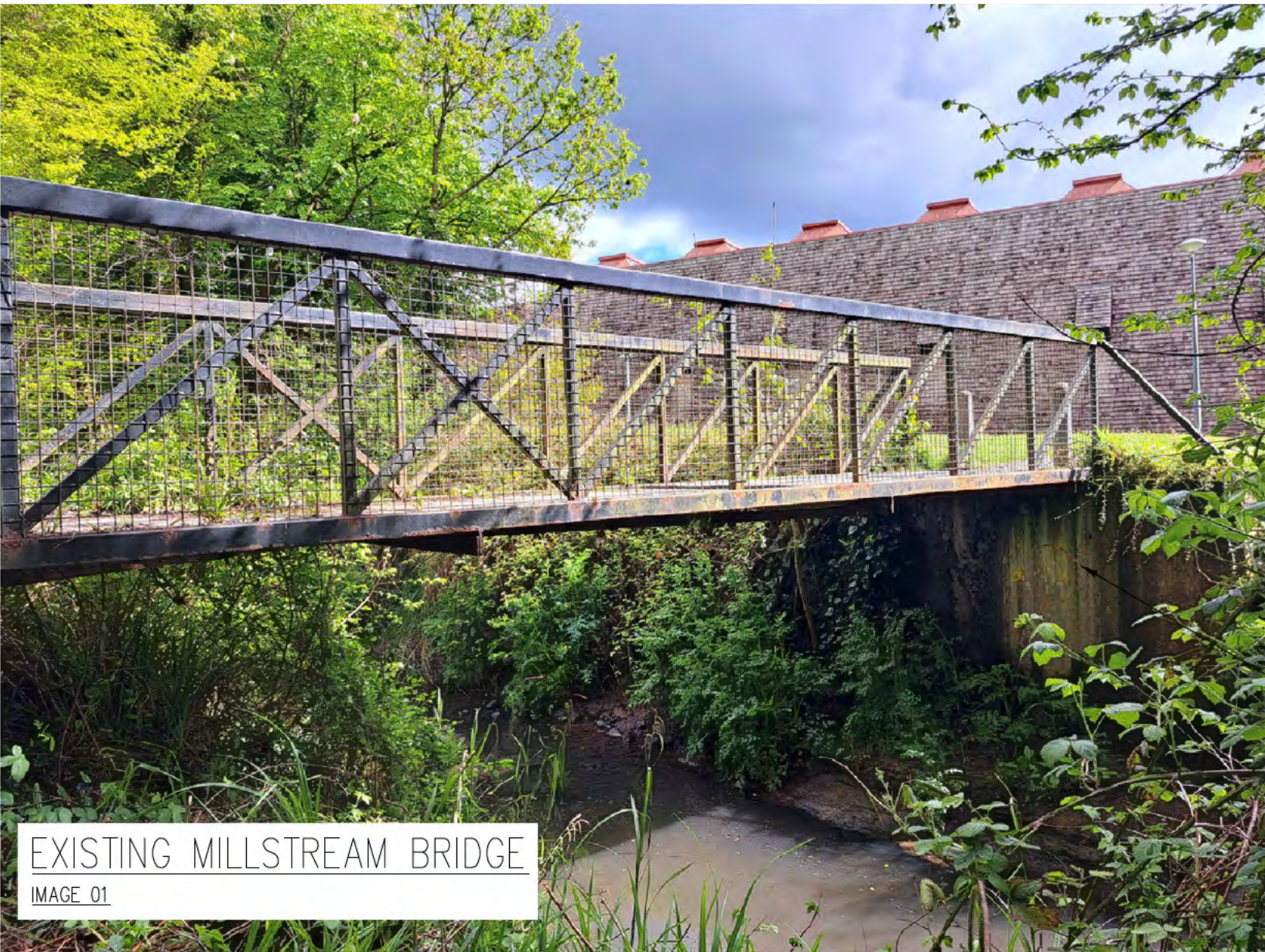
EXISTING CONCRETE HEAD WALLS SUPPORTING THE BRIDGE ON EITHER SIDE OF THE WATER CHANNEL.
