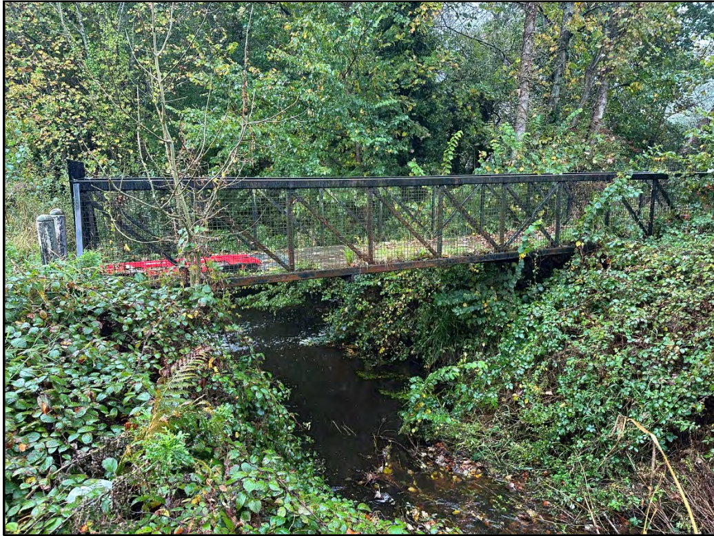
Plate 1: The existing bridge is a lightweight structure bolted to existing concrete piers. Viewed from the east.
