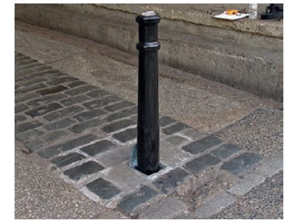
Telescopic or folding bollards with padlocks could be used to restrict private access while maintaining emergency or servicing access
