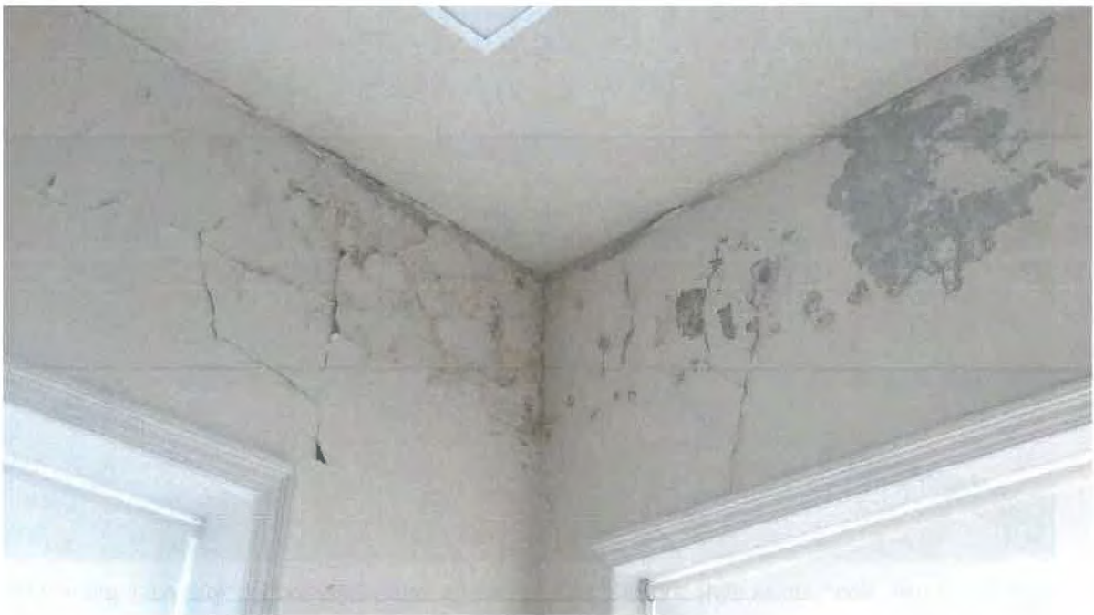
Photograph 042. South-West back corner top floor dampness due to gutter / lead bed leakage.
