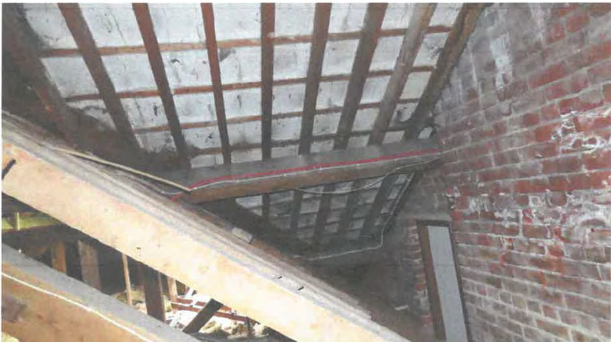
Photograph 020. Typical valley, jack rafter, common rafter & purlin intersection.
