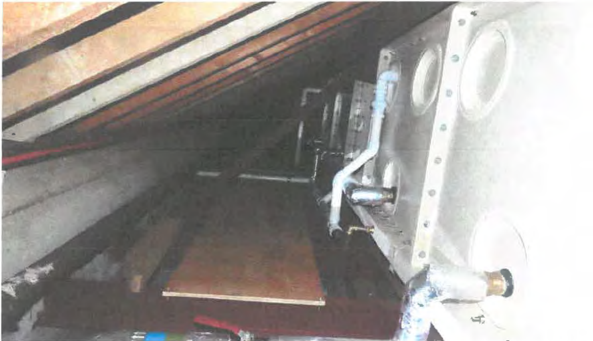
Photograph 039. North annex attic showing steel angle trusses, timber rafters, raised wall plate level over ceiling joist & water tank to the right.
