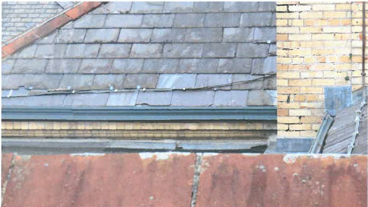
Photograph 025. Typical lead clip repairs due to slipping slates. Note clay hip tiles.
