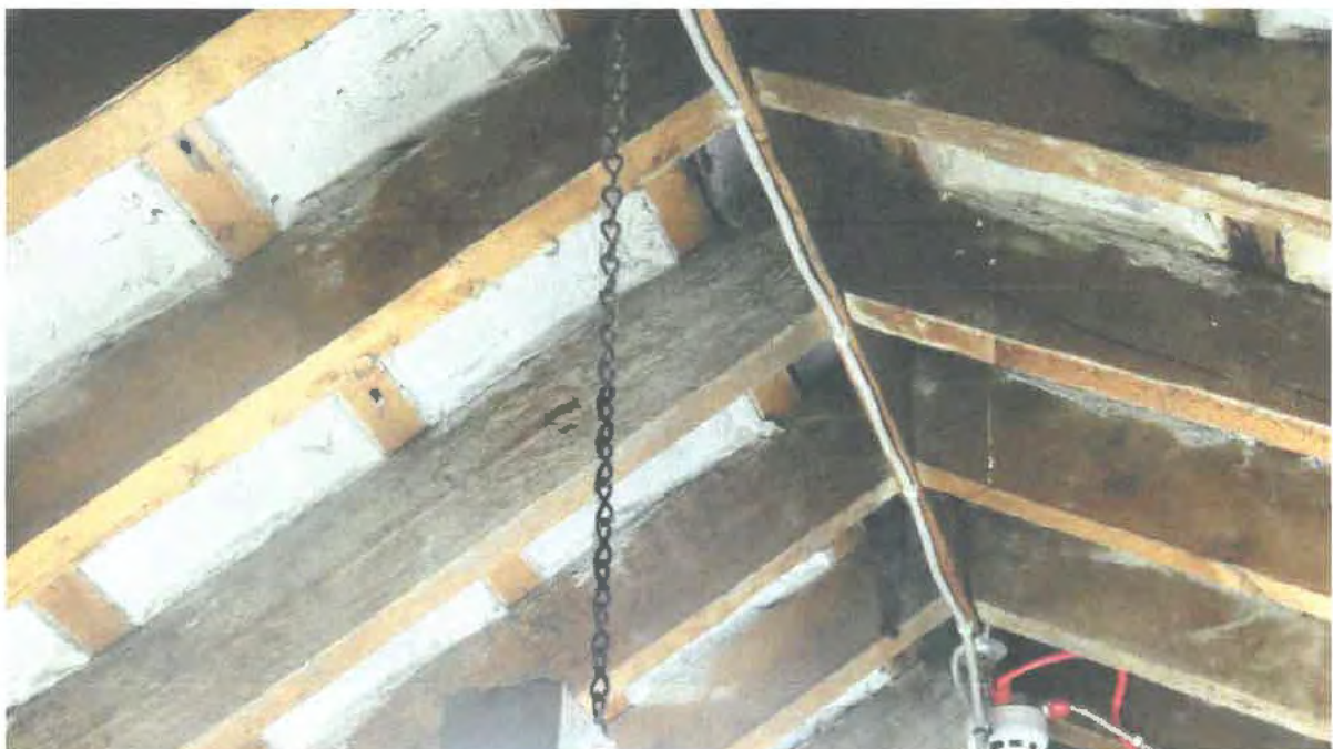
Photograph 014. Ridge board, common timber rafter, slating battens & lime parging.
