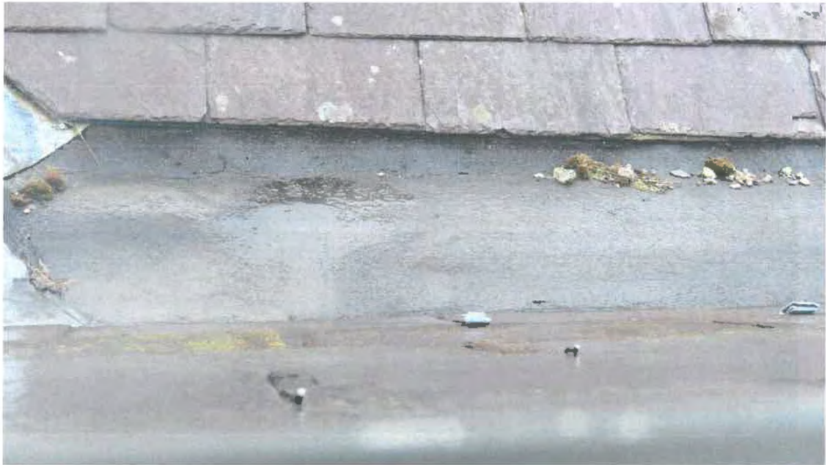
Photograph 033. Cracks in asphalt flat gutter annex building valley.
