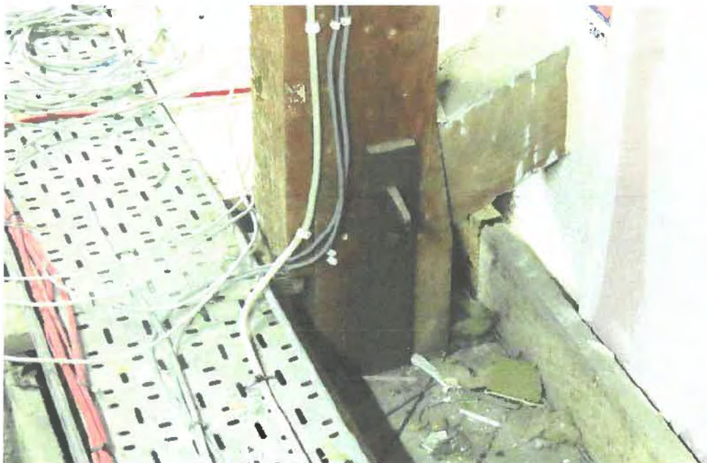
Photograph 012. Queen post with typical wrought iron stirrup.
