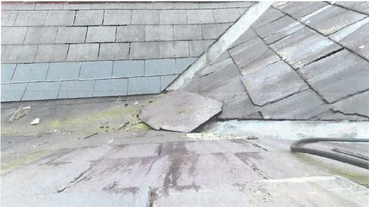
Photograph 023. Slipped slate in valley gutter & new repairs to annex building, check for asbestos.
