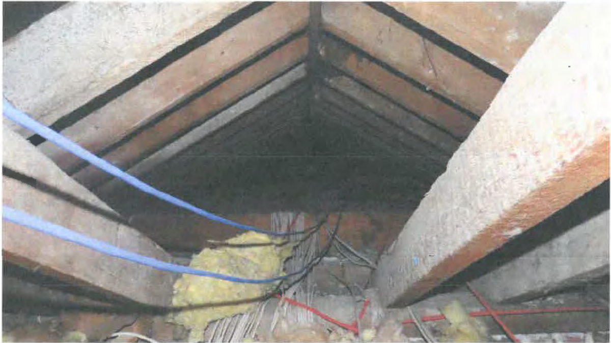
Photograph 017. Ridge board, common timber rafter, in annex building to the rear of the main building attic photograph.
