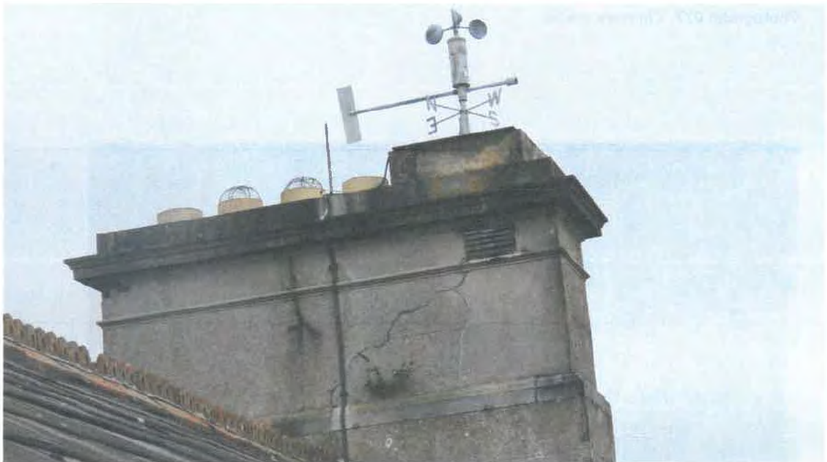
Photograph 030. Chimney cracks.
