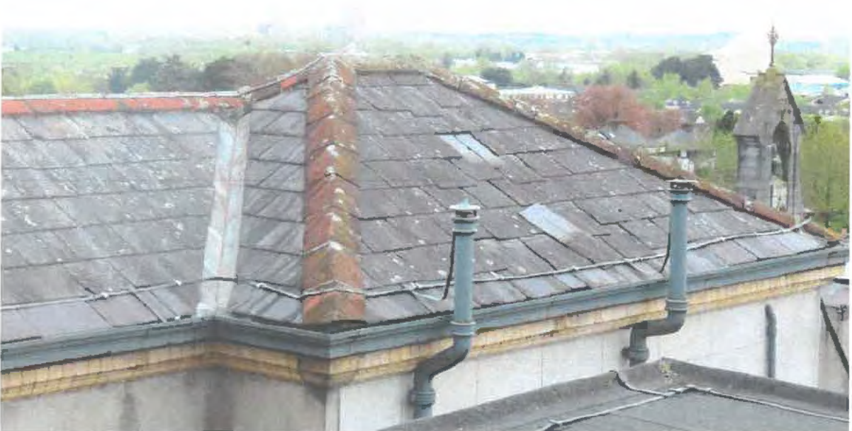
Photograph 032. Slipping slates annex building, clay ridge & hip tiles.
