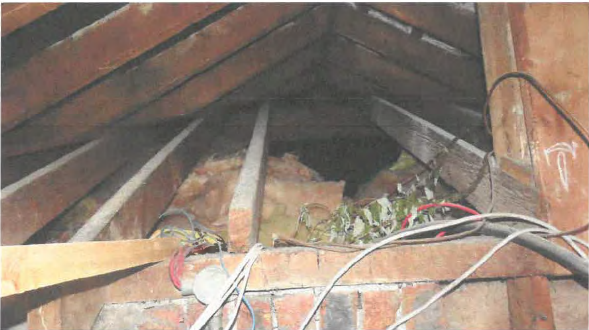
Photograph 040. North annex attic showing jack rafters for valley intersection with main pitched roof.
