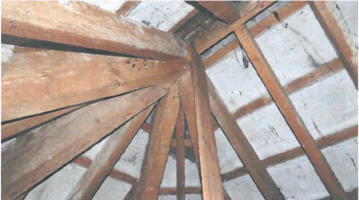
Photograph 018. Hip rafter's apex connection with jack & common timber rafters, slating battens & lime parging.
