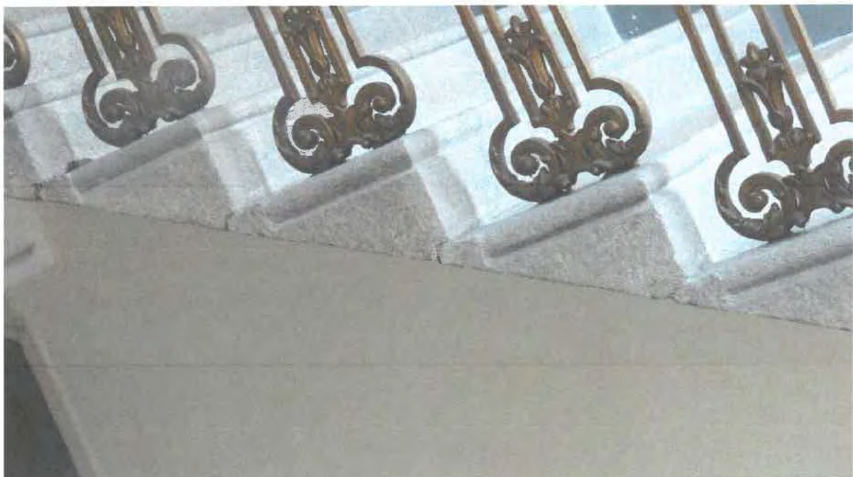
Photograph 044. Cantilever stone stairs (Review loading).
