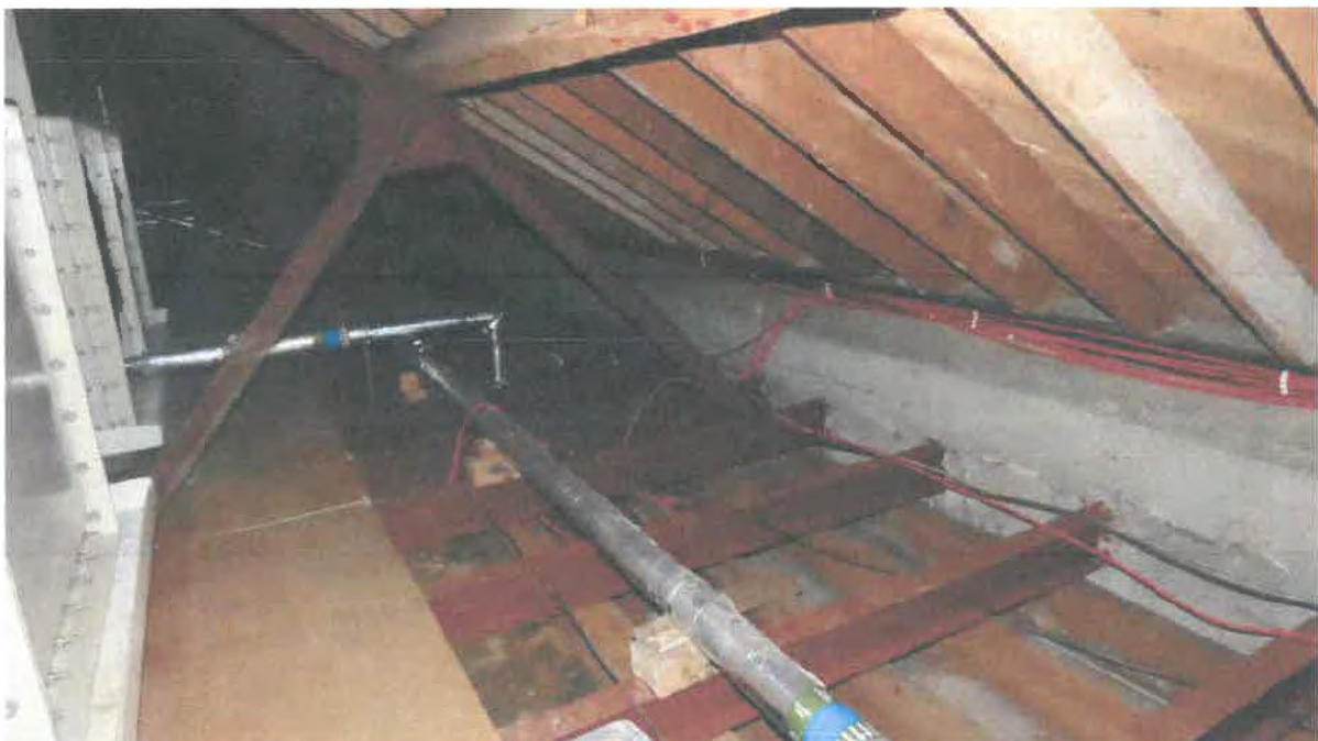
Photograph 038 North annex attic showing steel angle trusses, timber purlins, timber rafters, raised wall plate level over ceiling joist & water tank to the left.
