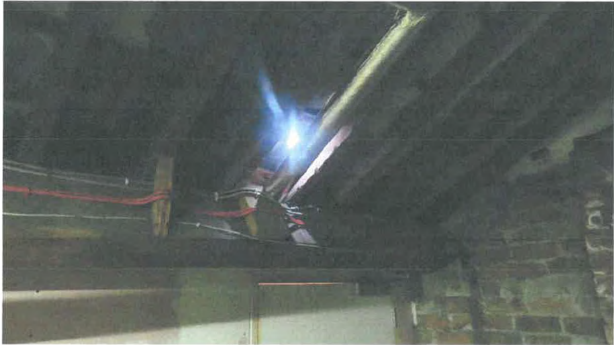
Photograph 009. Showing daylight coming through the slate plane due to slate slippage.
