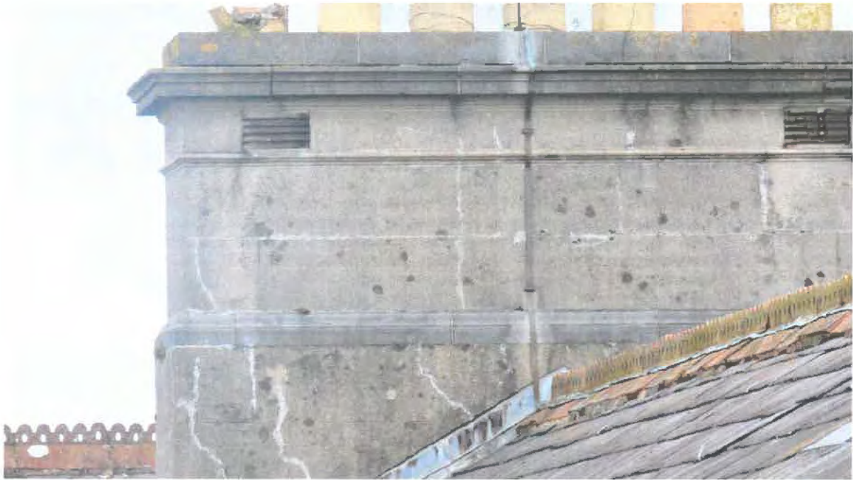
Photograph 029. Chimney cracks & damaged flue pot.
