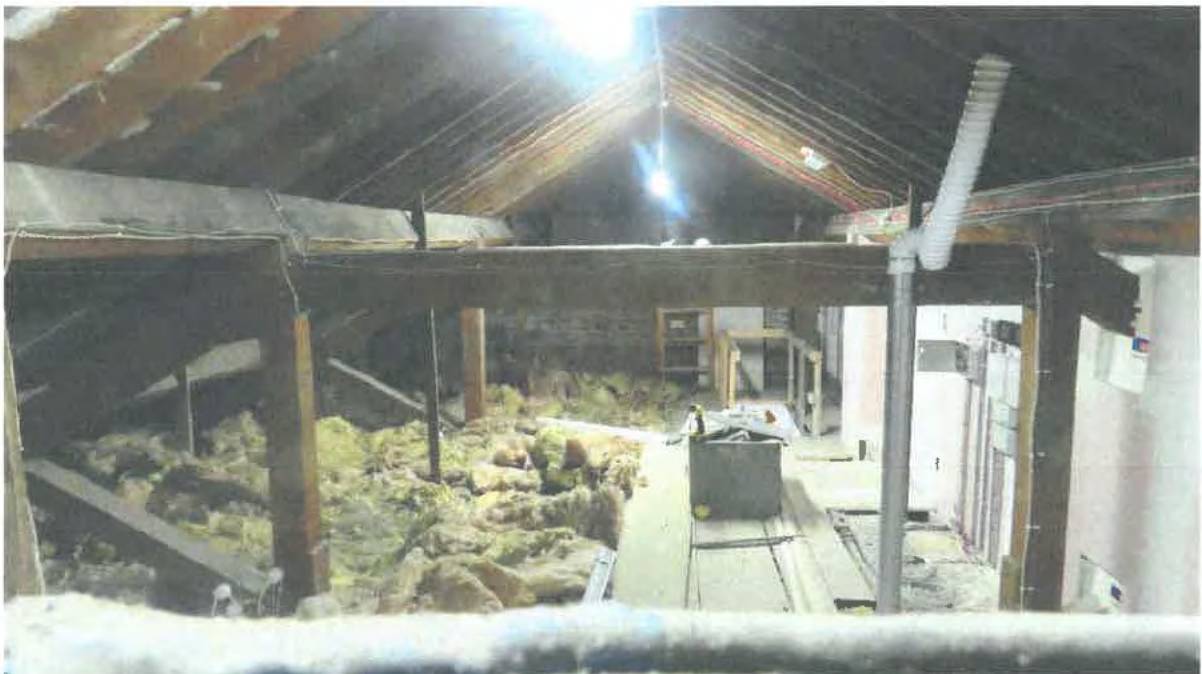
Photograph 006. Typical Timber King Post Truss with timber purlins & common timber rafters.
