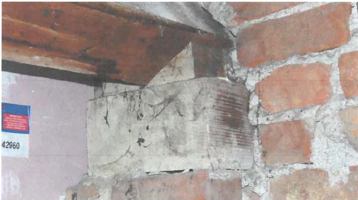
Photograph 016. Timber purlin with wedge bearing & timber block bearing pad on brick cross wall.
