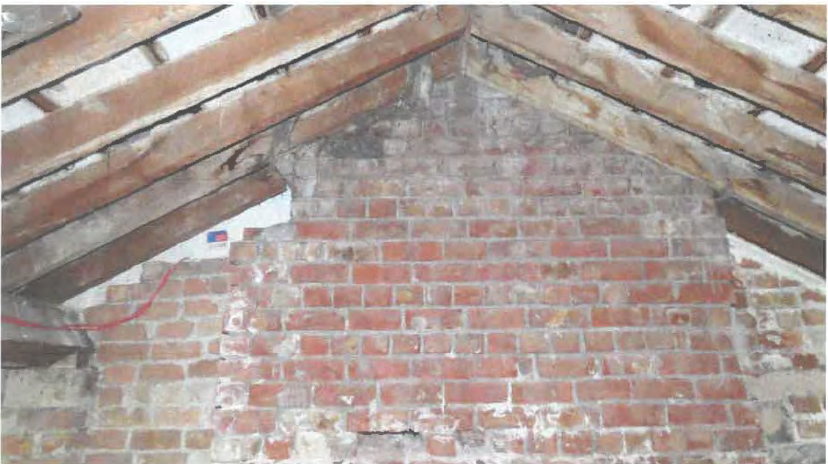
Photograph 008. Typical chimney breast constructed in brick using a form of English brick bond. No sign of dampness where the chimney penetrates the roof plane. Common timber rafters, slating battens, slate lime parging & timber purlins timber bearing pads & wedges bearing.
