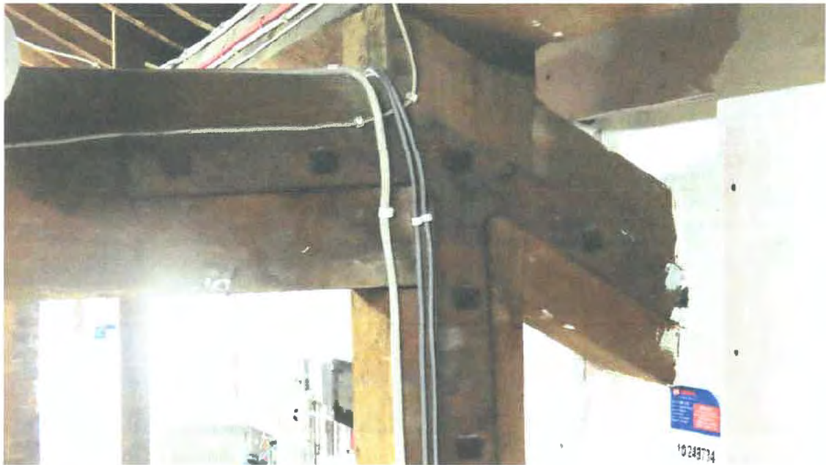
Photograph 013. Queen post with typical wrought iron joint strap.
