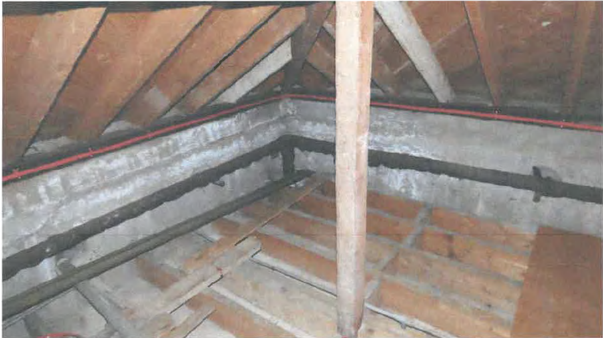
Photograph 037. North annex attic raised wall plate level over ceiling joist.
