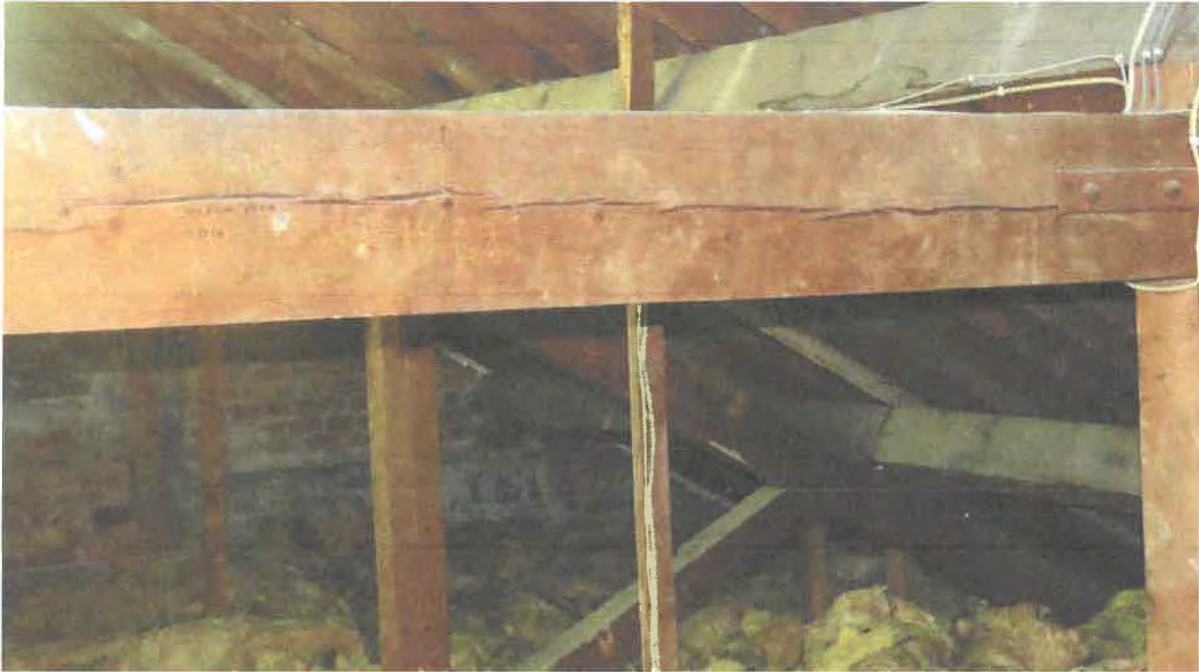
Photograph 015 Queen post collar with timber shake (not a structural problem).
