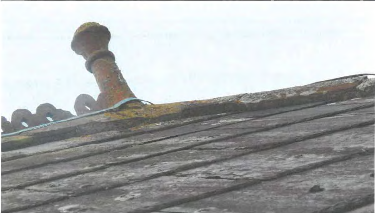
Photograph 031. Hip/ridge clay horn.
