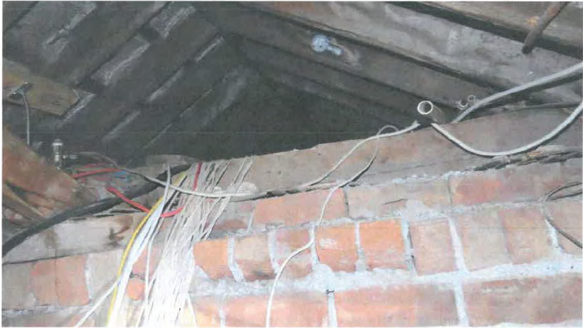
Photograph 041. South annex attic showing valley jack rafters intersection with main roof.
