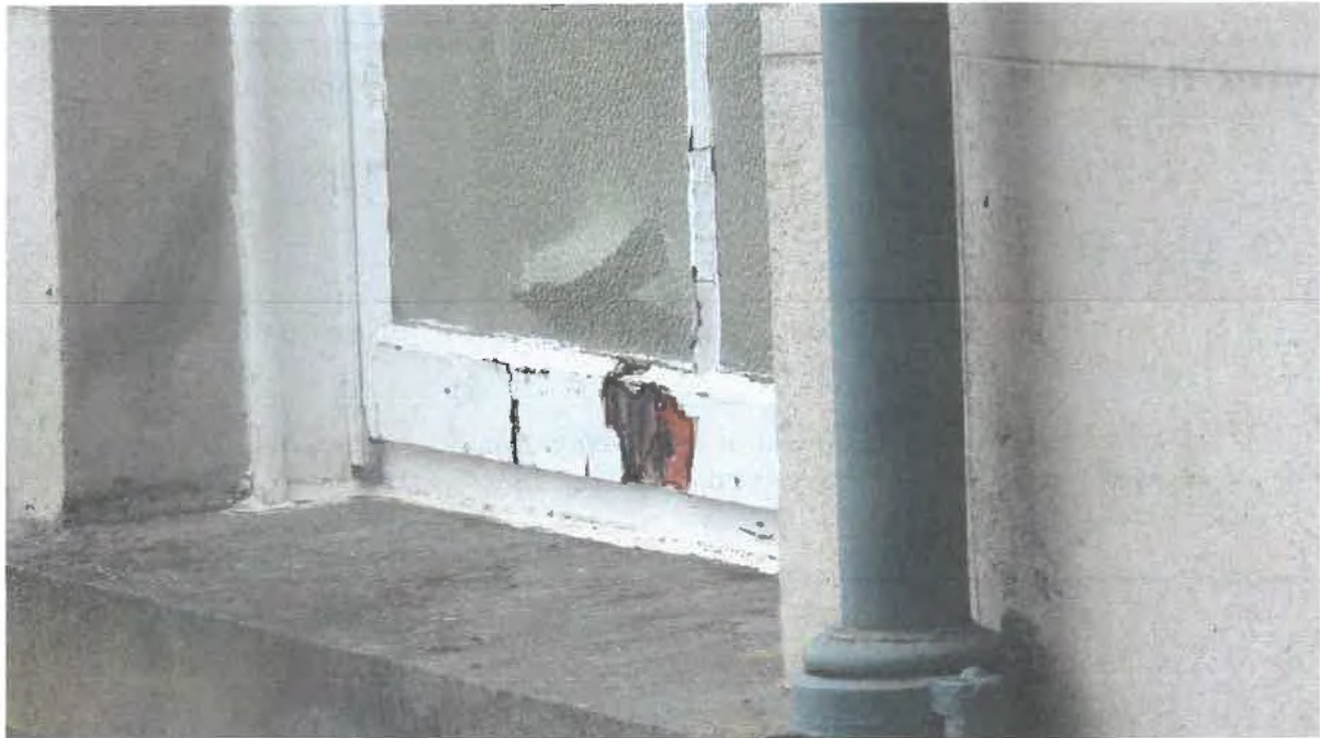
Photograph 043. Top floor annex building North end window rotting timber bottom rail.
