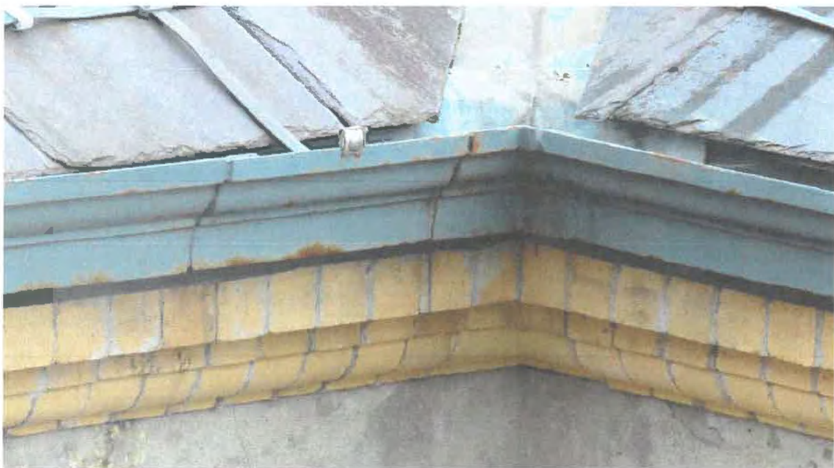
Photograph 036. Cast iron gutter with rust stain on lead bed on brick bullnosed corbel.
