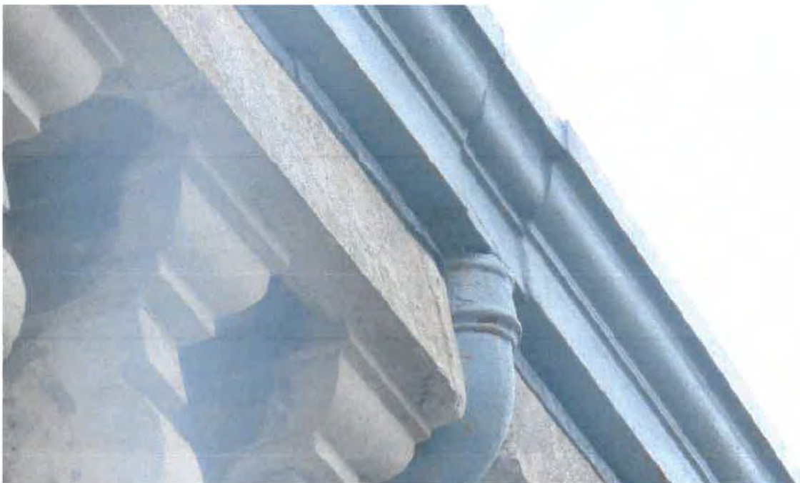
Photograph 034. Typical cast iron gutter on lead bed, on corbel masonry.
