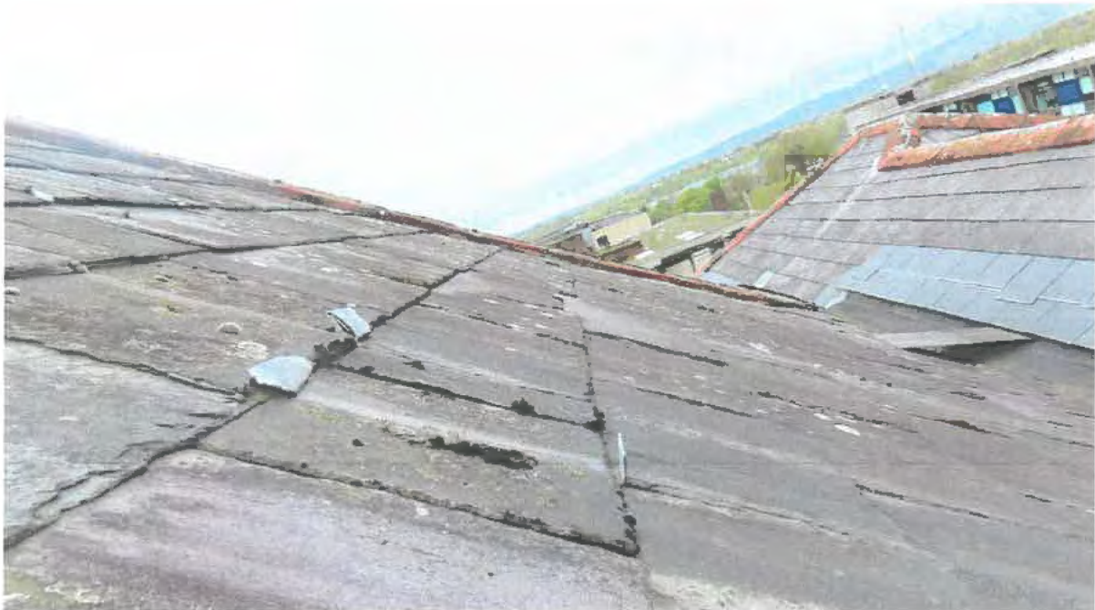
Photograph 024. Typical lead clip repairs due to slipping slates. Note clay ridge & hip tiles.
