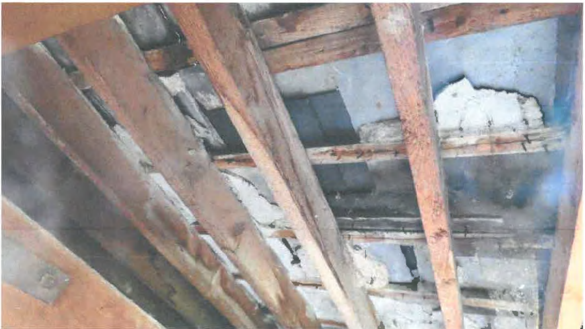
Photograph 022. Showing damaged / patched slates. In annex building.
