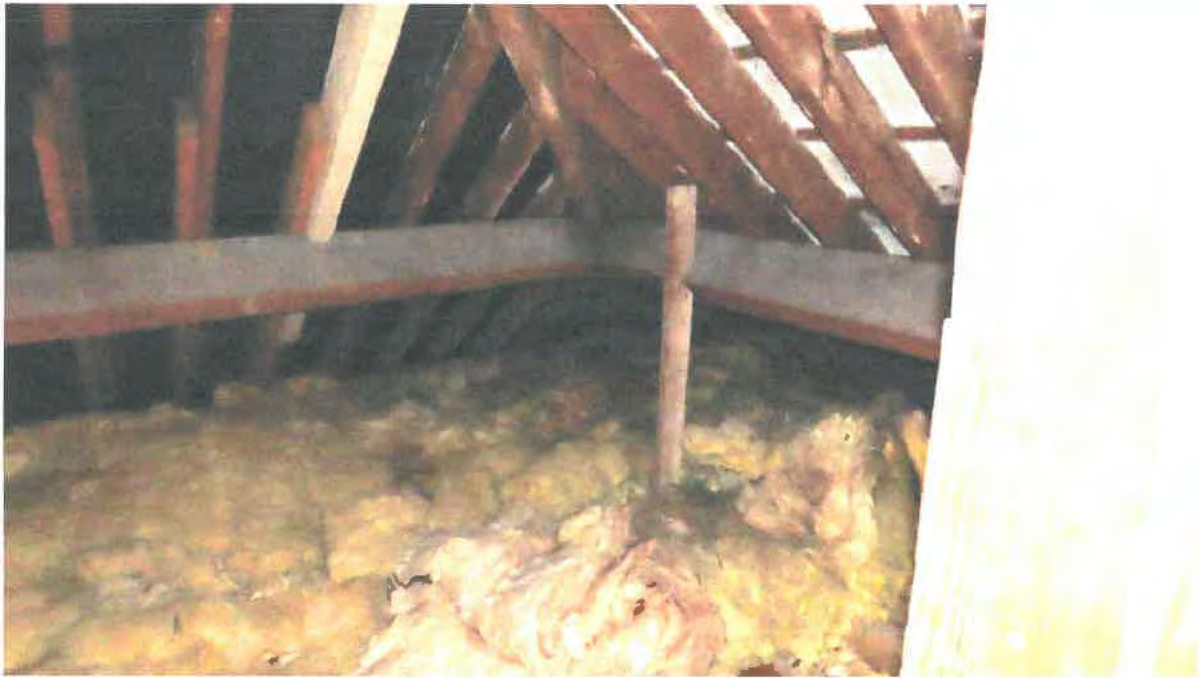
Photograph 021. Typical hip rafter with timber purlins on both sides, jack rafter & ceiling hangers.
