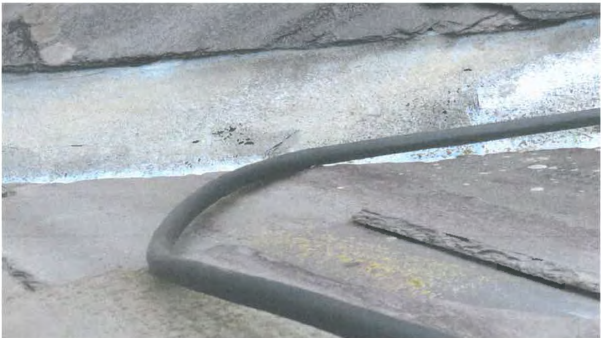
Photograph 026. Lead valley with perished lead / cracks.
