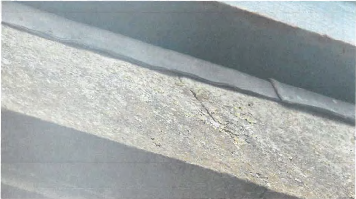
Photograph 035. Typical cast iron gutter on lead bed.
