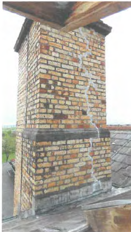
Photograph 027. Chimney cracks.
