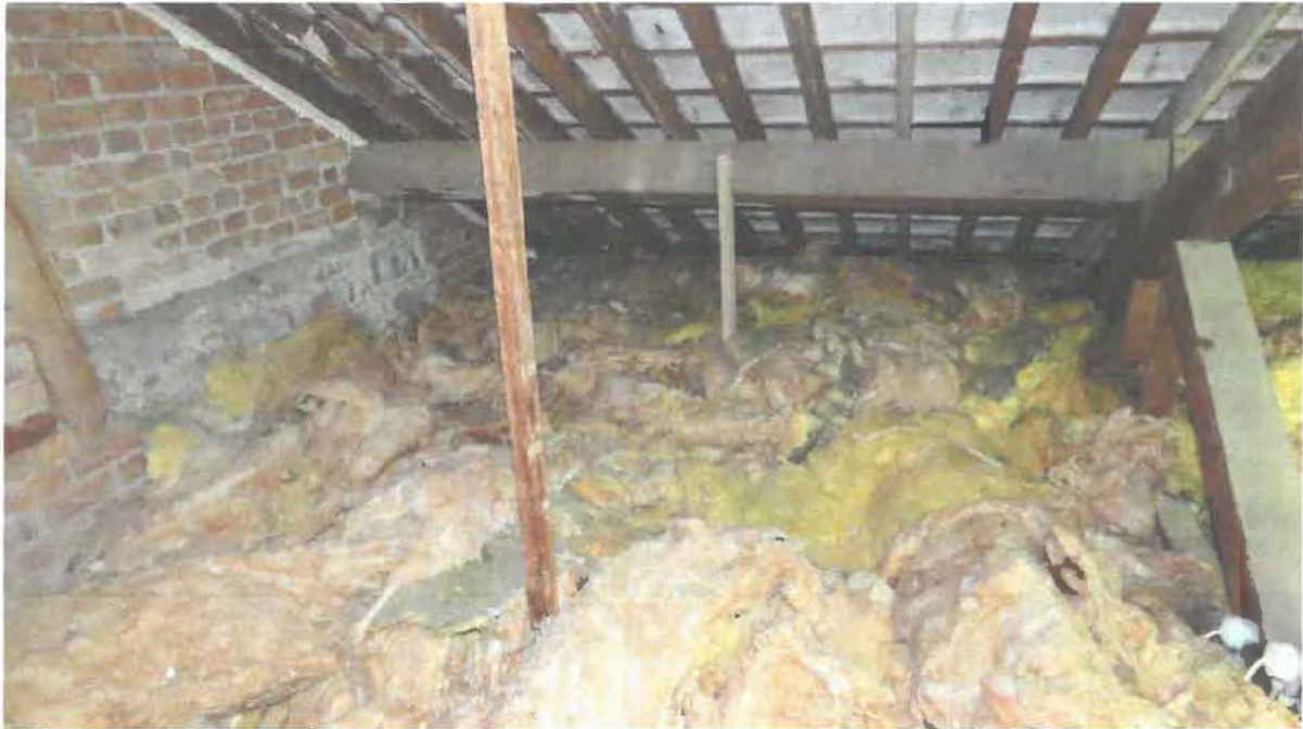
Photograph 007. Typical timber purlins bearing into cross walls, common timber rafters, slating battens, lime parging (torching) to the underside of the natural stone slates & ceiling joist hangers.
