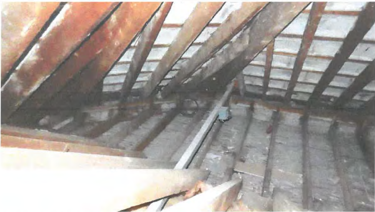
Photograph 019. Wall plate, jack rafters & ceilings joist at the hip octagon end of the roof.
