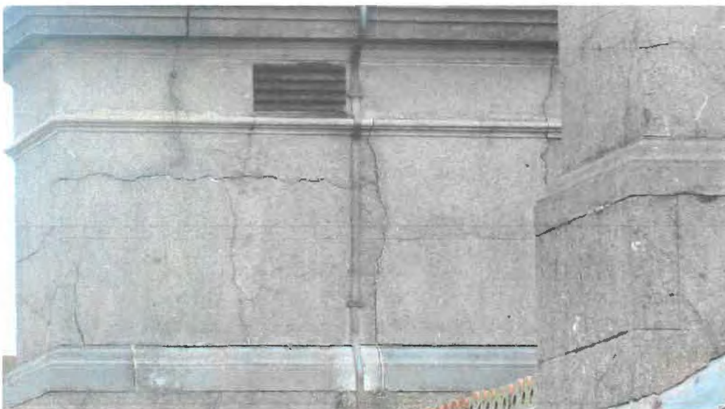
Photograph 028. Chimney cracks.
