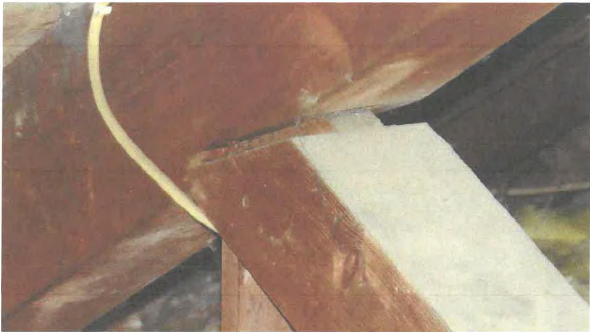
Photograph 011. Open struct joint in the Queen post truss due to shrinkage / truss bottom boom deflection.
