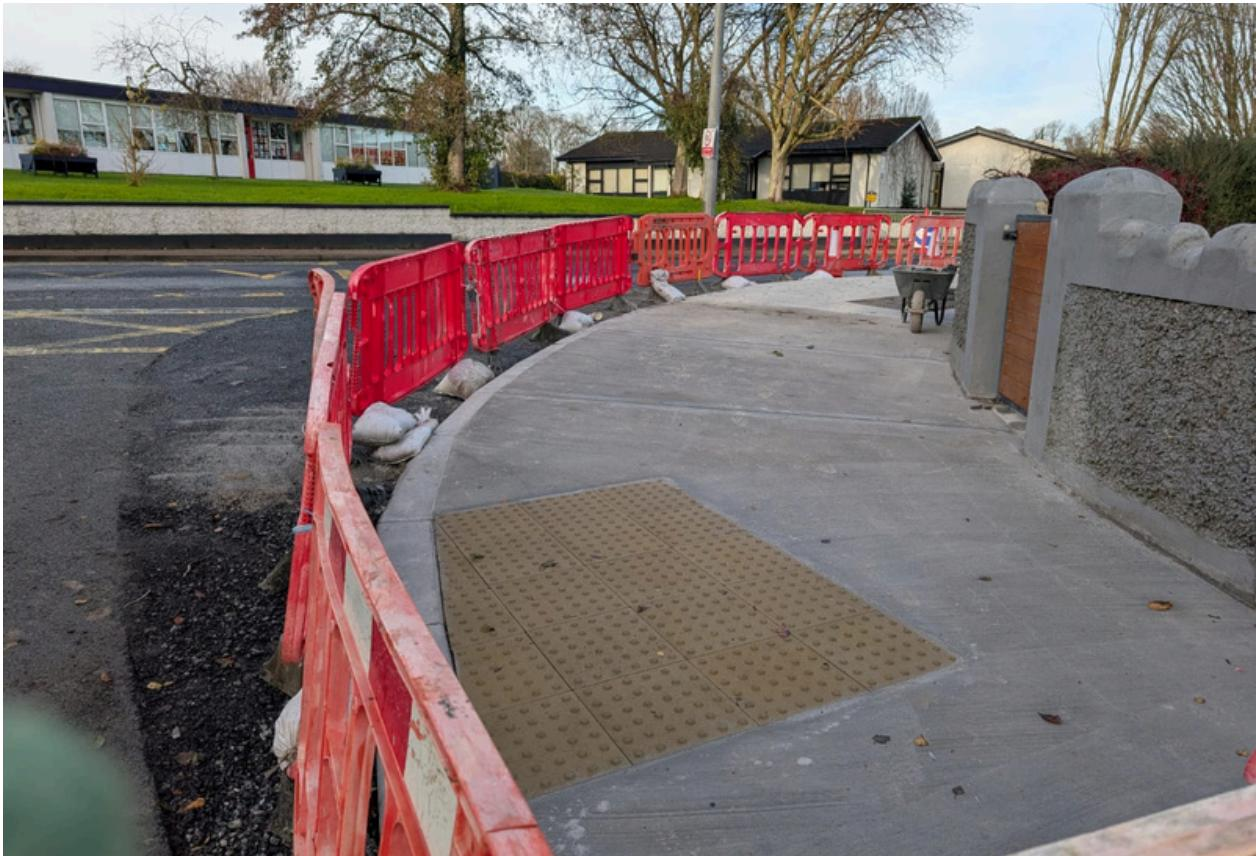
The work continues with the excavation of footpaths at the junction of Lanahrone Avenue and Corbally Road. New kerbs are in place at different sections and fresh concrete is being poured.
