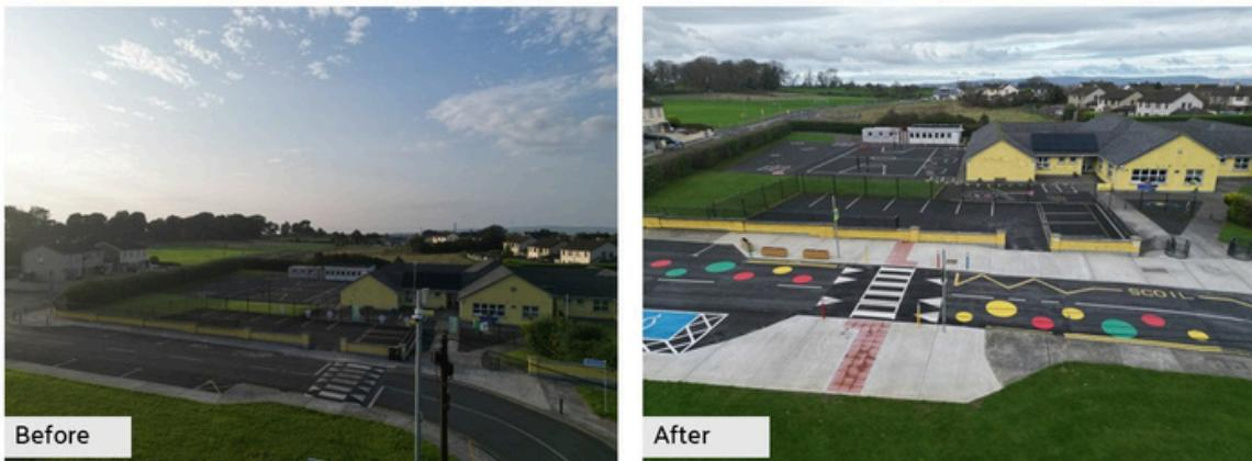
The safety improvements around Patrickswell NS are now completed. The works involved installing a raised pedestrian crossing at Lisheen Park to improve safety for schoolchildren. Additional works included traffic-calming build-outs and footpath widening to enhance visibility and create safer walking routes. A new bus bay was also constructed to relocate school bus parking away from the main entrance, reducing congestion and improving overall road safety.
