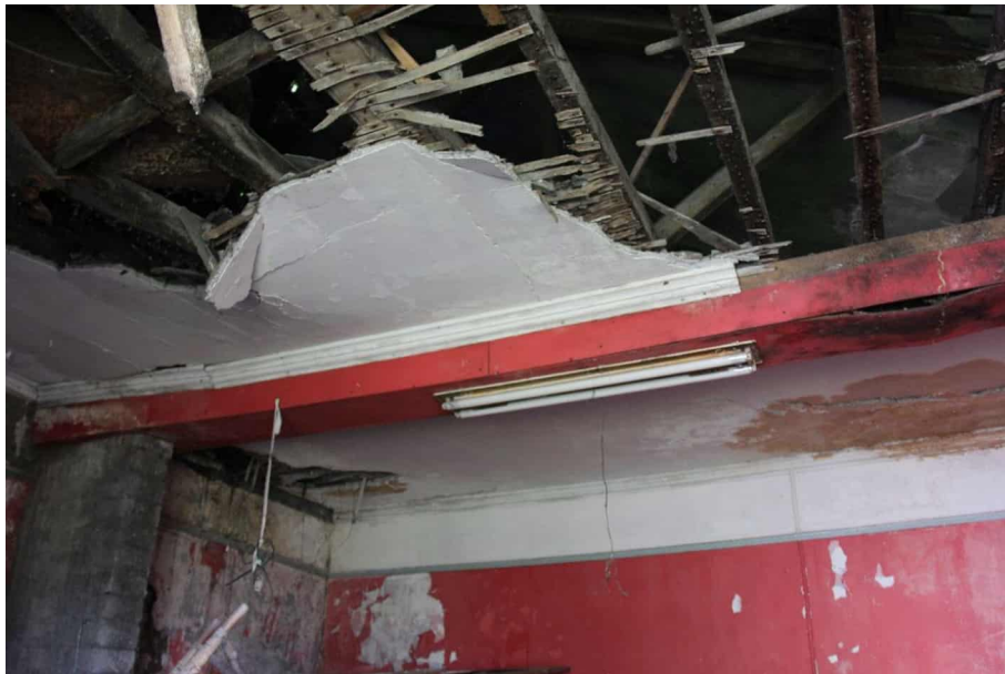
Photograph 6 View of the failed ceiling of the end room. Note laths and sections of coving.
