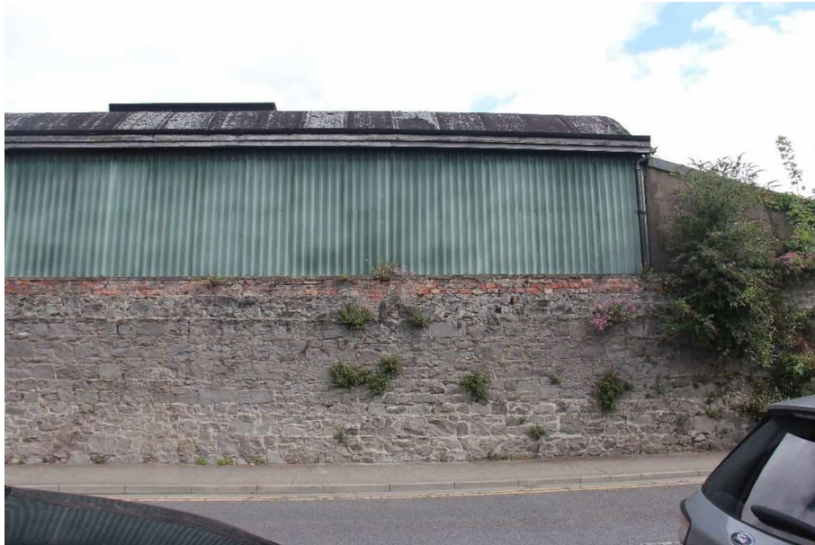
Photograph 4 Example of the external wall cladding to the southern elevation.
