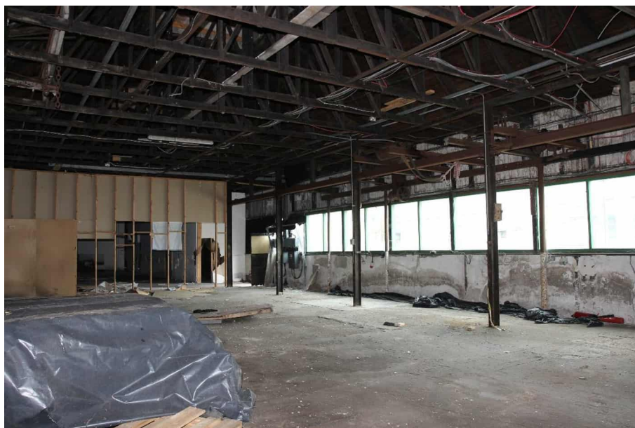
Photograph 11 View, facing westwards. Note concrete infill to the lower section of the northern wall.
