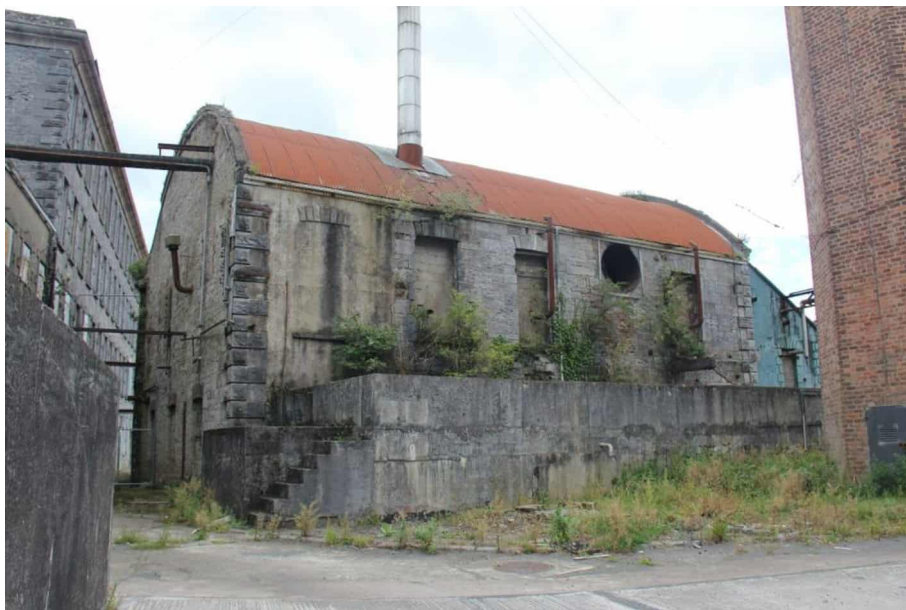
Photograph 2 External view of the Engine House. Note curved corrugated sheeting and chimney stack protruding from the roof.
