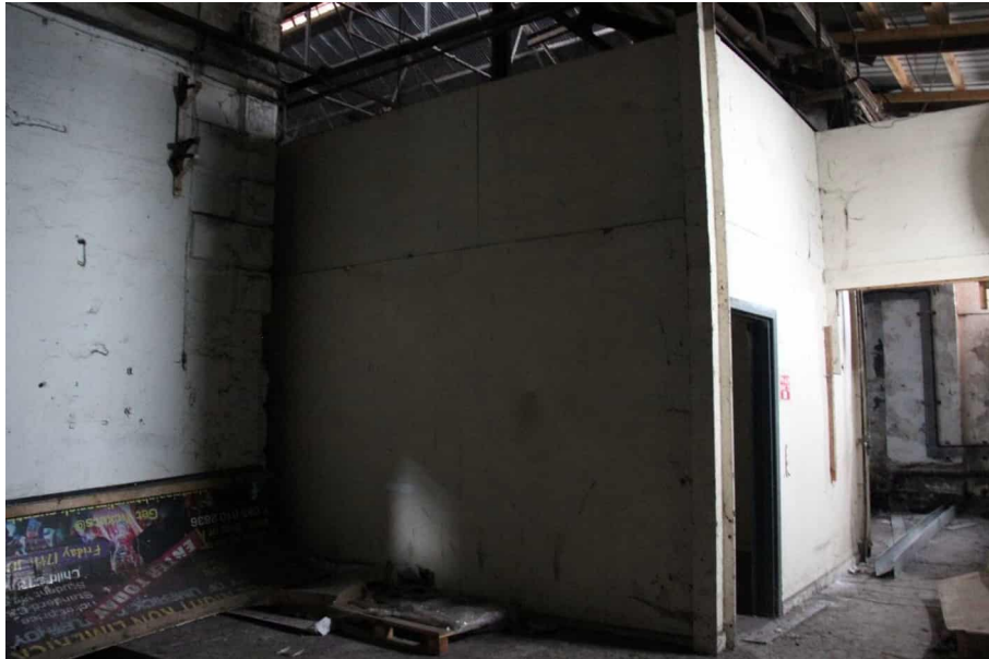
Photograph 21 Exterior of timber stud partitioned room.
