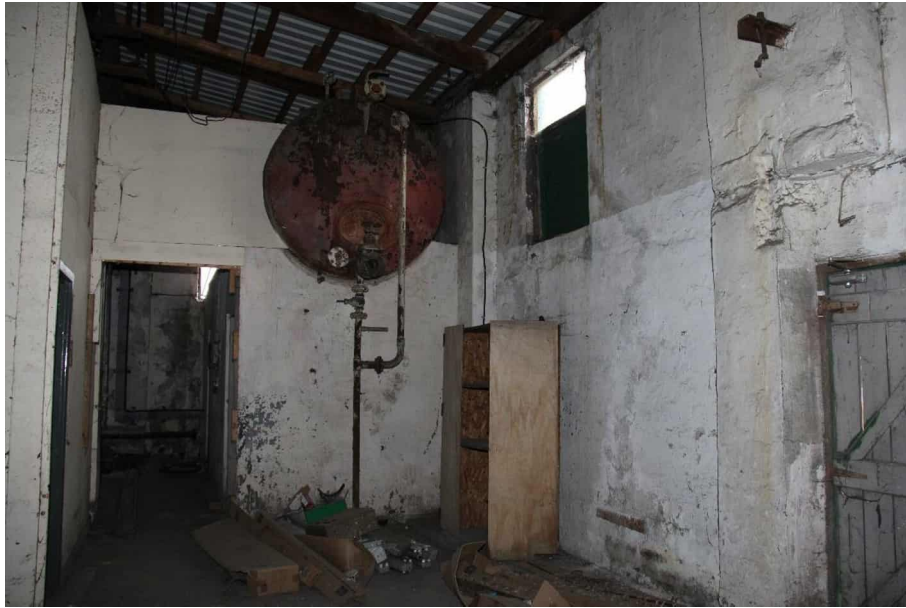
Photograph 20 Masonry support for a fuel tank, with timber partitions to the LHS.
