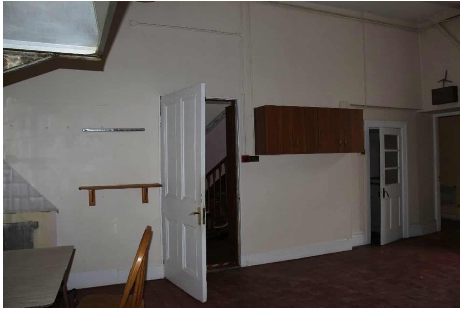
Photograph 27 - Modern hollow 4 panel door with brass-effect lever handle.
