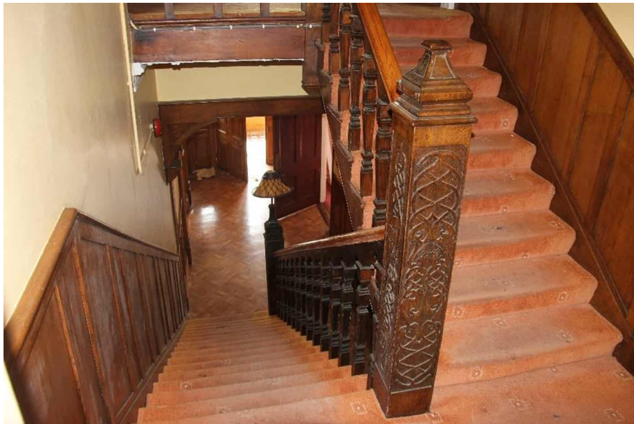
Photograph 44 - Decorative newels and timber wainscoting to Return level or main staircase.
