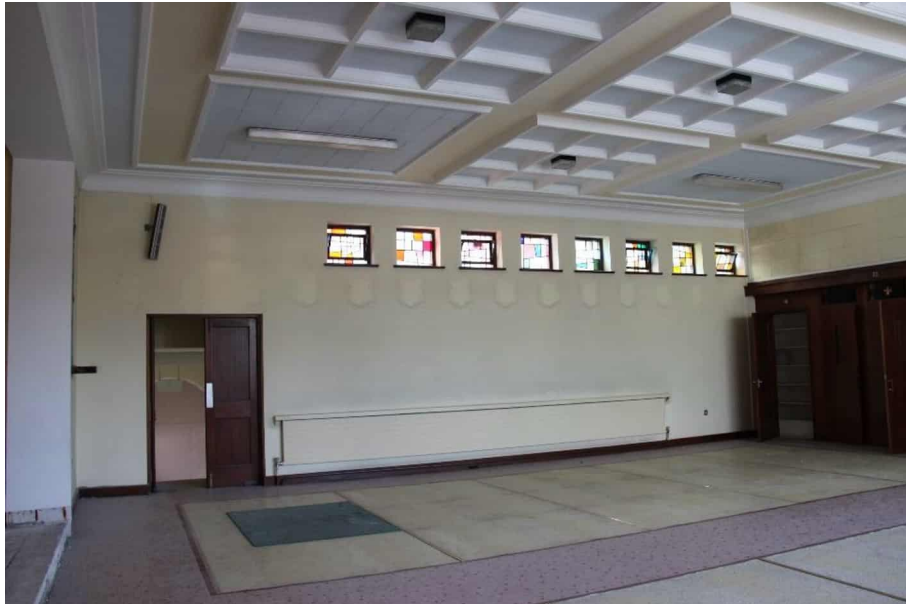
Photograph 40 - Modern ceiling with acoustic liners in Chapel (Return).
