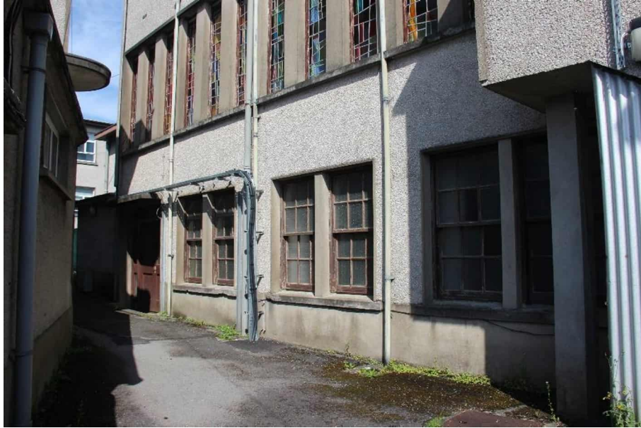
Photograph 13 - Modern timber sliding sash with obscured glazing.
