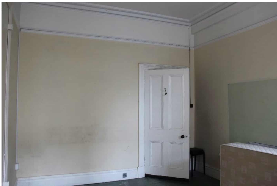
Photograph 42 - 4 panel solid timber door with timber knob in earlier building.
