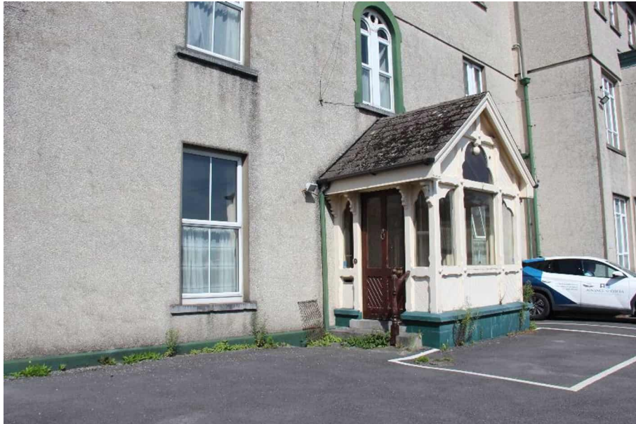
Photograph 4 - 'A' pitch with cementitious slates.
