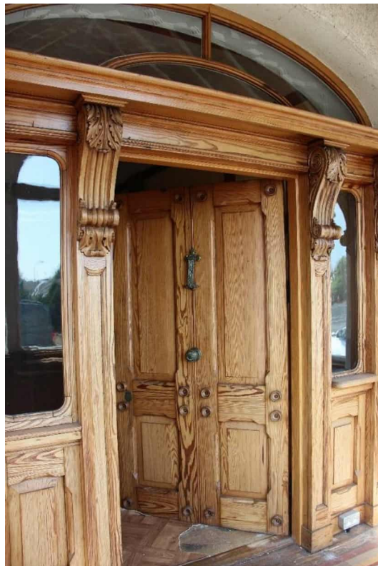
Photograph 24 - with stylised oak corbels and scrolls, timber header and cornice with brass ironmongery
