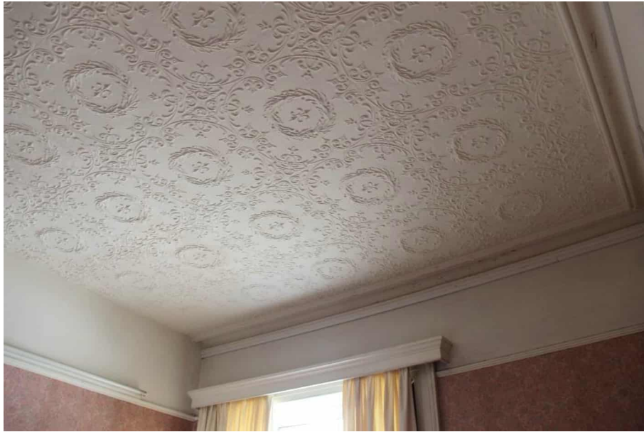
Photograph 39 - Modern decorative ceiling tiles affixed directly (not suspended).
