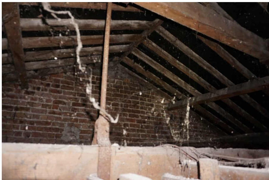
Photograph 26 - Roof Space indicating cast iron hanger.
