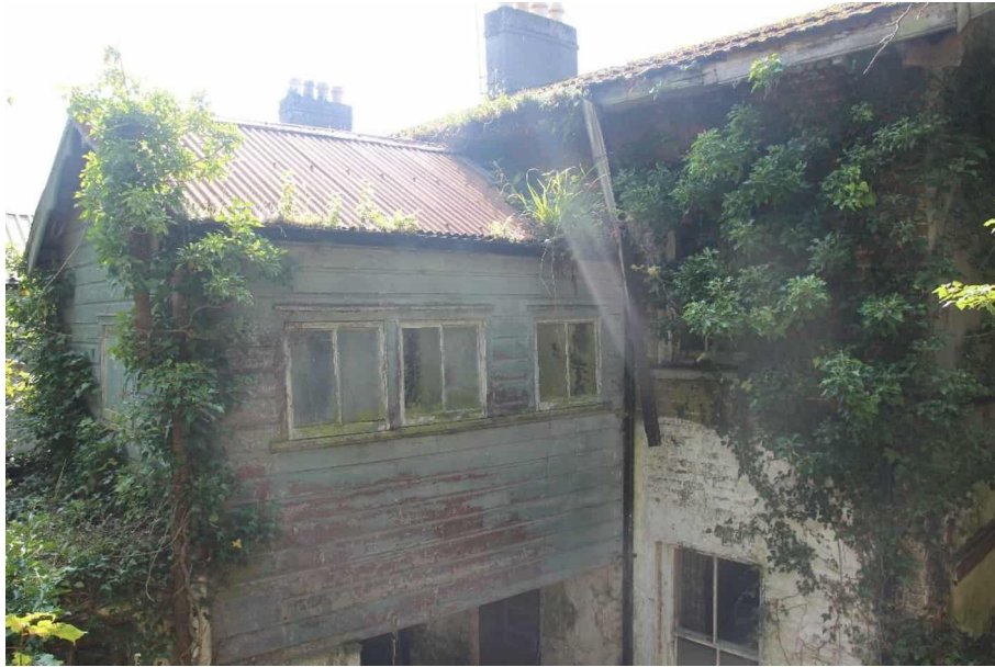
Photograph 5 - Timber clad Return Annex with corrugated iron roof and painted brick to main building.
