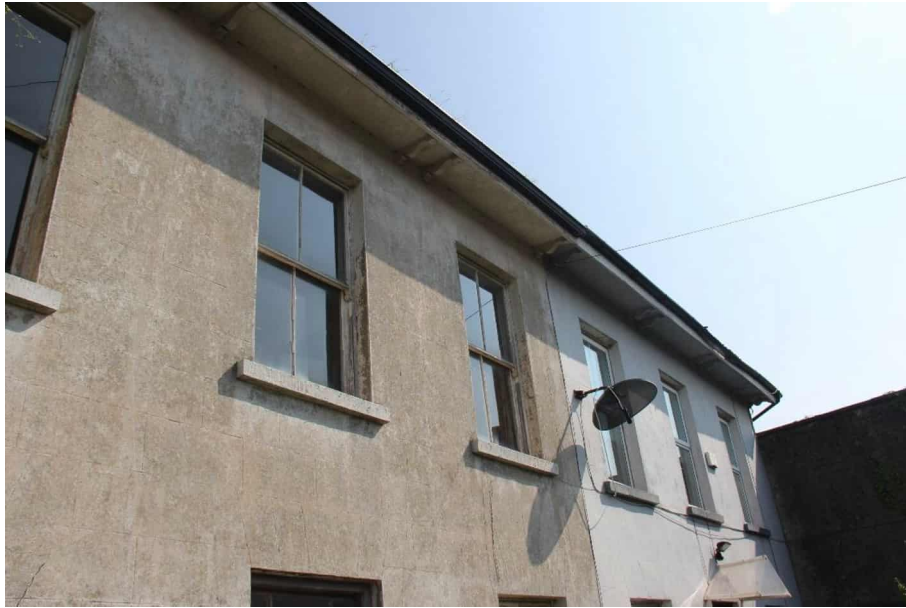
Photograph 3 - Cementitious render ruled and lined.
