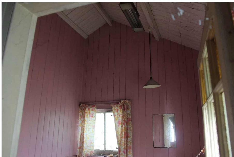
Photograph 22 - Timber boarding to Return Annex walls.
