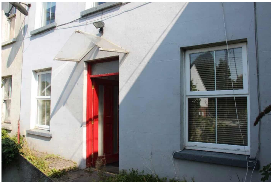
Photograph 29 - Front facade lower, cementitious render ruled and lined and painted.
