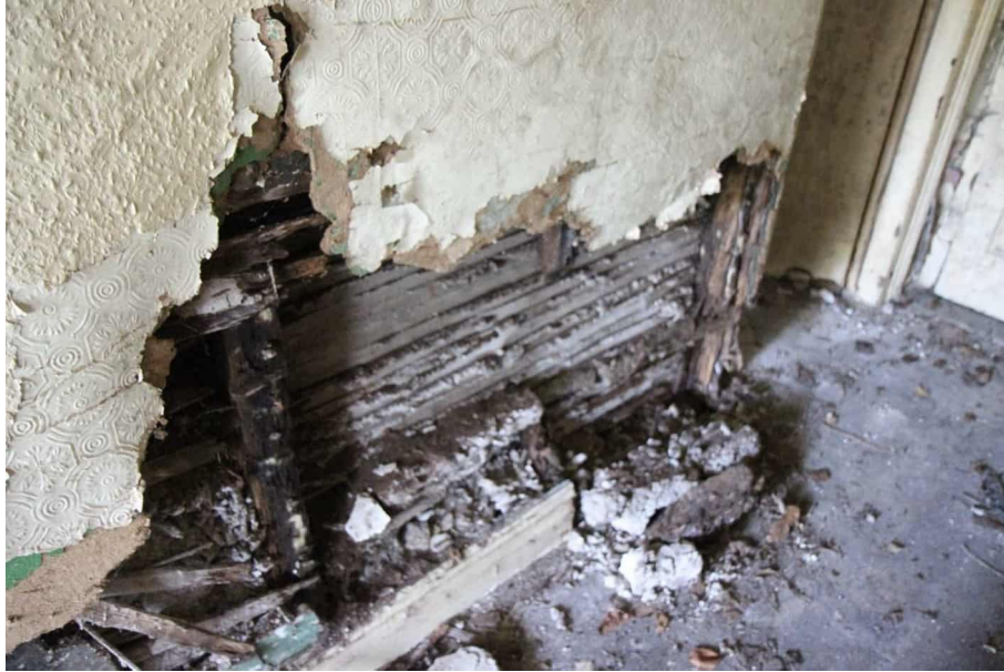
Photograph 11 - Lath-and-plastered stud wall to hall corridor.
