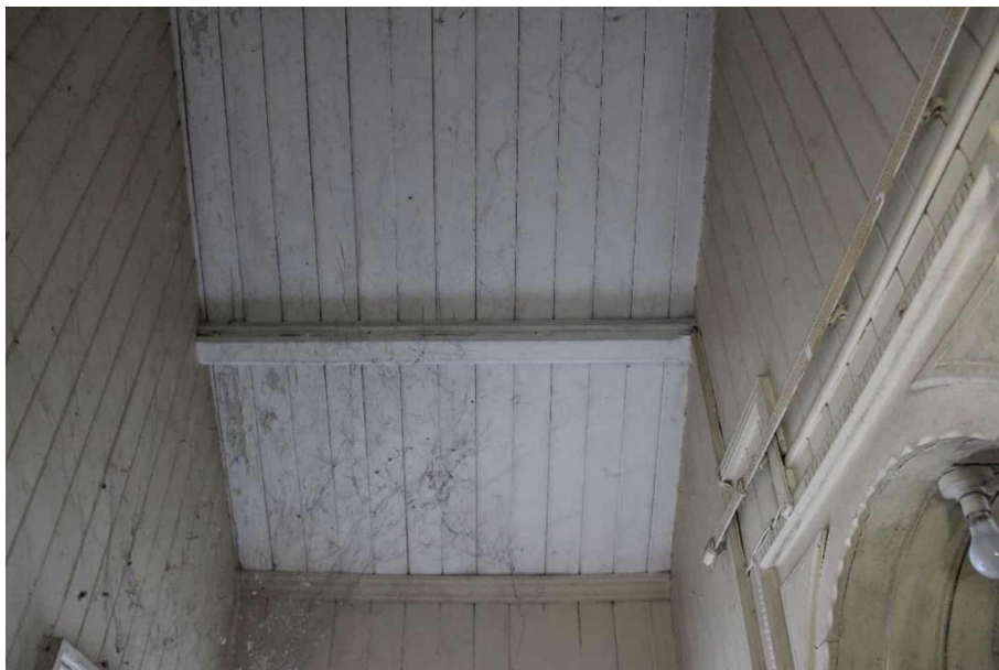
Photograph 20 - timber boarded ceiling to Return Annex.
