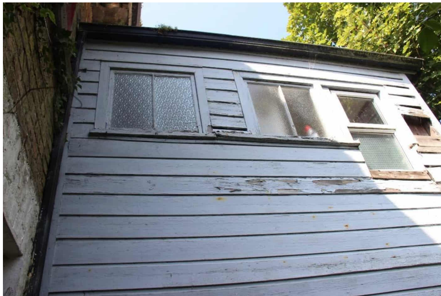
Photograph 31 - Return Annex timber cladded walls of site facade.
