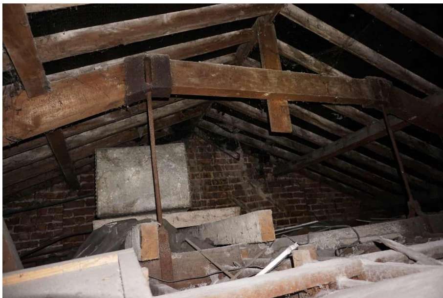
Photograph 48 - Truss with cast iron hanger.
