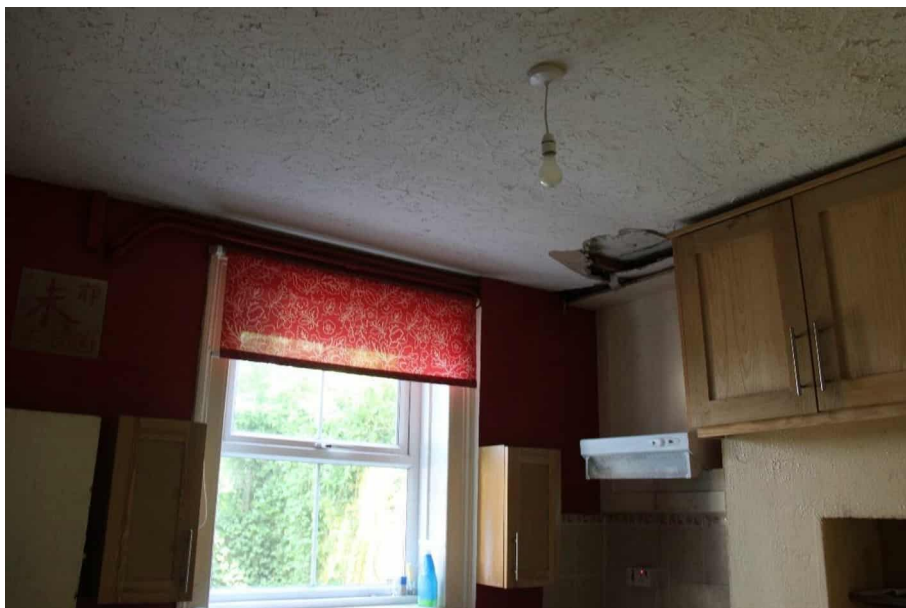
Photograph 35 - Stippled ceiling in Kitchen - possible Artex.
