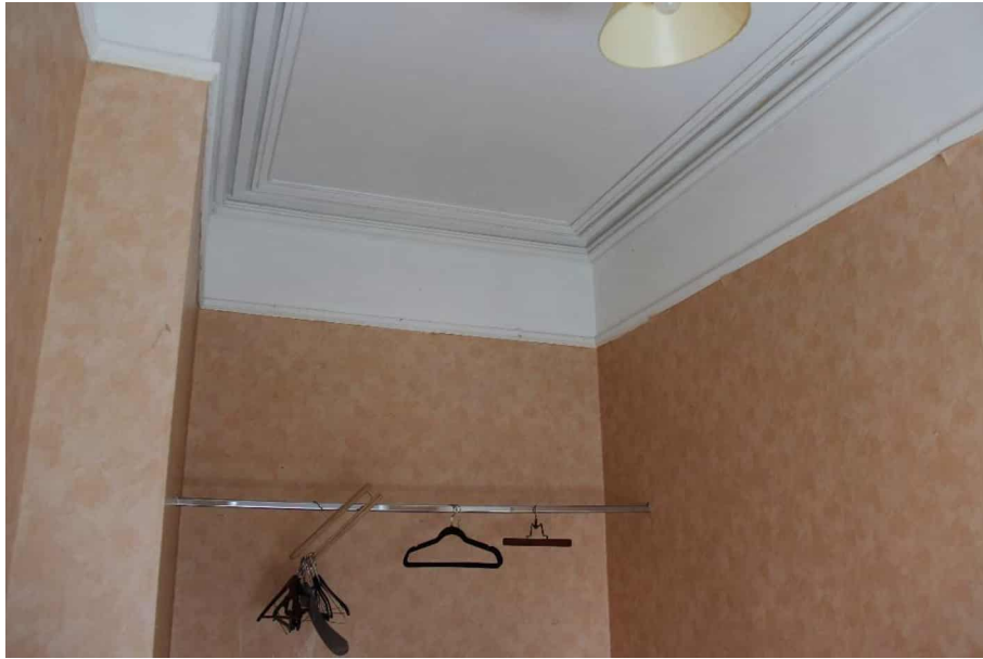
Photograph 44 - smooth plastered ceilings with coving.
