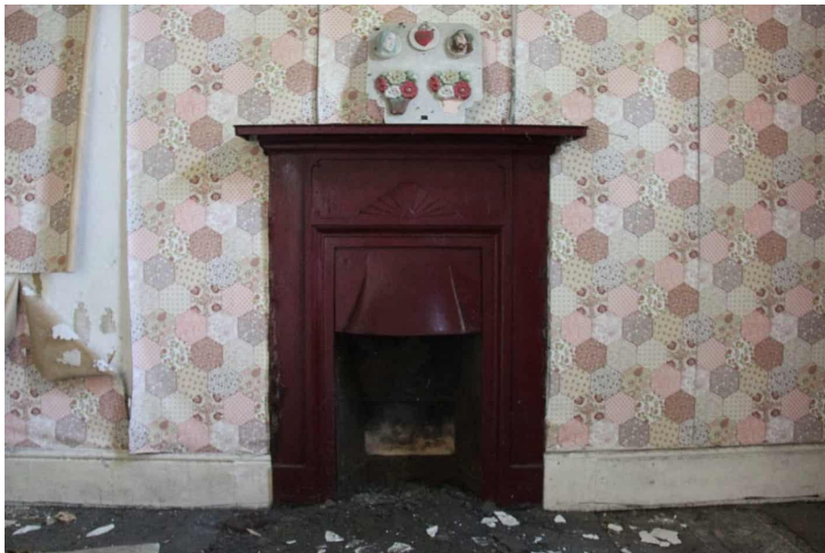
Photograph 24 - Original cast iron fireplace to rear bedroom.
