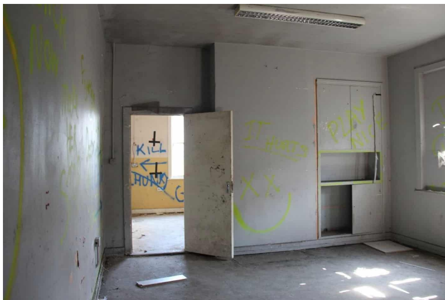
Photograph 6 General internal view of the “welfare” building, with a modern plaster slab ceiling, and modern plaster slabbed drylined internal walls.
