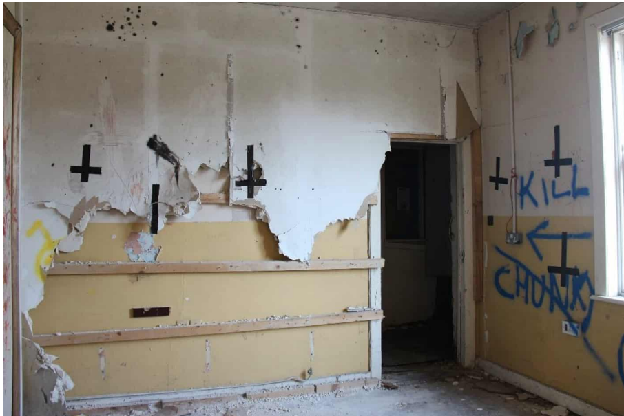
Photograph 8 View of the damaged internal lining within the “welfare” building.
