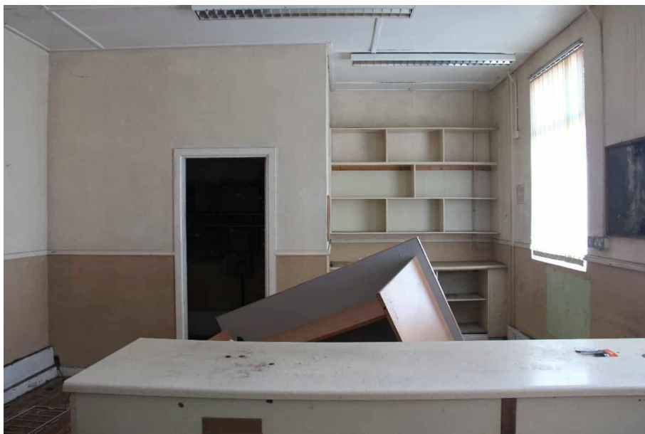
Photograph 10 Front office, with modern plasterboard applied to the walls.
