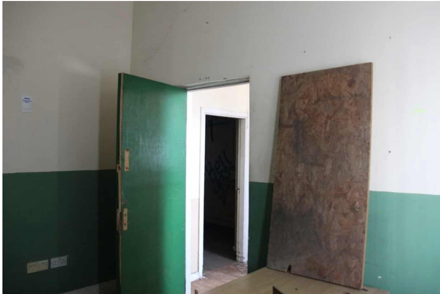
Photograph 12 Example of a hollow core door leaf, found mostly to the western section of the main building.
