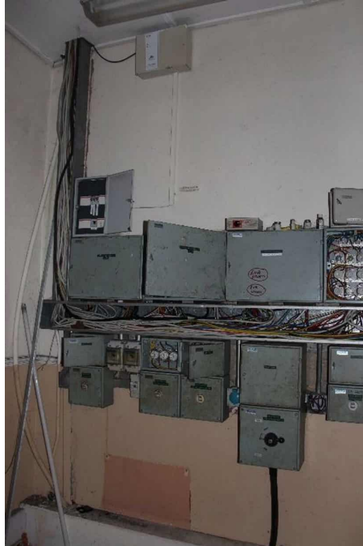
Photograph 16 Surviving fuse boxes, meters, alarm systems etc.
