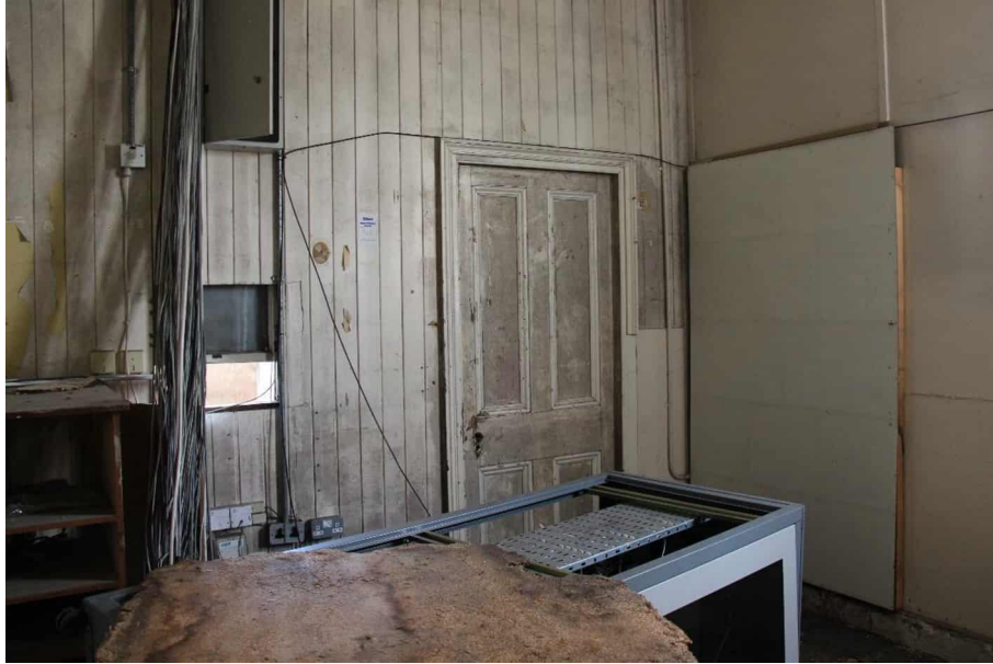
Photograph 9 Example of the variance of internal wall finishes, with T&G Panelling visible and more recent “beauty board” panelling.
