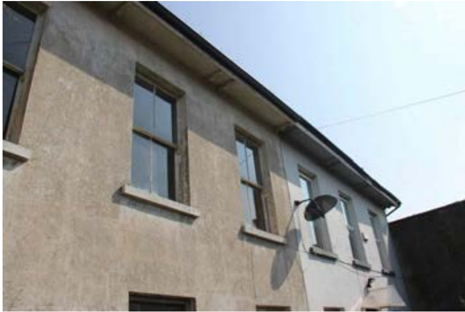
Photograph 3 - Cementitious render ruled and lined.
