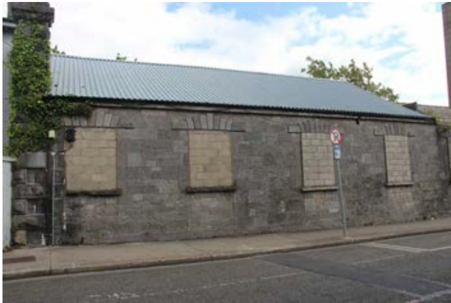
Photograph 2 North Circular Road elevation of the end section of the Cheese Plant. Note pressed metal sheeted roofing.
