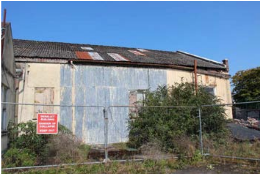
Photograph 4 View of the southern elevation, showing the corrugated sheeted panels.
