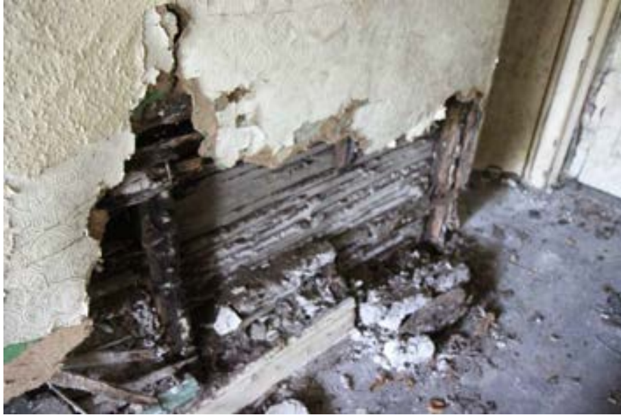
Photograph 11 - Lath-and-plastered stud wall to hall corridor.
