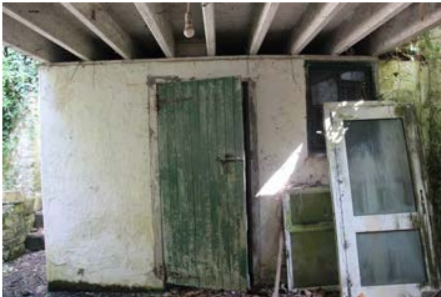
Photograph 18 - Outbuilding front facade with exposed joists to underside of Return Annex.
