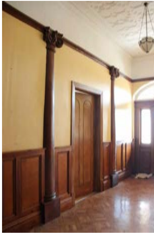
Photograph 25 - a 2-panel solid timber door opposes a 4-panel solid timber door in the main hall.
