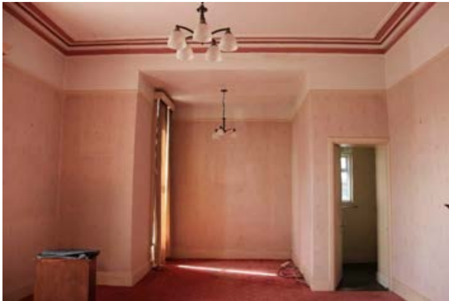
Photograph 19 - Original gable wall broken through to provide for modern extension.
