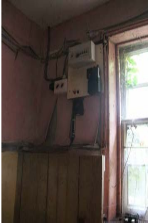
Photograph 17 - Modern fuse box located in home office.
