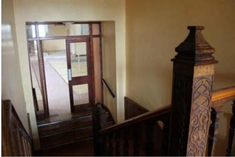
Photograph 43 - Modern timber and glazing doors with vestibule screen to chapel.
