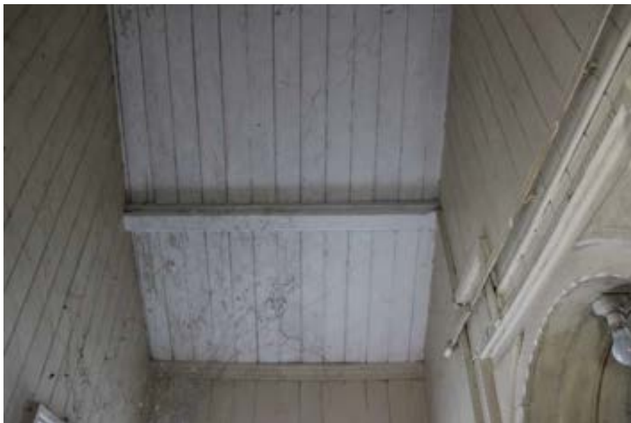
Photograph 20 - timber boarded ceiling to Return Annex.
