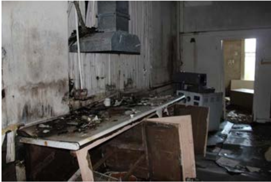
Photograph 15 Laboratory with an example of the timber sprung floors, all decimated with rot now.
