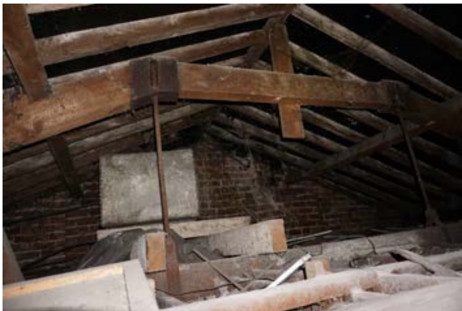
Photograph 48 - Truss with cast iron hanger.
