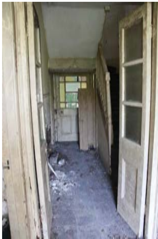
Photograph 15 - Double leaf door used to separate front of house from rear.
