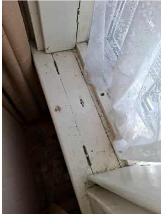
Photograph 33 - Hidden shutter in the bay window in room off 1st room RHS.
