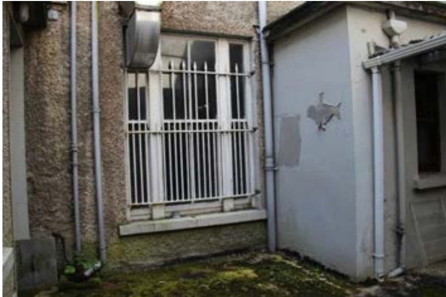
Photograph 8 - Original Wyatt timber window at kitchen.
