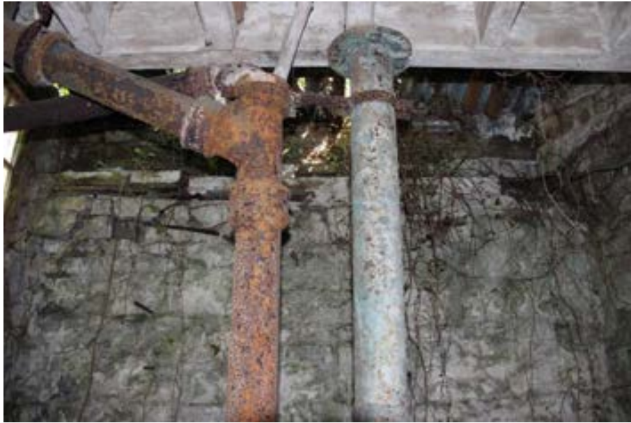
Photograph 19 - Cast iron support system for Return Annex floor.
