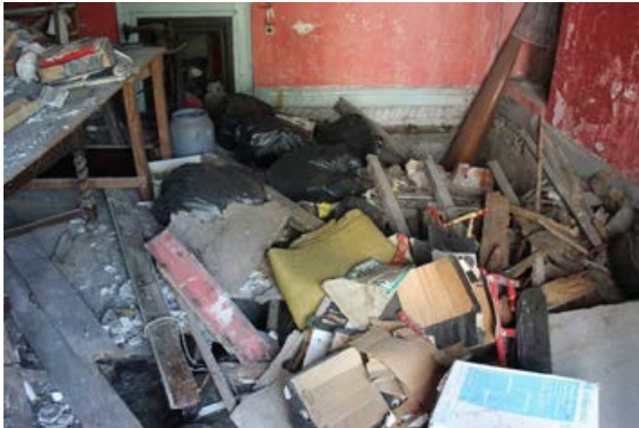
Photograph 9 View of the floor of the end room. Sprung timber floor. Failed.
