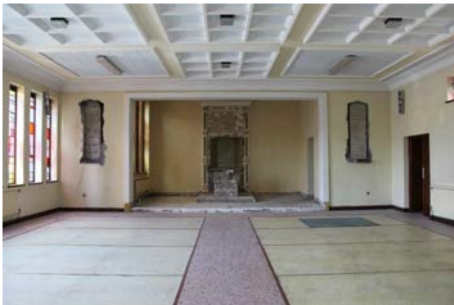
Photograph 50 - modern chapel floor with mosaic and linoleum floor covering. Alter removed.
