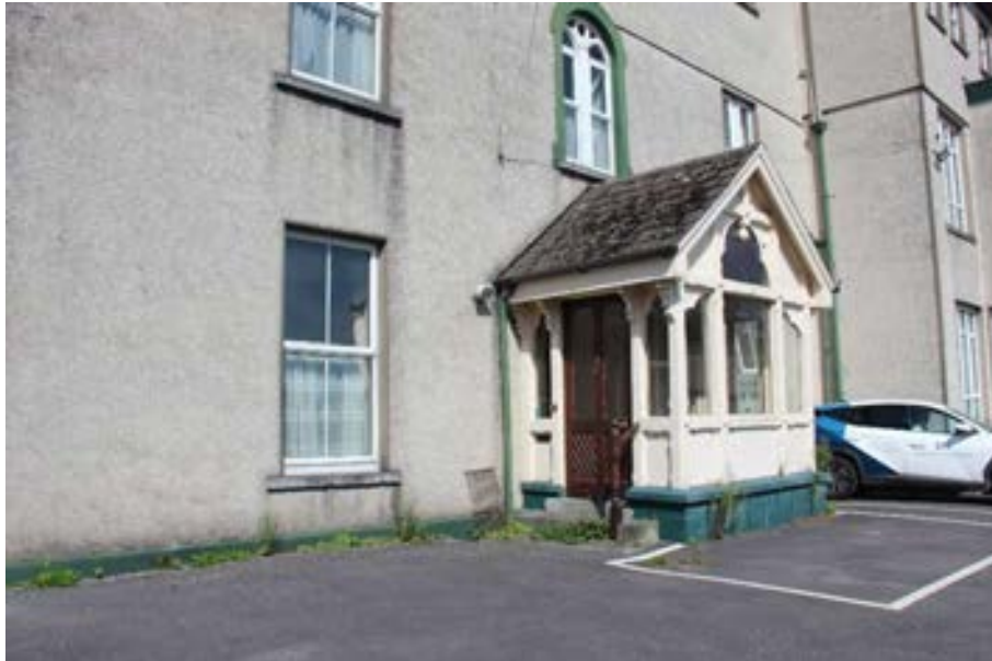
Photograph 4 - 'A' pitch with cementitious slates.
