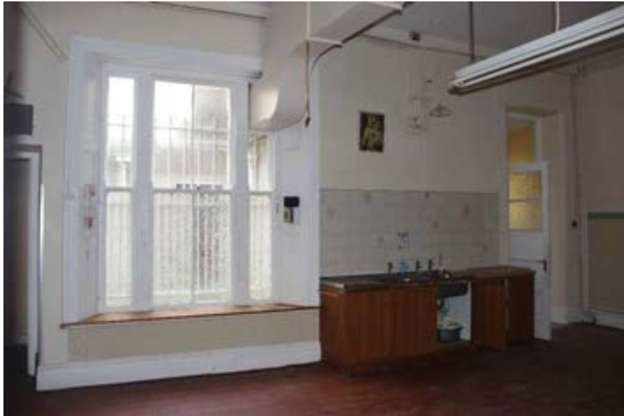
Photograph 31 - Shutter boxes extant in the Kitchen. Also, units with sink remain.
