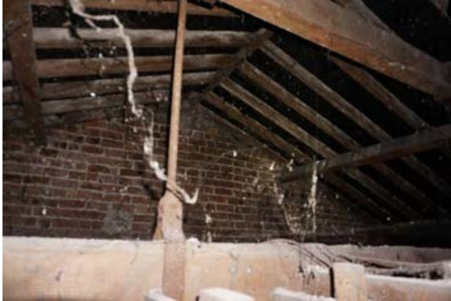
Photograph 26 - Roof Space indicating cast iron hanger.
