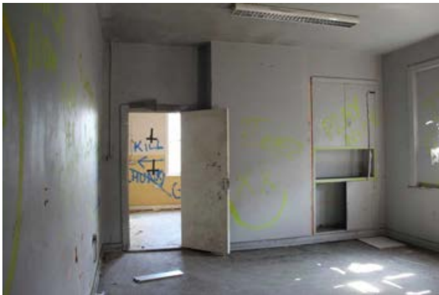
Photograph 6 General internal view of the “welfare” building, with a modern plaster slab ceiling, and modern plaster slatted drylined internal walls.
