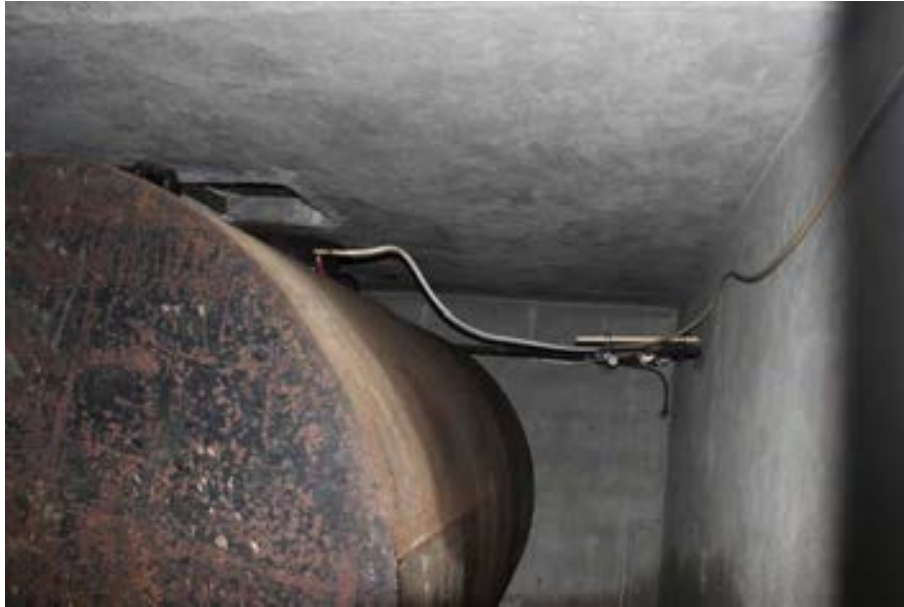
Photograph 36 - Small basement rooms house the oil tanks and burner. Electrical distribution boards may also be located here.
