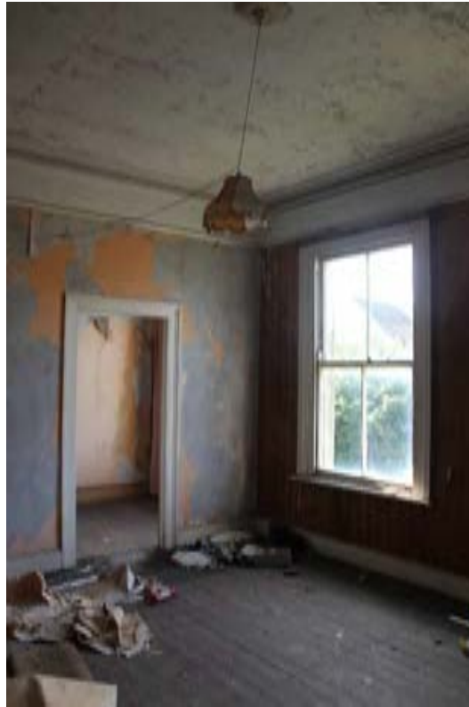
Photograph 21 - Lath-and-plaster ceilings to front room.
