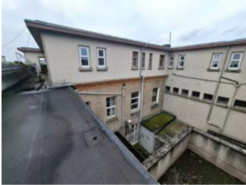
Photograph 5 - Earlier render remains on the original building at rear elevation.
