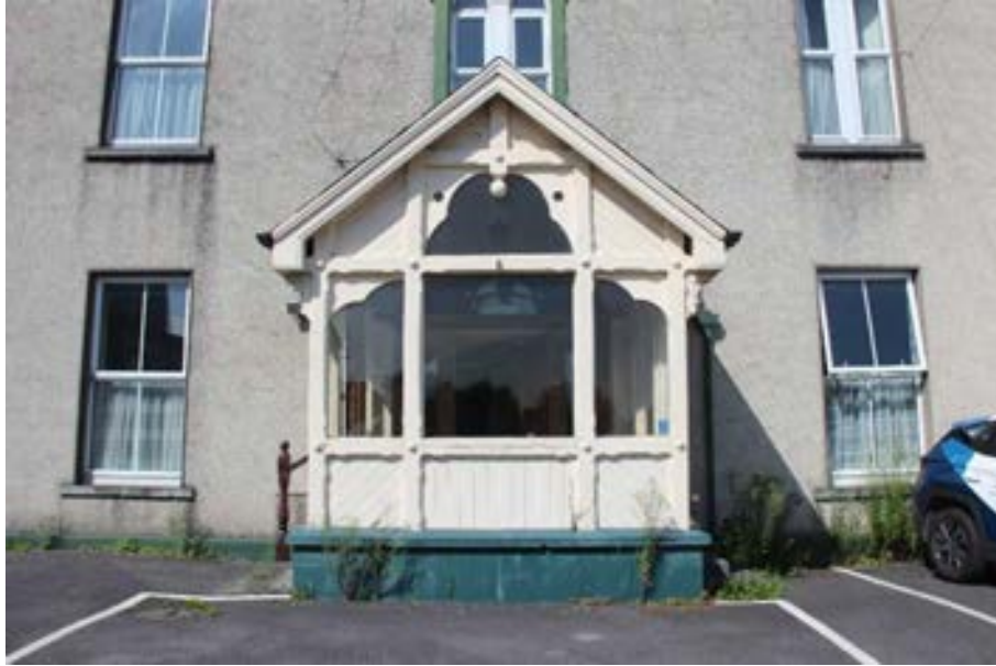
Photograph 7 - Porch with timber frame and panelling over a masonry dwarf wall.
