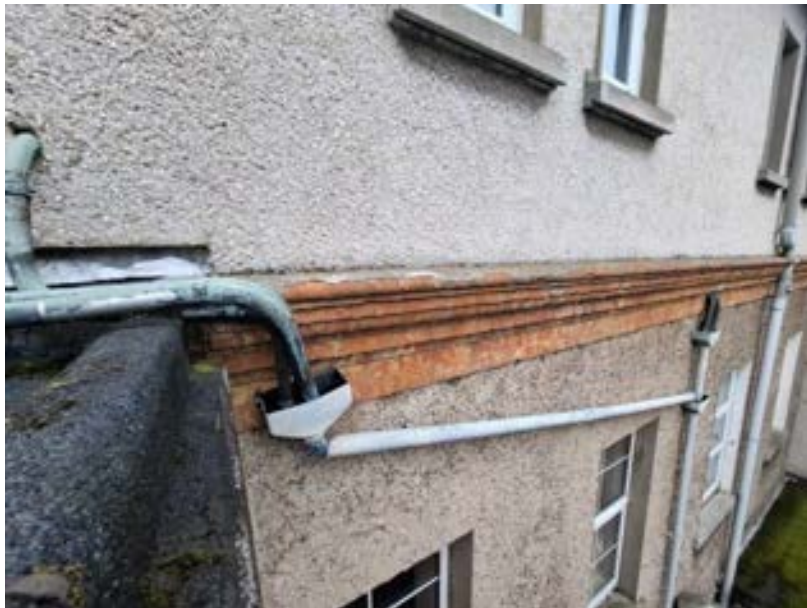
Photograph 6 - Brick cornice and string eaves course preserved along this section of building.
