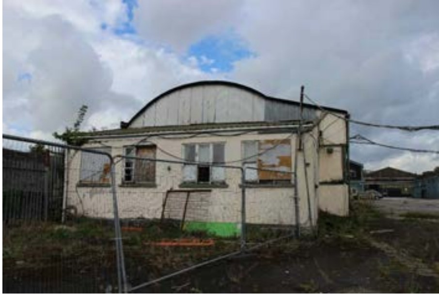
Photograph 3 Lean to building, eastern elevation. With a pressed metal roof covering.
