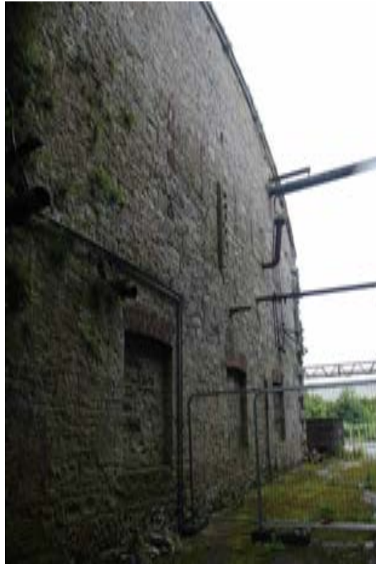
Photograph 5 Northeast elevation of the Engine House, random rubble natural stone construction.
