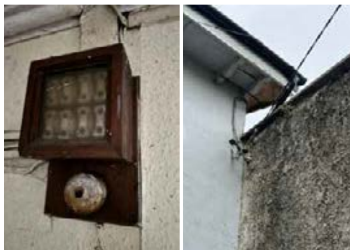
Fig.80 Fuses to left house and junction of right house to gable wall of the mill complex - overhanging closed eaves
