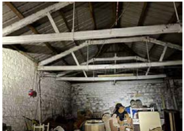
Fig.34 Interior of the Linen Store showing the boundary walls from the inside face and queen post trusses above
