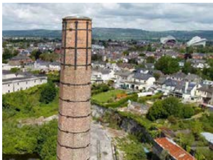
Fig.50 Brick Chimney 1852, with bands and modern capping
