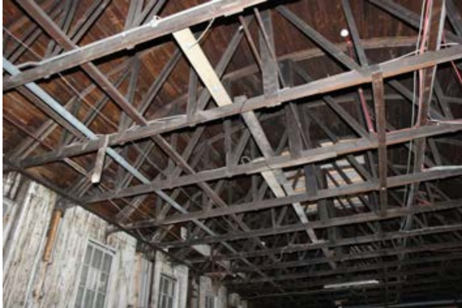
Photograph 8 View of the roof structure, an array of Belfast trusses. Note the underside of the timber sarking boards.
