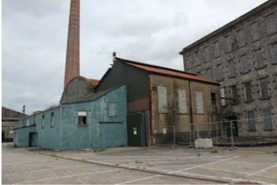
Photograph 3 General view of Building 2, with Corrugated Steel roof covering. Note split pitch of Building 3.
