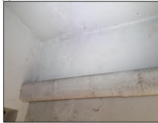
Plate 3-3 Heating pipe wrapped in insulation
