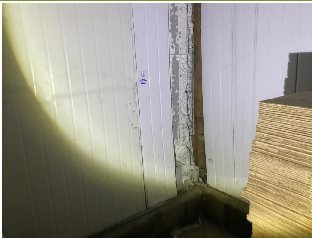
Polystyrene insulation in the wall panels of building 8
