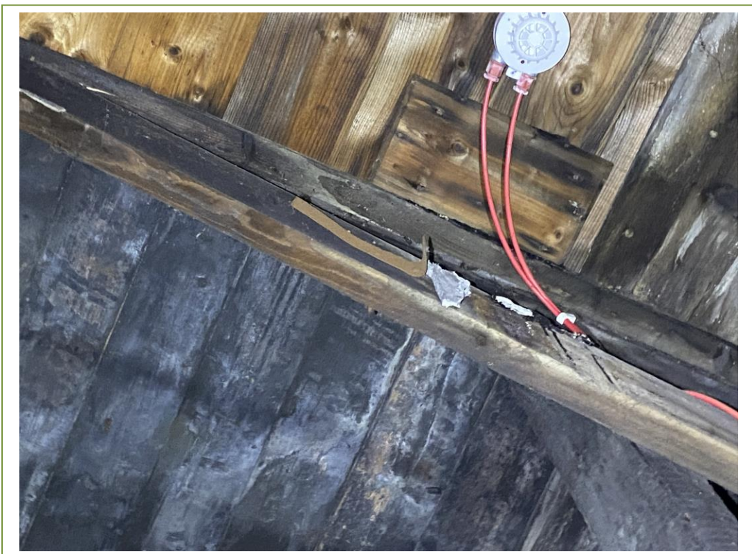
View of the remaining millboard on the higher level of the truss
