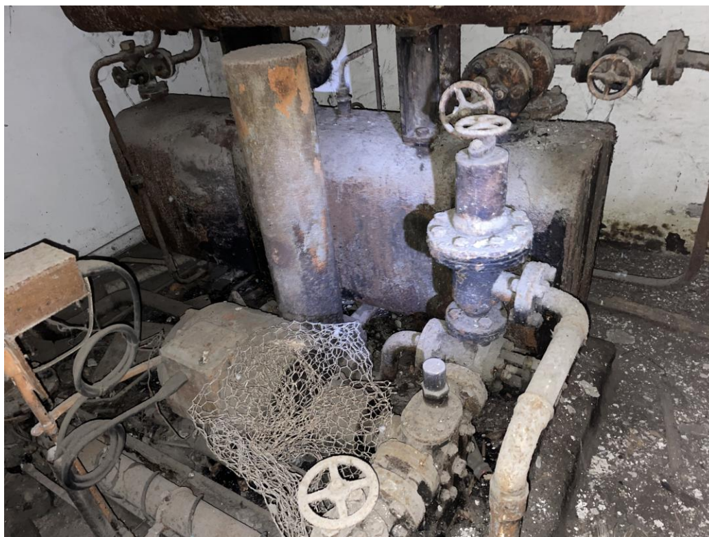
Asbestos containing thermal insulation residue on the boiler unit in the boiler room
