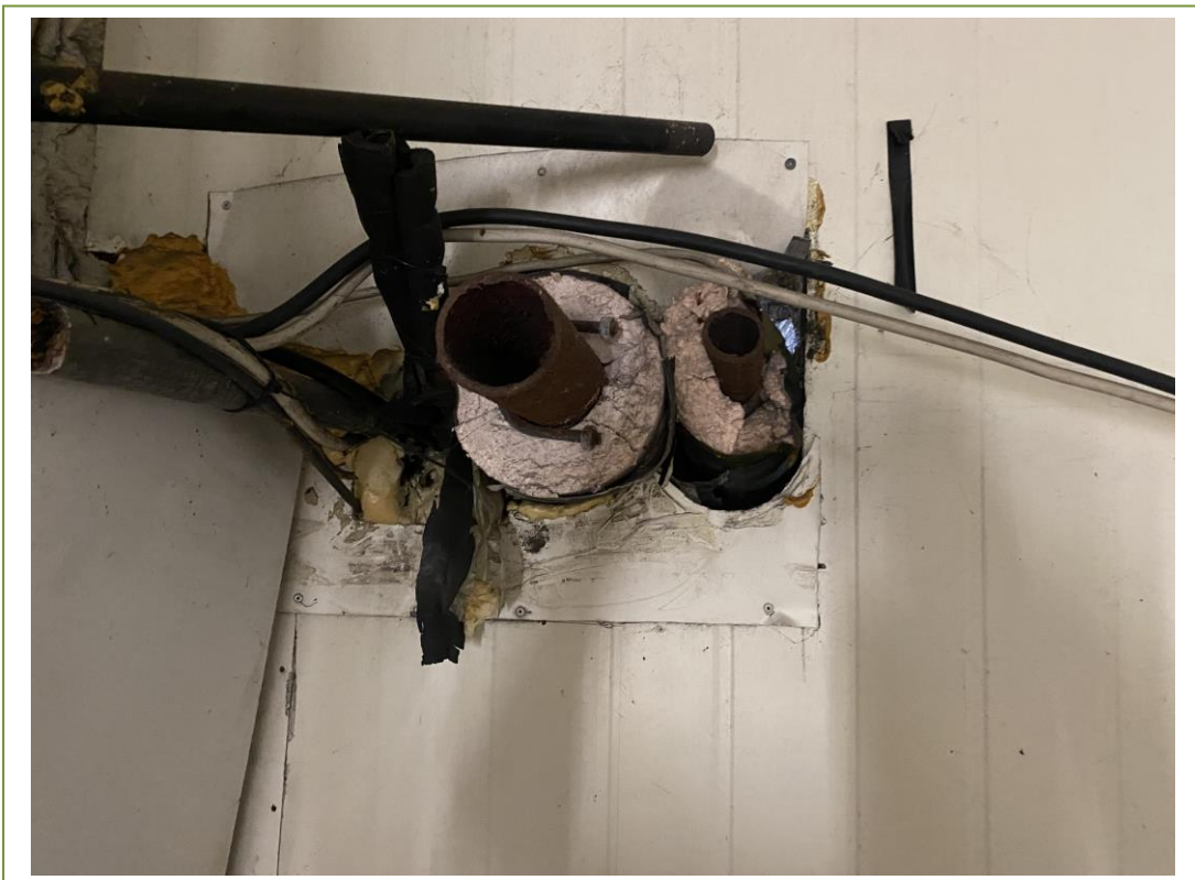
Pipework insulation sampled in building 5
