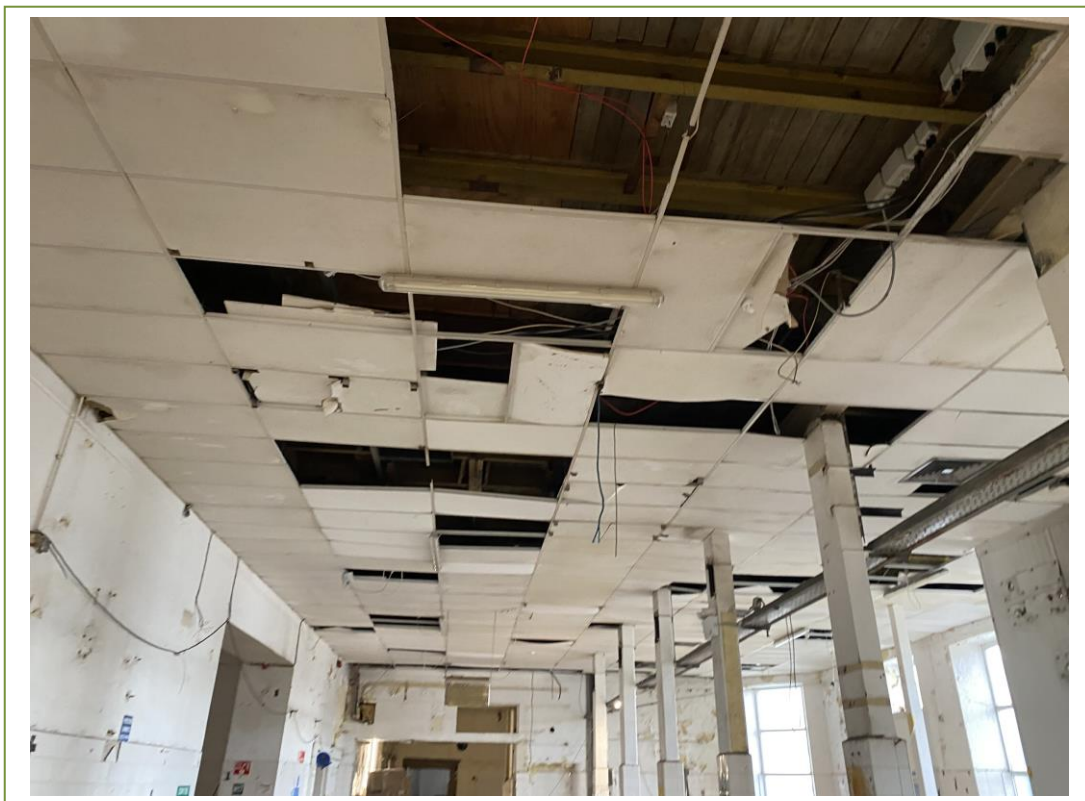
Plasterboard ceiling tiles in building 5
