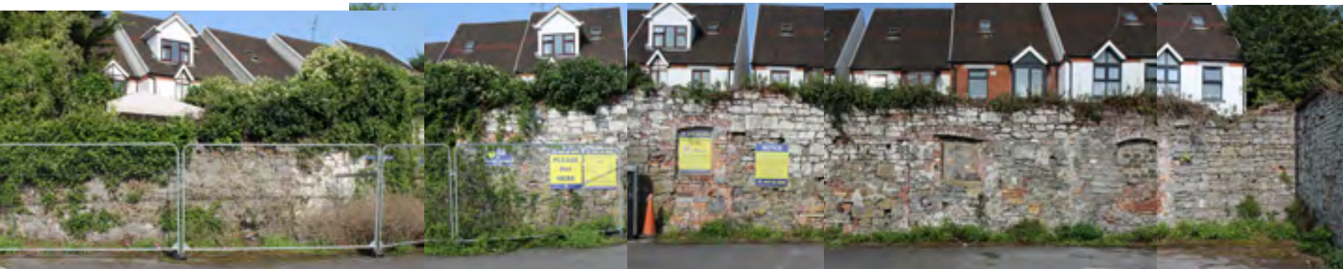
Figure 3.6.1 - Shipyard north walls - currently condition poor requiring repair and rebuilding in parts
