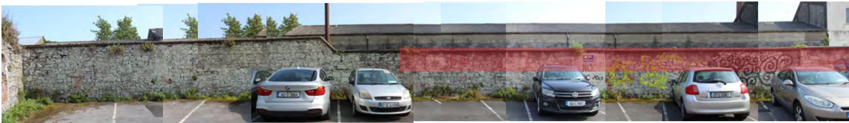
Figure 3.6.2 - Shipyard walls onto North Circular Road - section in red to be lowered in line with raised level of the road.
