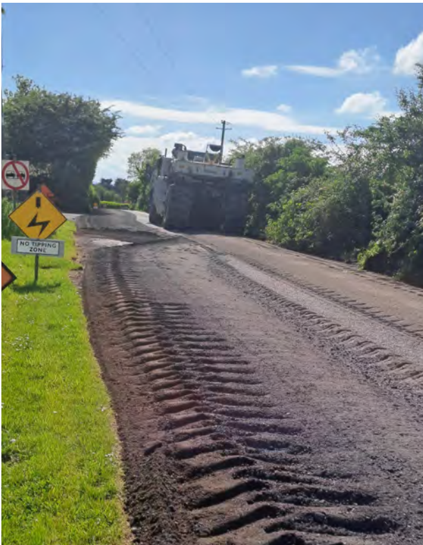
Milling works at Granagh
