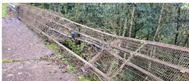
Impact at CB-M08-009.00 Knocknahorgan Bridge
