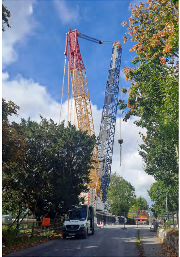
600 tonne Lattice Boom Crawler Crane reinstalling Refurbished Adare Bridge
