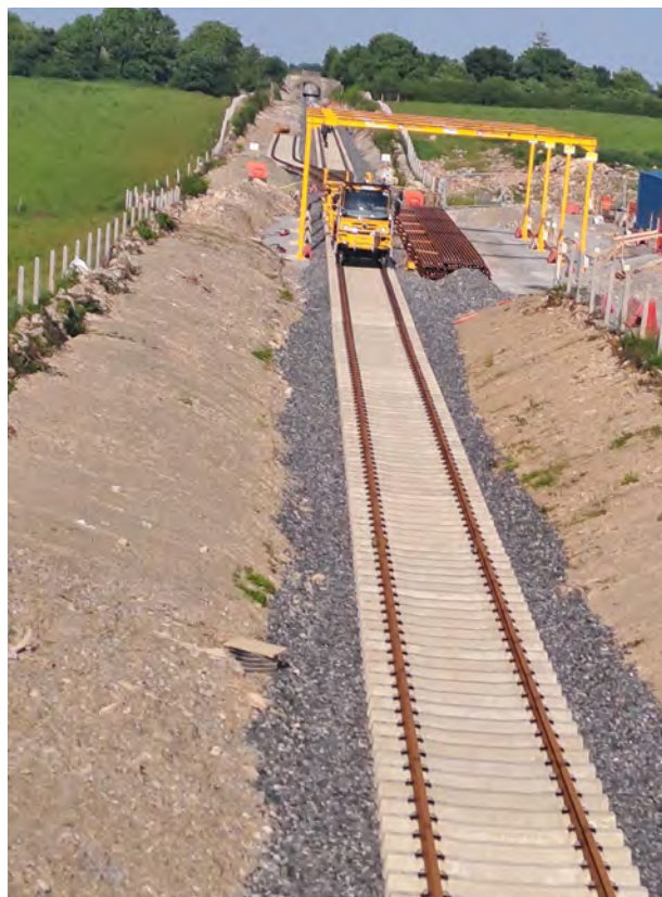
Irish Rail Track Laying at Borigone Askeaton
