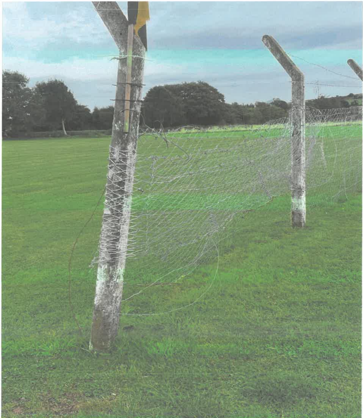
Broken Fence and skewed post
