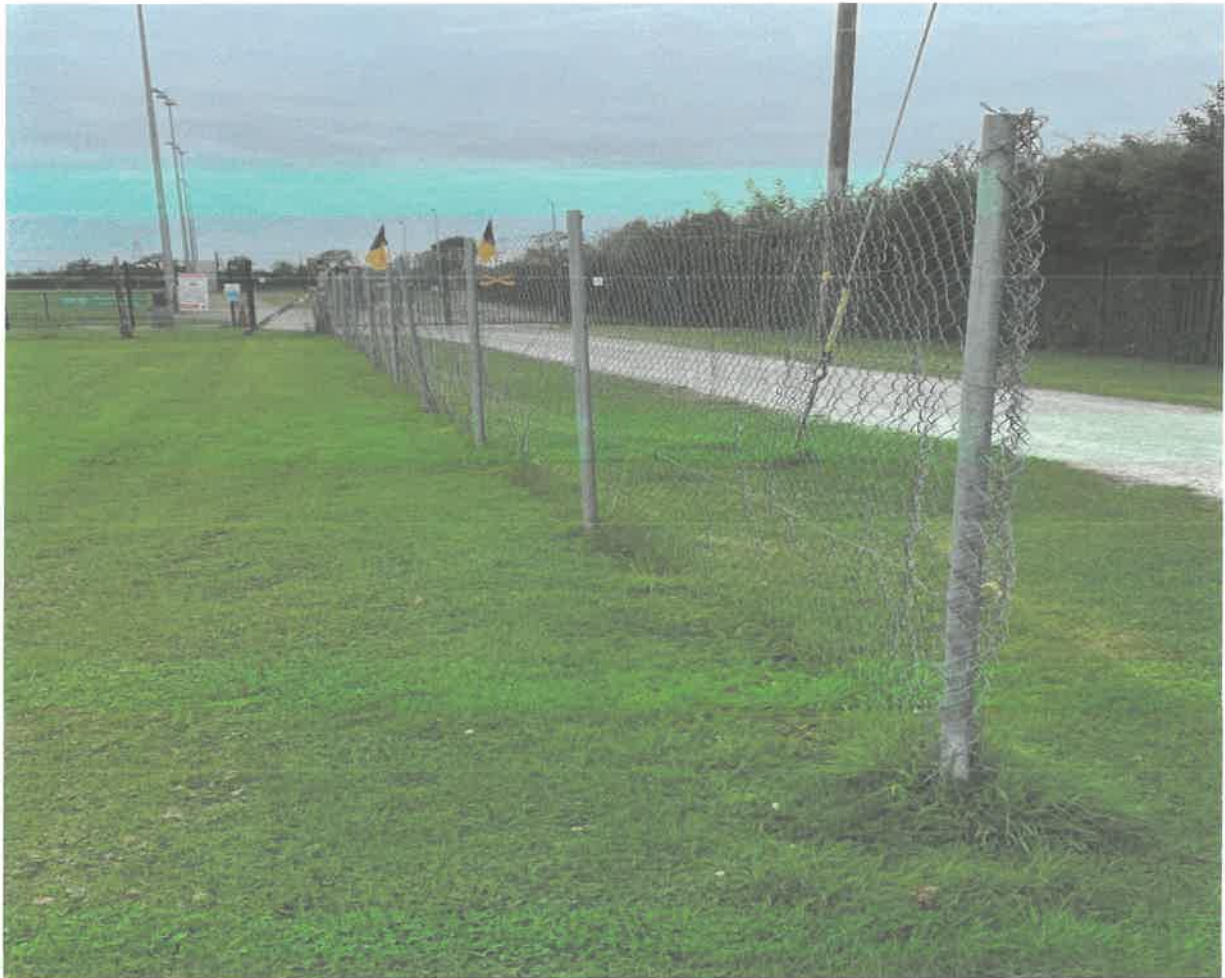
Damaged fence tied back to prevent injury
