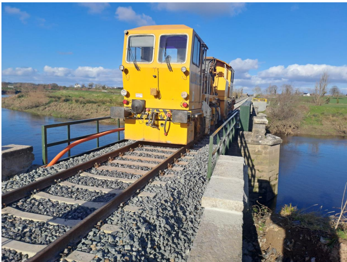
Adare Railway Bridge
