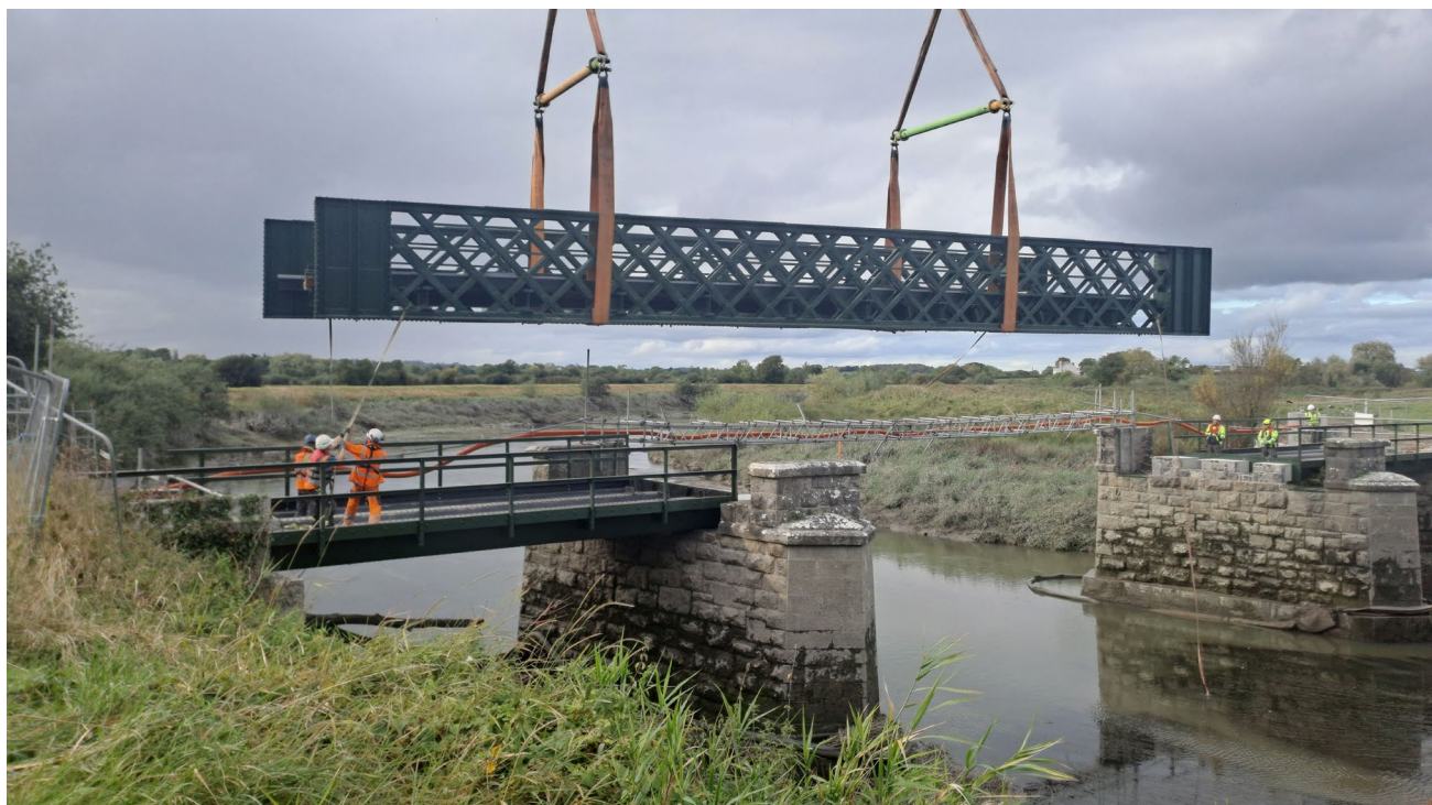
Reinstalling Adare Rail Bridge
