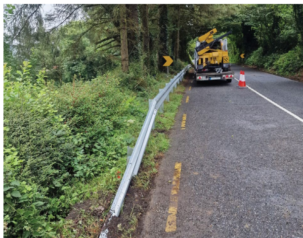
Safety barrier installation on R517
