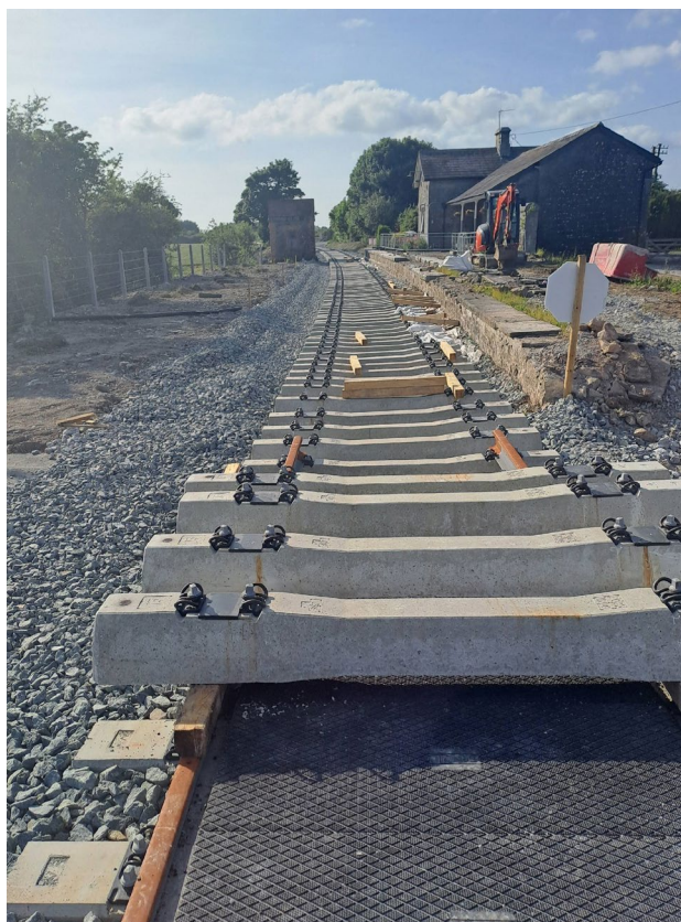
Irish Rail Track Laying at Askeaton Station
