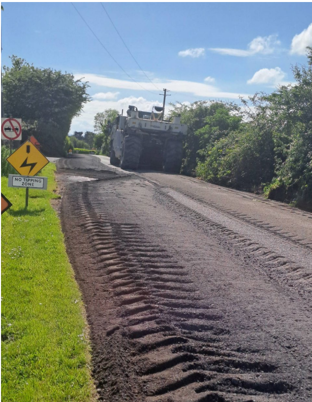
Milling works at Granagh
