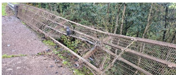
Impact at CB-M08-009.00 Knocknahorgan Bridge
