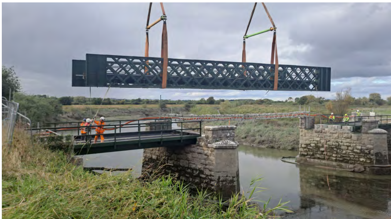
Reinstalling Adare Rail Bridge
