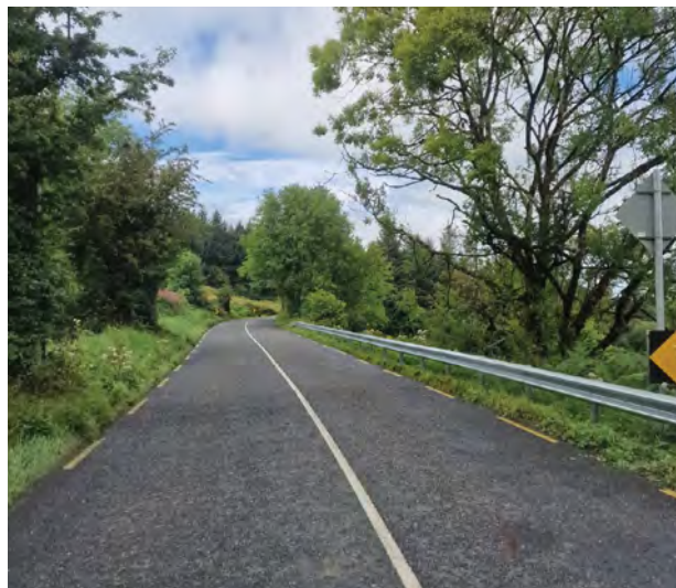
Safety barrier installation on R513
