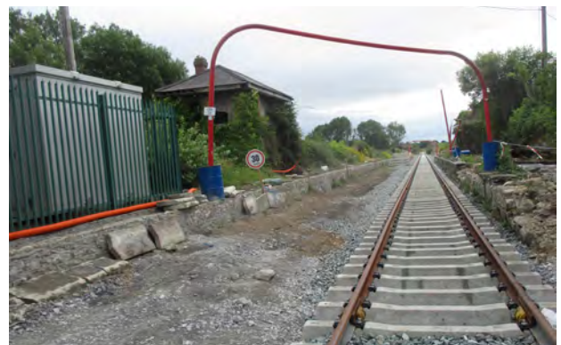
Ongoing railway works
