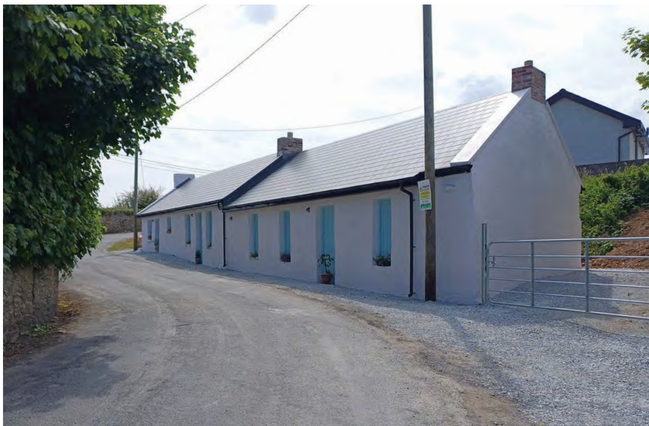
Brewery Lane Askeaton after renovation
