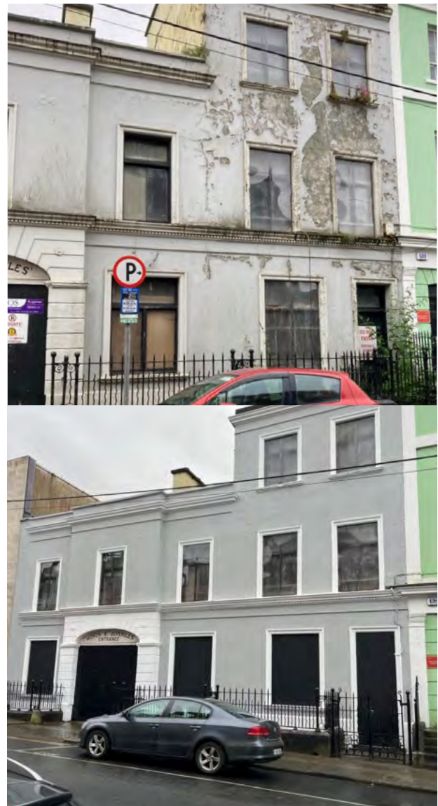
Before and after works
