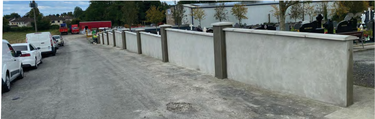
St. Mary's Cemetery, Patrickswell Boundary Wall Repair
