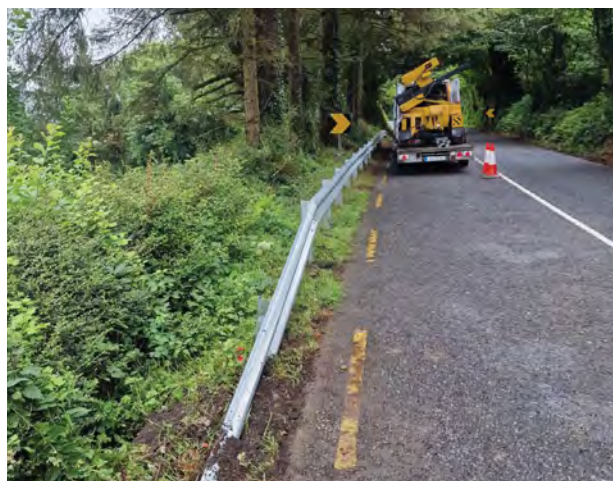
Safety barrier installation on R517
