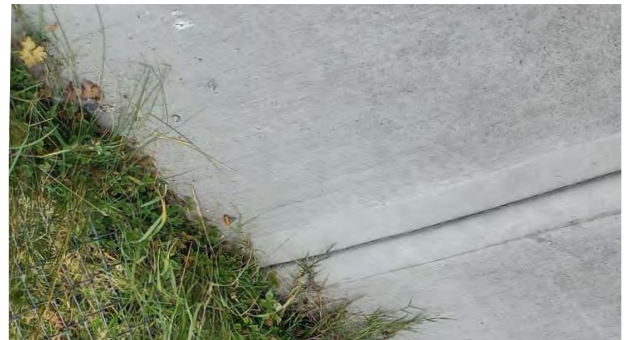
Footpath replacement/extension Athlacca
