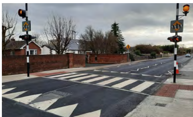
Ballycummin Road Pedestrian Crossing Scheme 2024
