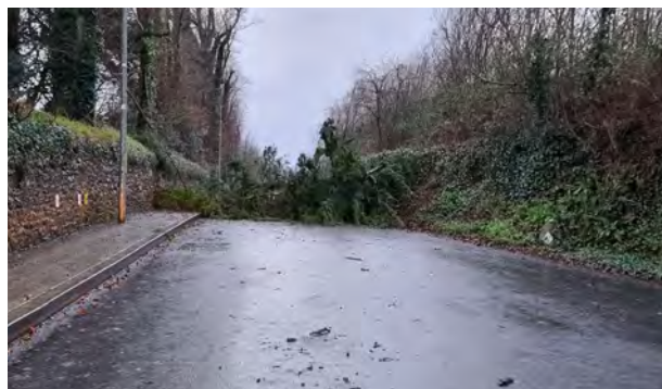
Storm Isha January 2024 – Don Bosco Road Pallaskenry
