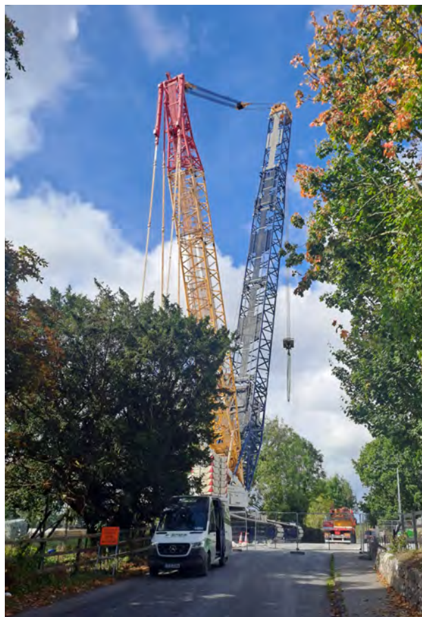
600 tonne Lattice Boom Crawler Crane reinstalling Refurbished Adare Bridge
