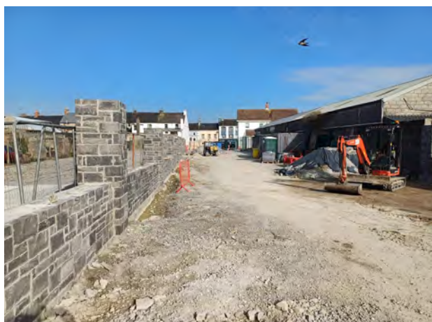
Demolition of O'Riordan's Bar
