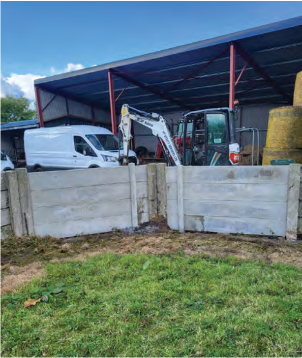
Killonan Graveyard_Boundary Wall Repair
