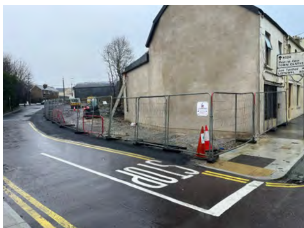
Demolition of property on Colbert Terrace
