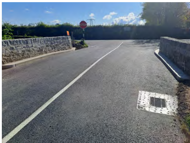
Graigeen Bridge, Cappagh
