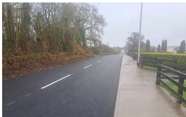
Kyletaun Rathkeale R518 Restoration Improvement Works
