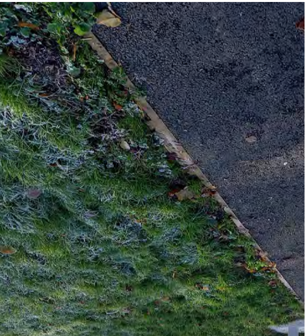
ORIS Riverside Park Redevelopment Kilmallock
