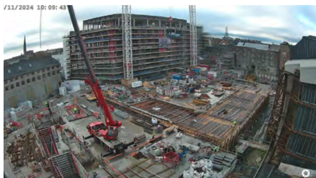
Parcel 1 Concrete Frame Complete (December 2024)
