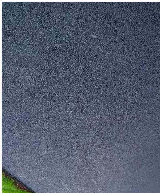
Mount Saint Oliver Cemetery - Footpath Replacement Works
