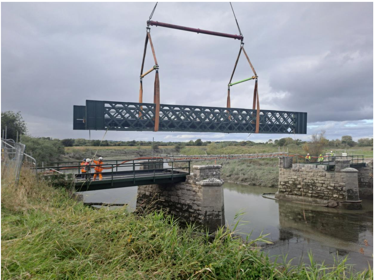
600t Lattice Boom Crane – Adare Rail Bridge Lift
