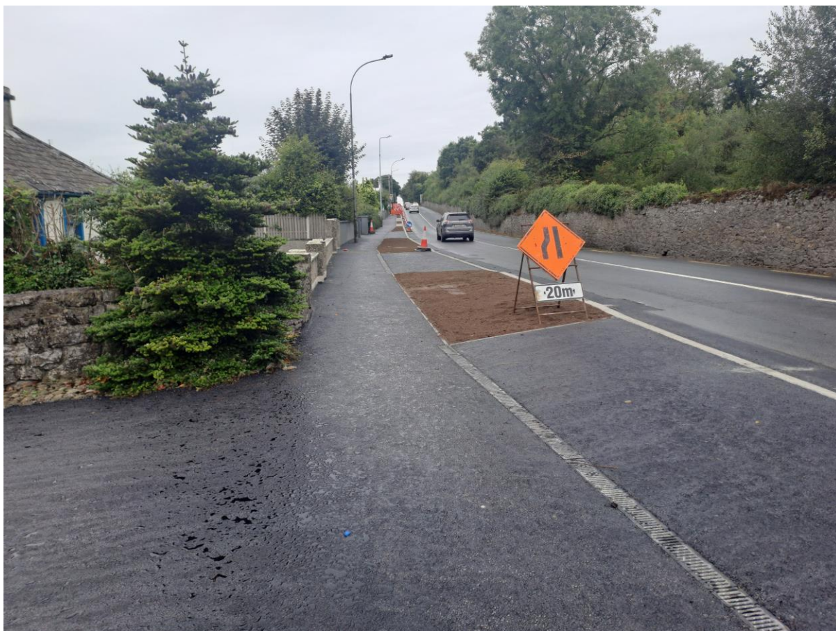
N21 Western Approach Adare- Footpath Works
