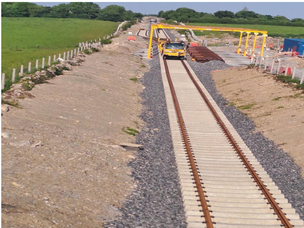
Irish Rail Track Laying Borrigone
