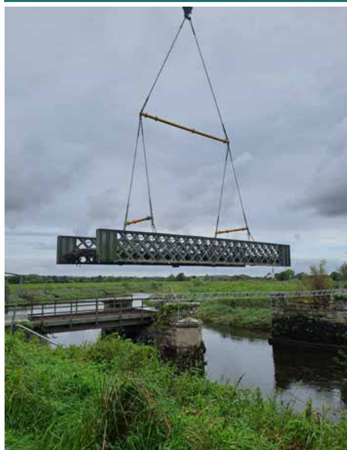
700tonne Crane Lift
