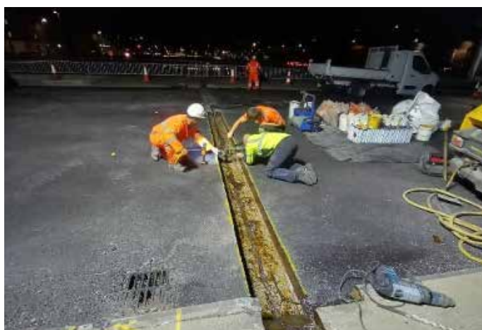
Installation of the type 6 joint
