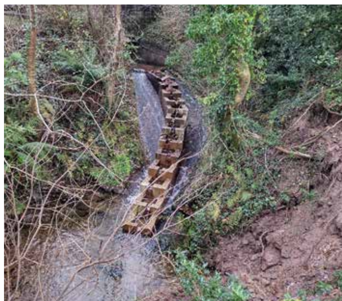
Completed fish pass work at Glenbeigh.
