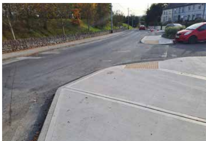
Junction tightening St. Senan's Terrace Croom
