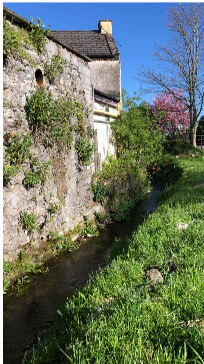
Figure 5.5: Barnakyle River in the Village Centre
