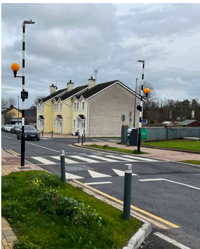
Fig. 7.2 Pedestrian Crossing on Main Street constructed as part of Patrickswell Phase 2 Village Renewal Scheme
