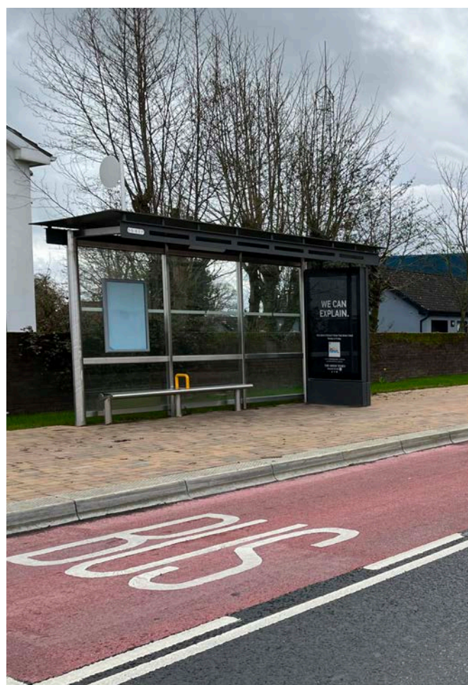
Figure 7.1: Bus Stop Facilities Constructed as part of Phase 2 Of A Village Renewal Scheme on Main Street
