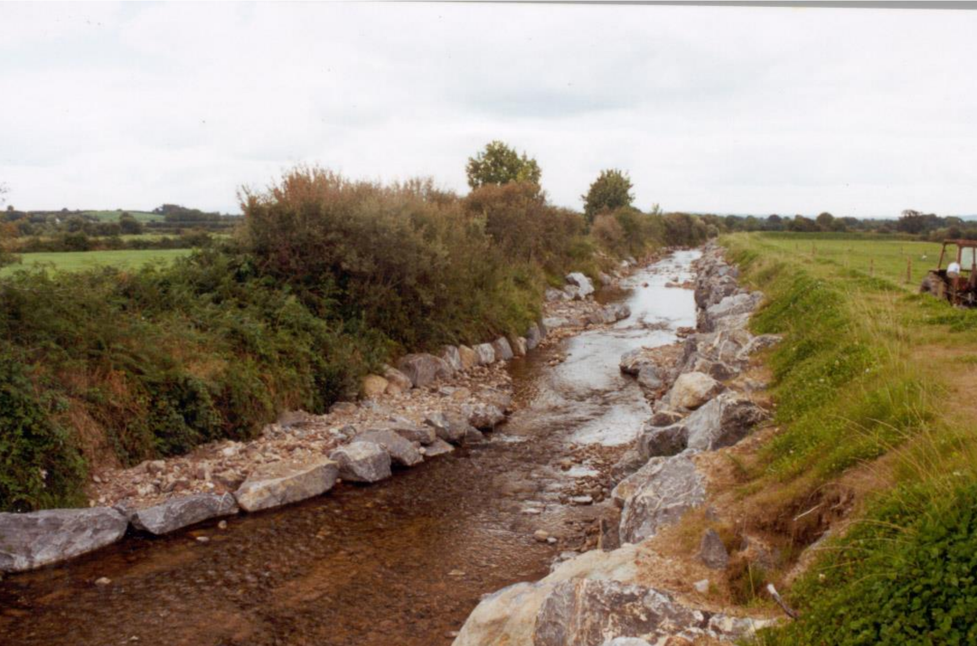
Instream River Restoration – Alternating deflectors
