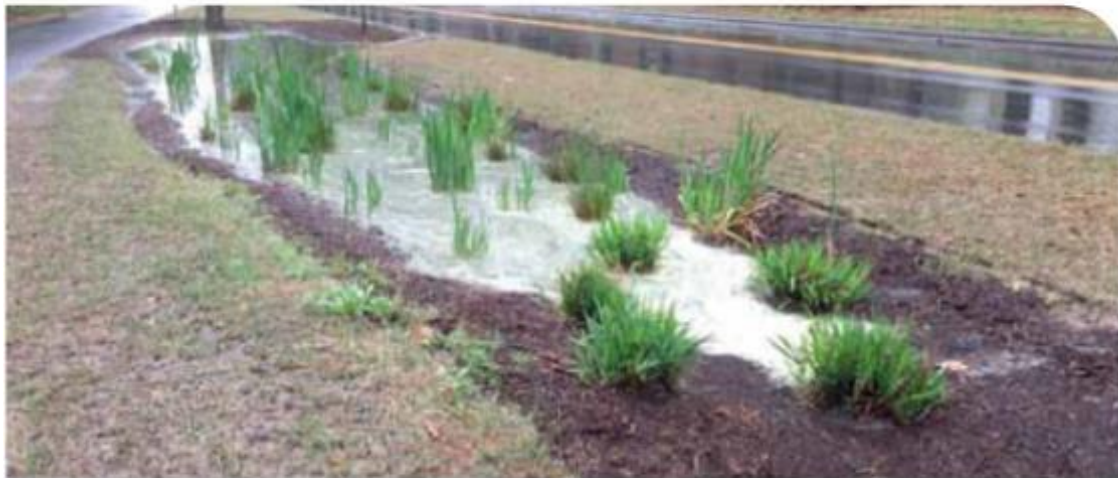
Example of Rain Gardens treating surface water runoff from a road
