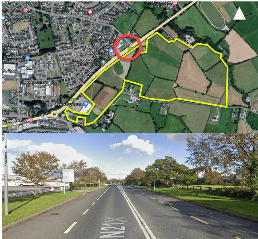
Figure 4.10 Zone 1: Appropriate junction access with the N21 carriageway.
