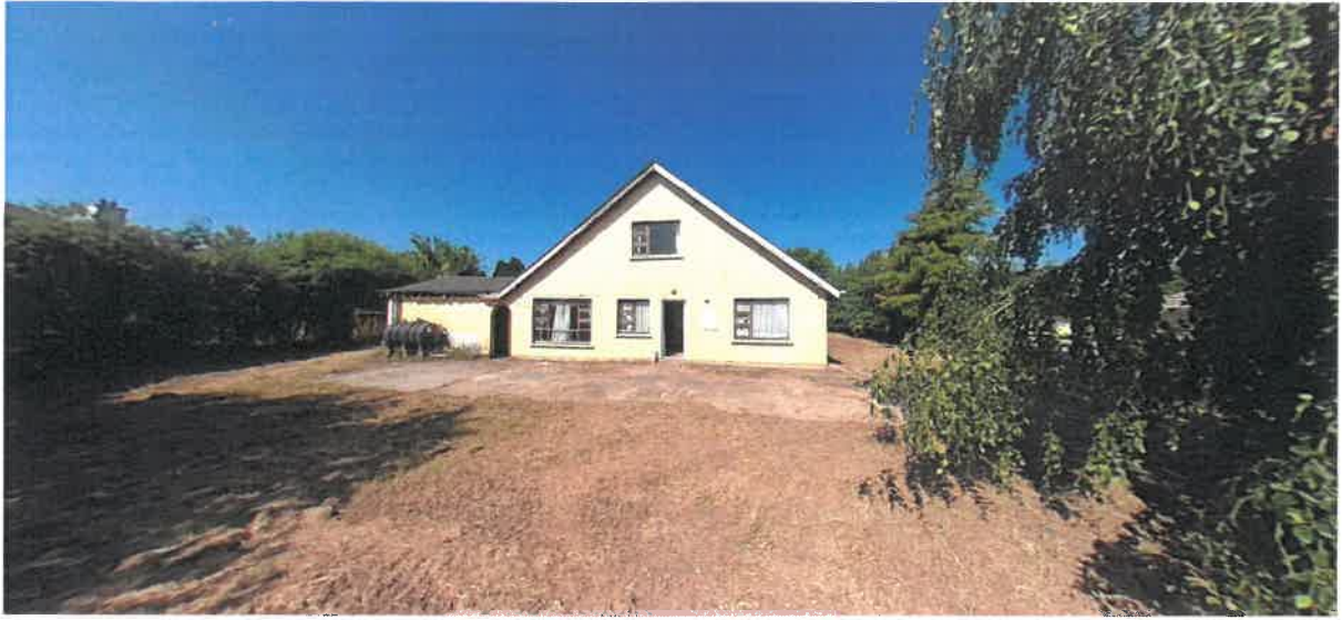
Rear of Property following Site Clearance
