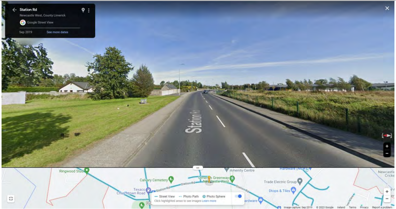
Figure 10.3 Station Road (c: Google)
