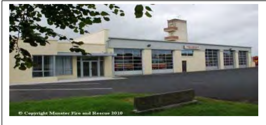
Figure 9.3 Newcastle West Fire Station
