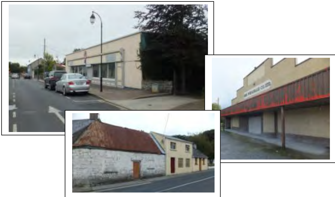
Figure 10.1 Examples of vacant buildings on Lower Maiden Street, Sheehans Road and Knockane
