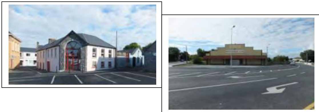
Figure 3.2 Large scale vacant prominent buildings in Newcastle West
