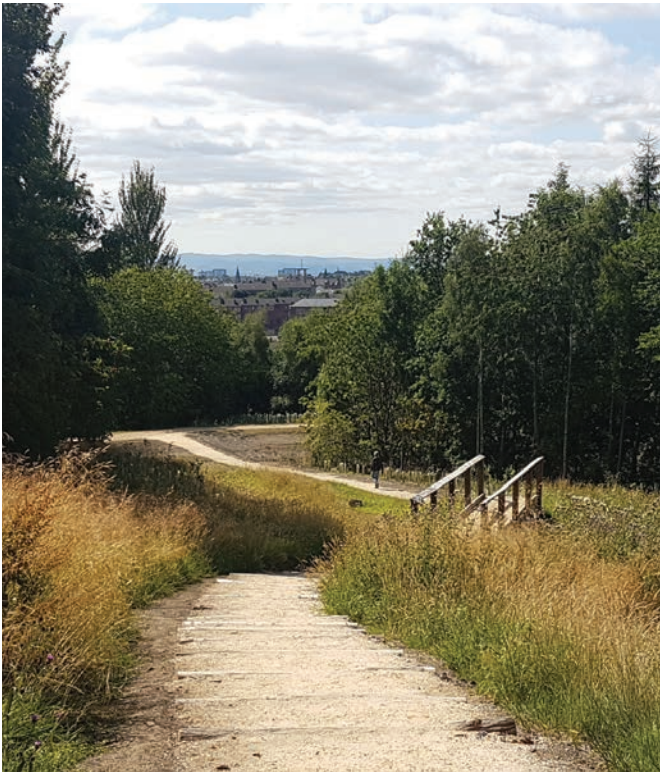
▲ Installation of multi-user routes
