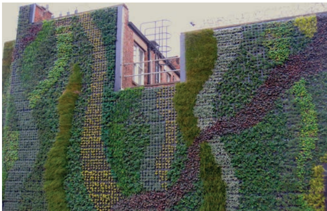
▲ Green walls as a mechanism to improve air quality, enhance biodiversity and regulate urban temperatures
