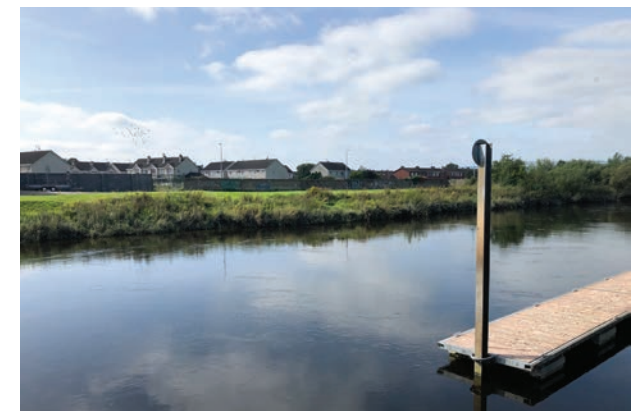
▲ Existing slipway on the River Abbey, adjacent Athlunkard Boat Club
