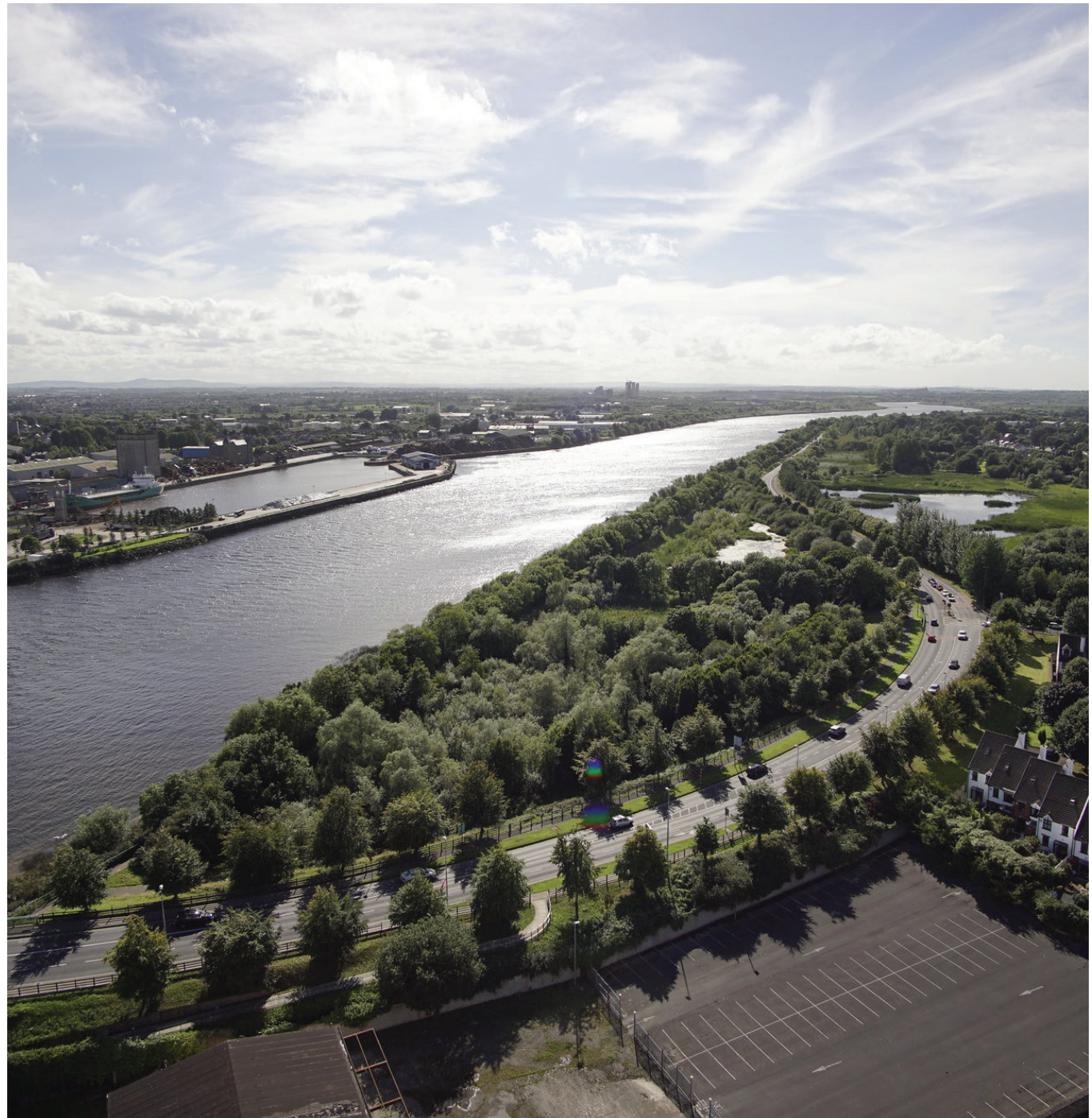
▲ View looking west following the alignment of the R527 parallel to the River Shannon
