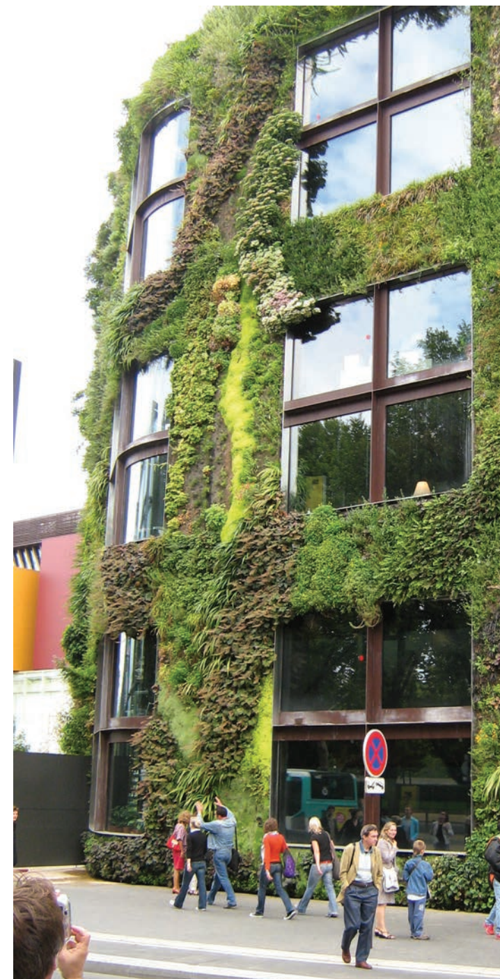
▲ Vertical greening / green walls
