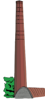
Red brick chimney stack
