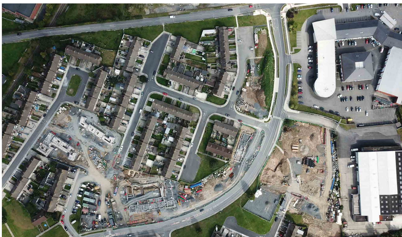
Dalgaish Park/Cosgrave Park under construction
