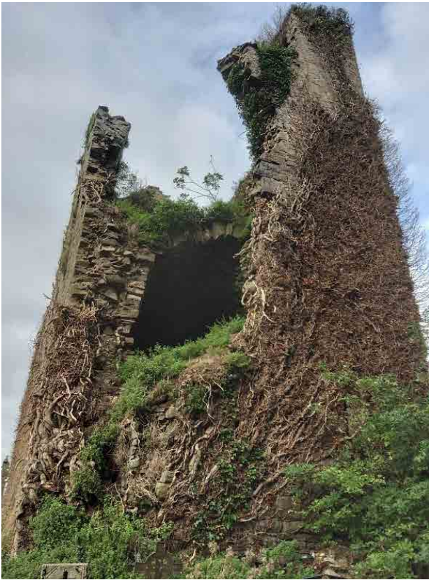
Works at Ballynoe, Bruree Before
