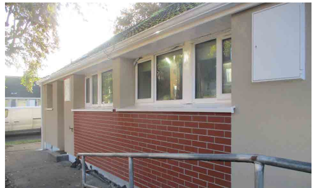
Energy Retrofit 2022 – Schoolhouse Lane, Limerick
