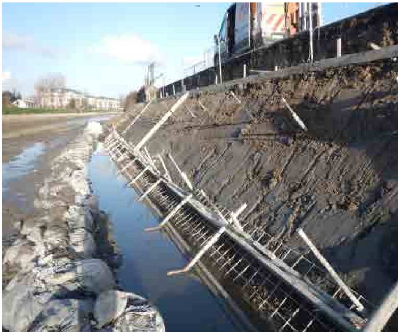
Blennerville Canal Walls - Ground anchors installed, awaiting grouting and masonry finish
