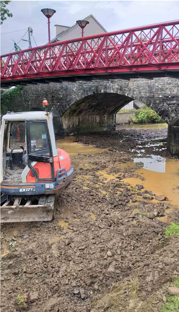
Athea Flood Relief Scheme - Advanced Works
