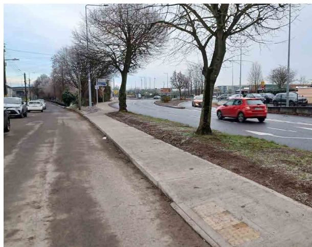
New Footpath Link at Ballykeeffe Roundabout
