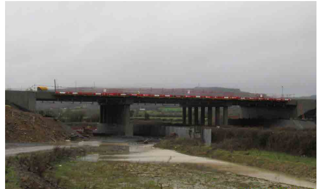
Ballygrennan Bridge under construction
