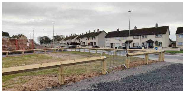
Galvone Arms site Southill post-demolition
