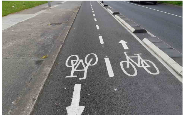
Childers Road looking towards Kilmallock Roundabout
