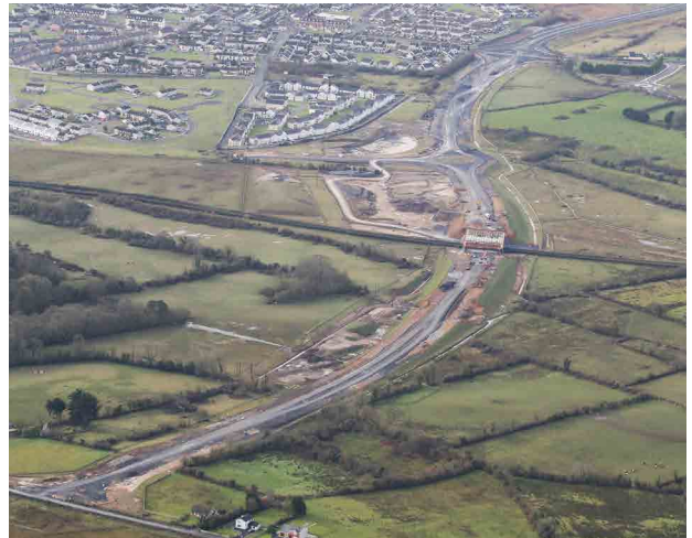
Aerial View of the Coonagh Knockalisheen Distributor Road March 2022
