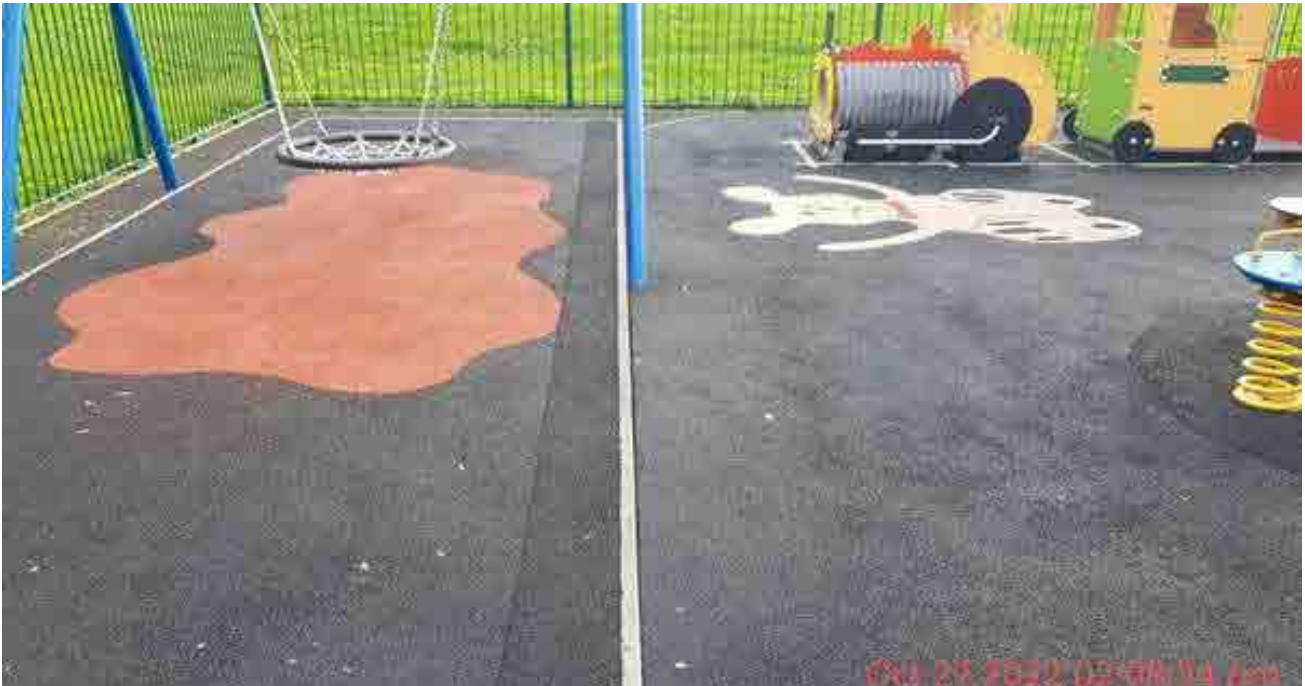
Rathkeale Community Playground: Surface Wetpour edging repairs under Repair and Upgrade Scheme of Assistance for Community Playgrounds
