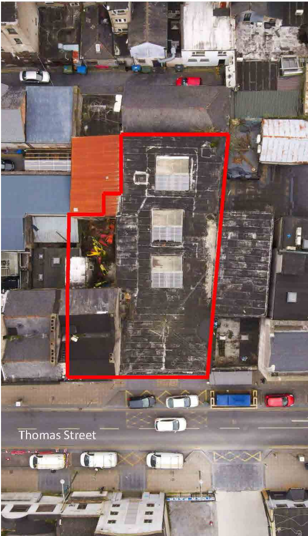
Aerial View of 33 and 34 Thomas Street
