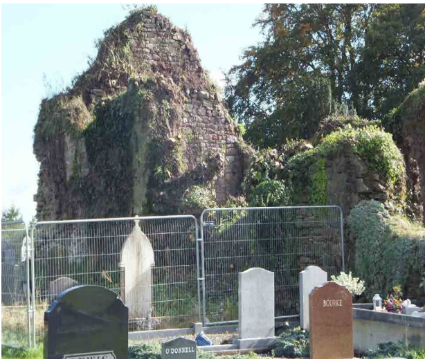
Works at Galbally Church
