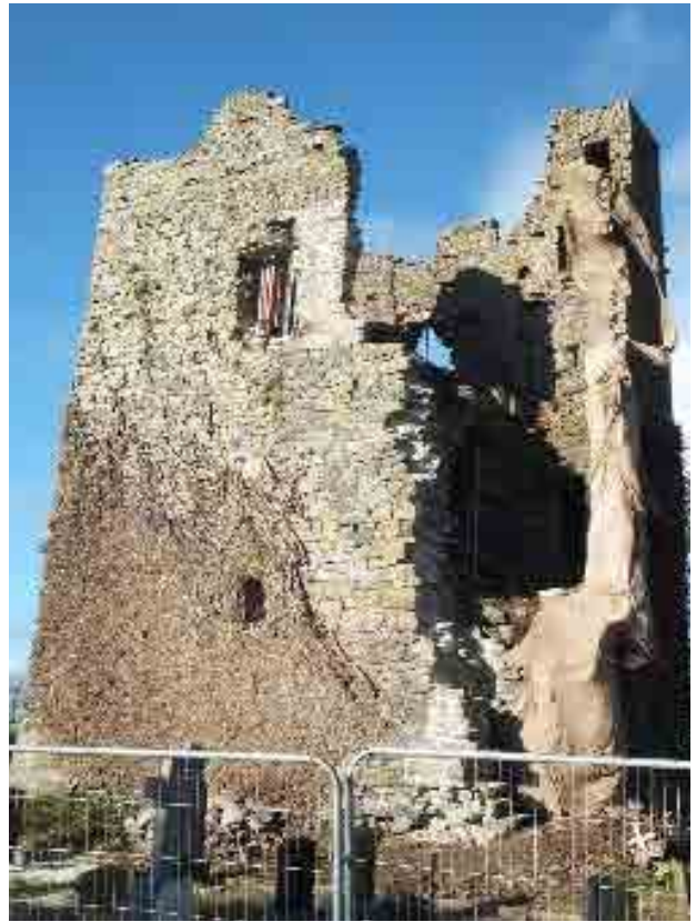
Works at Ballynoe, Bruree After
