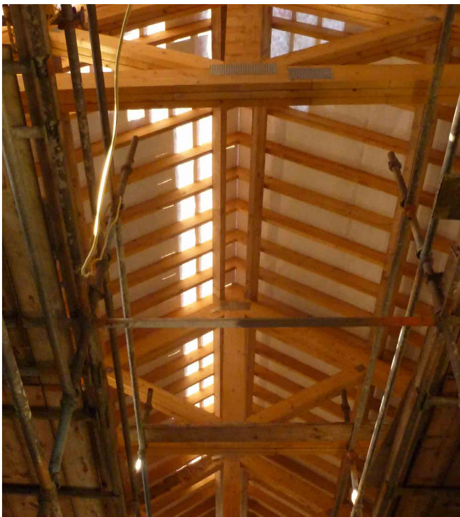
Interior View of the Roof Structure of the Canal Harbour Building
