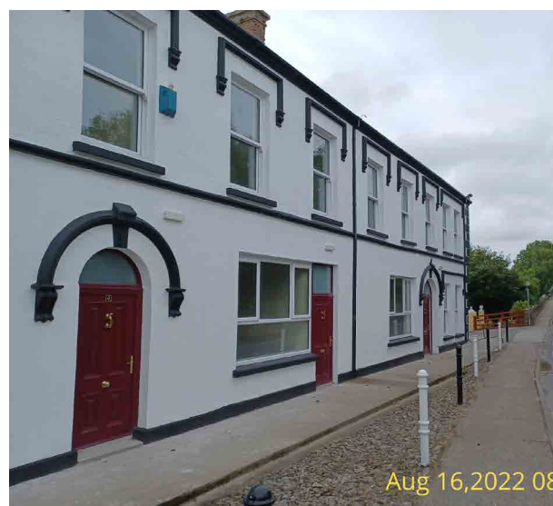
Pallasgreen Property after refurb by owner
